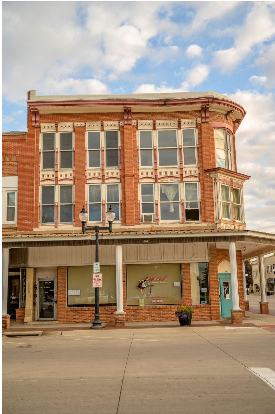
Photograph 44-00366-002. South elevation, looking north (October 2023)
