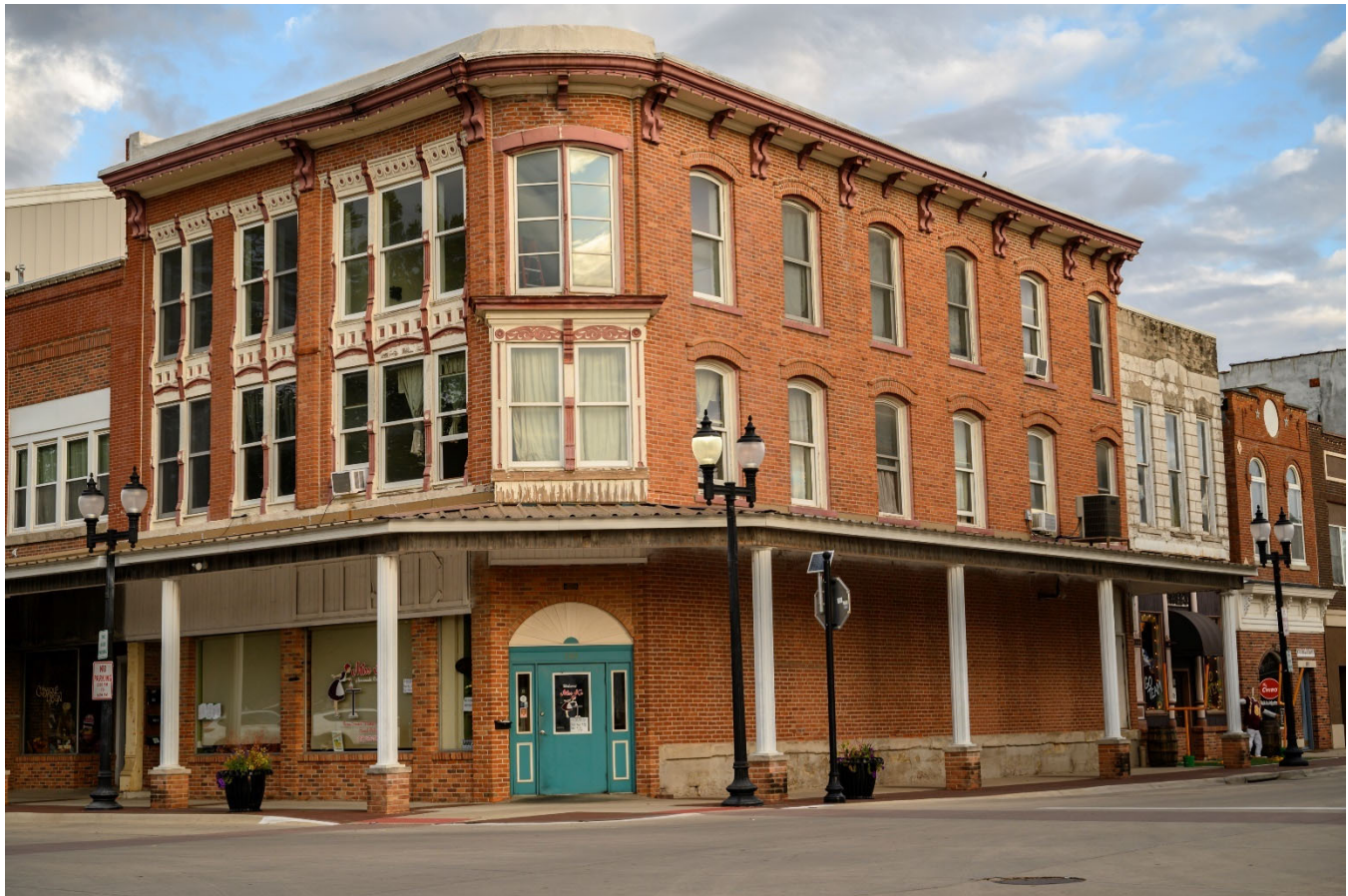
Photograph 44-00366-001. South and west elevations, looking northwest (October 2023)
