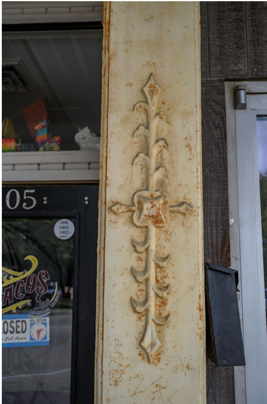
Photograph 44-00367-002. Cast iron column detail on south elevation, looking north (October 2023)
