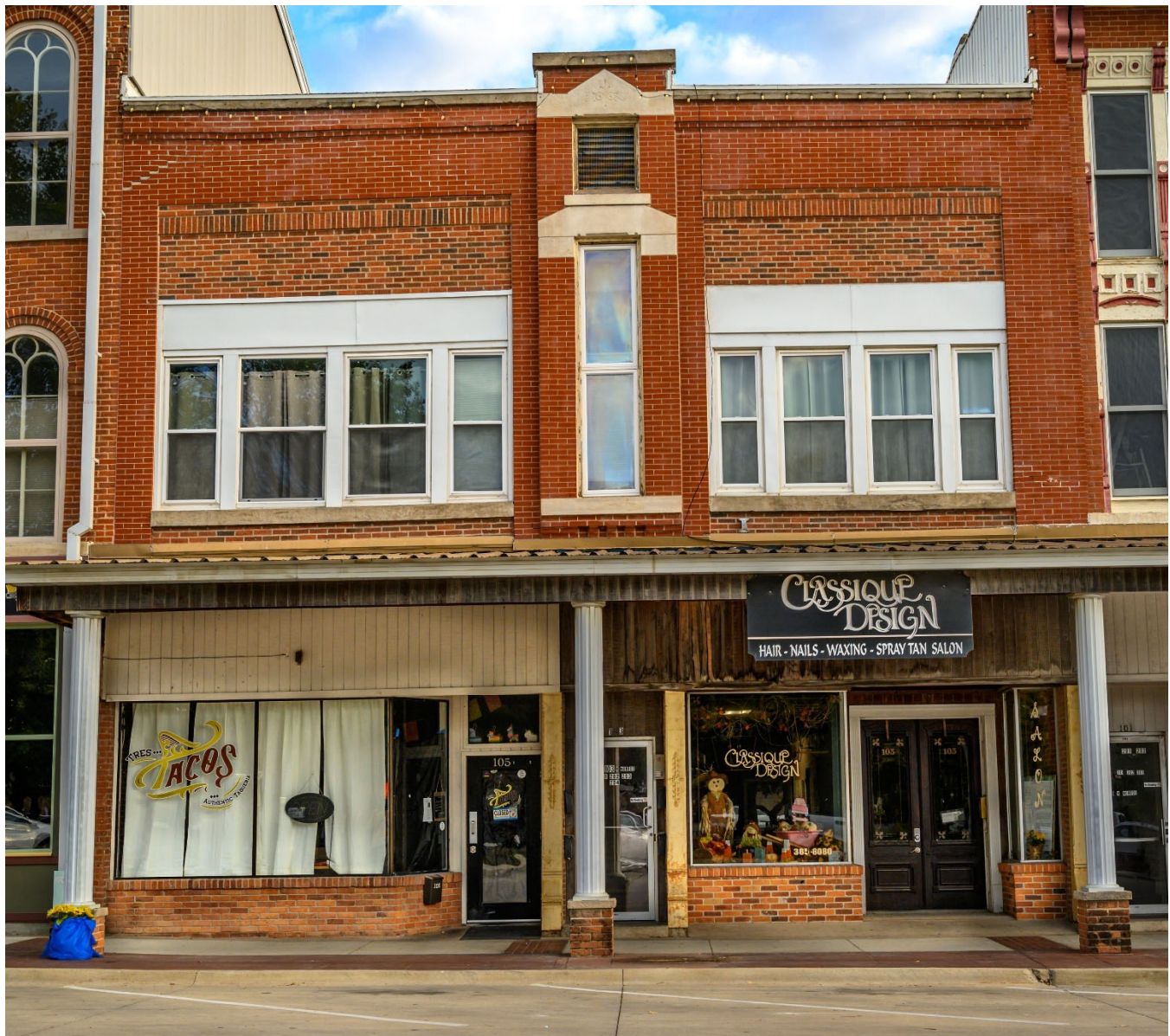
Photograph 44-00367-001. South elevation, looking north (October 2023)
