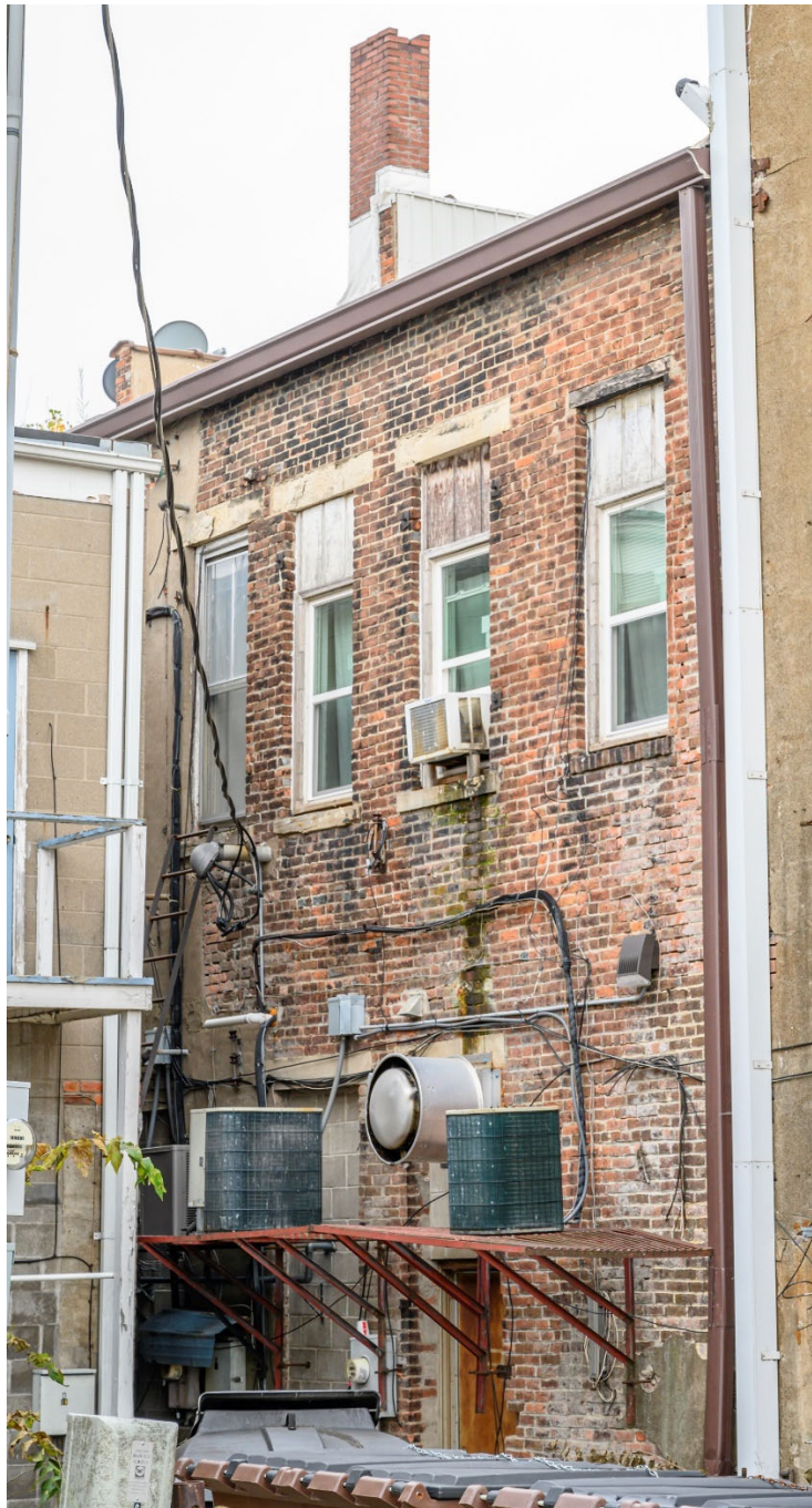
Photograph 44-00367-003. North elevation, looking southeast (October 2023)
