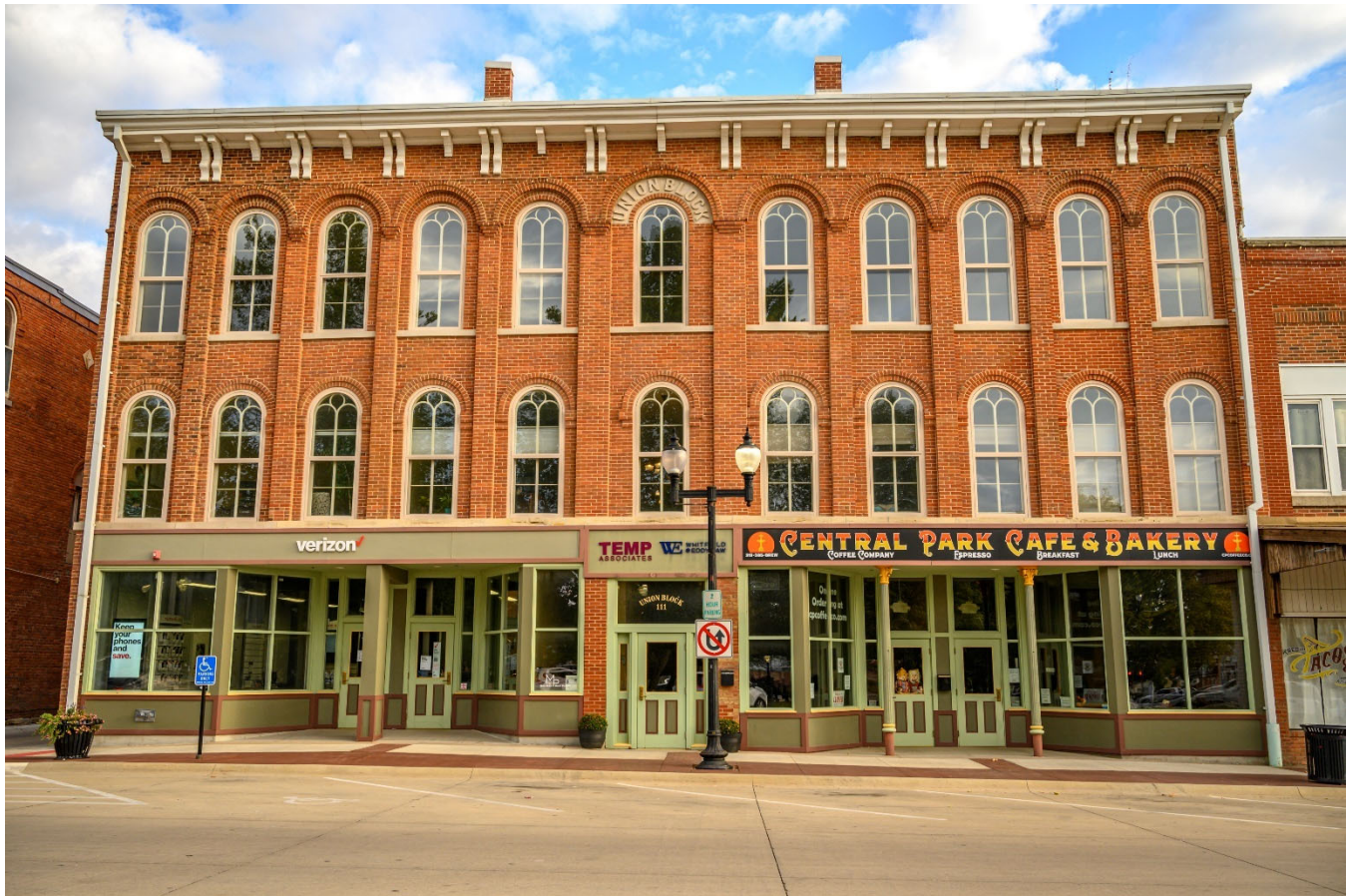
Photograph 44-00368-001. South elevation, looking north (October 2023)
