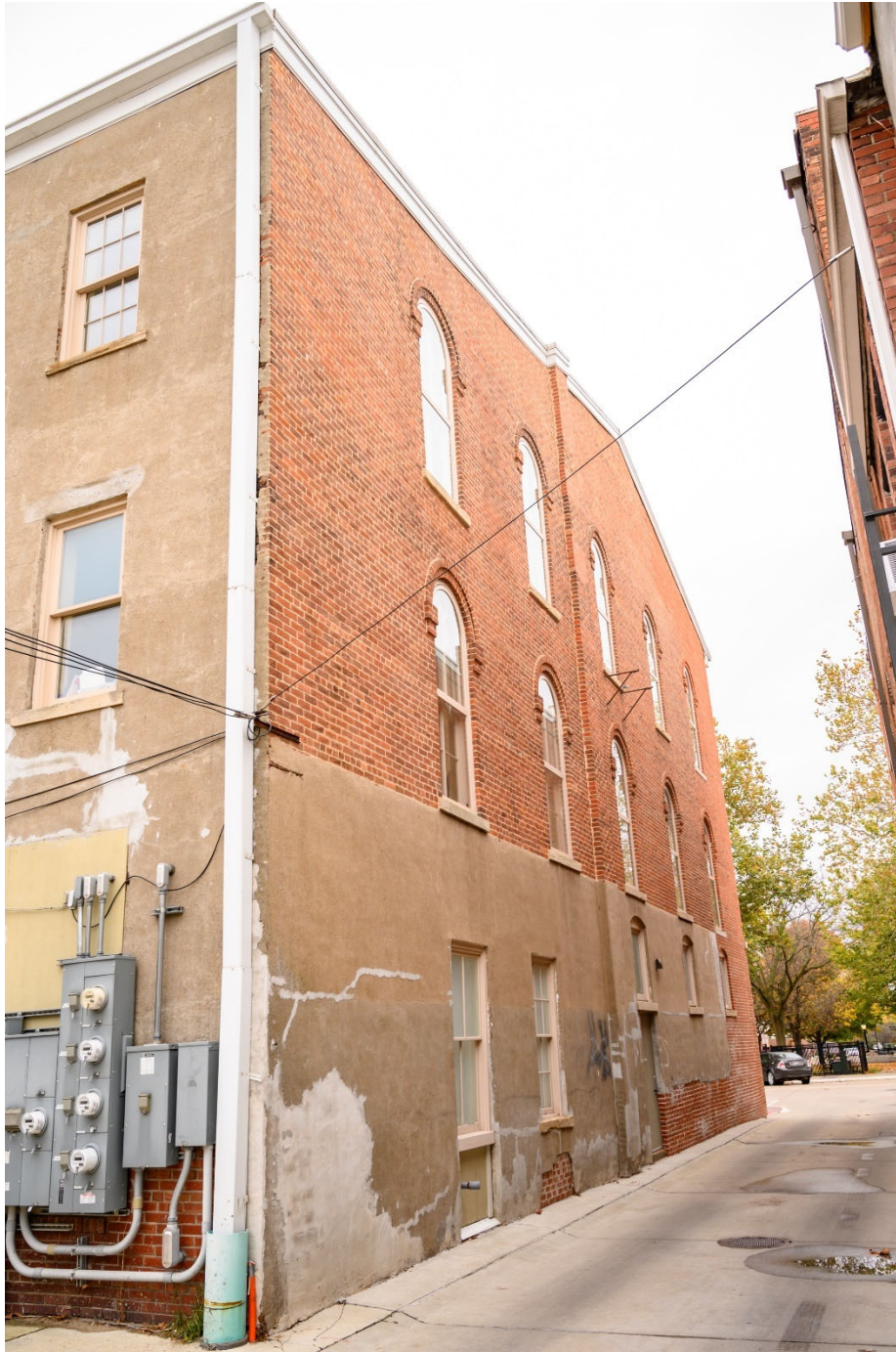
Photograph 44-00368-003. West elevation, looking southeast (October 2023)
