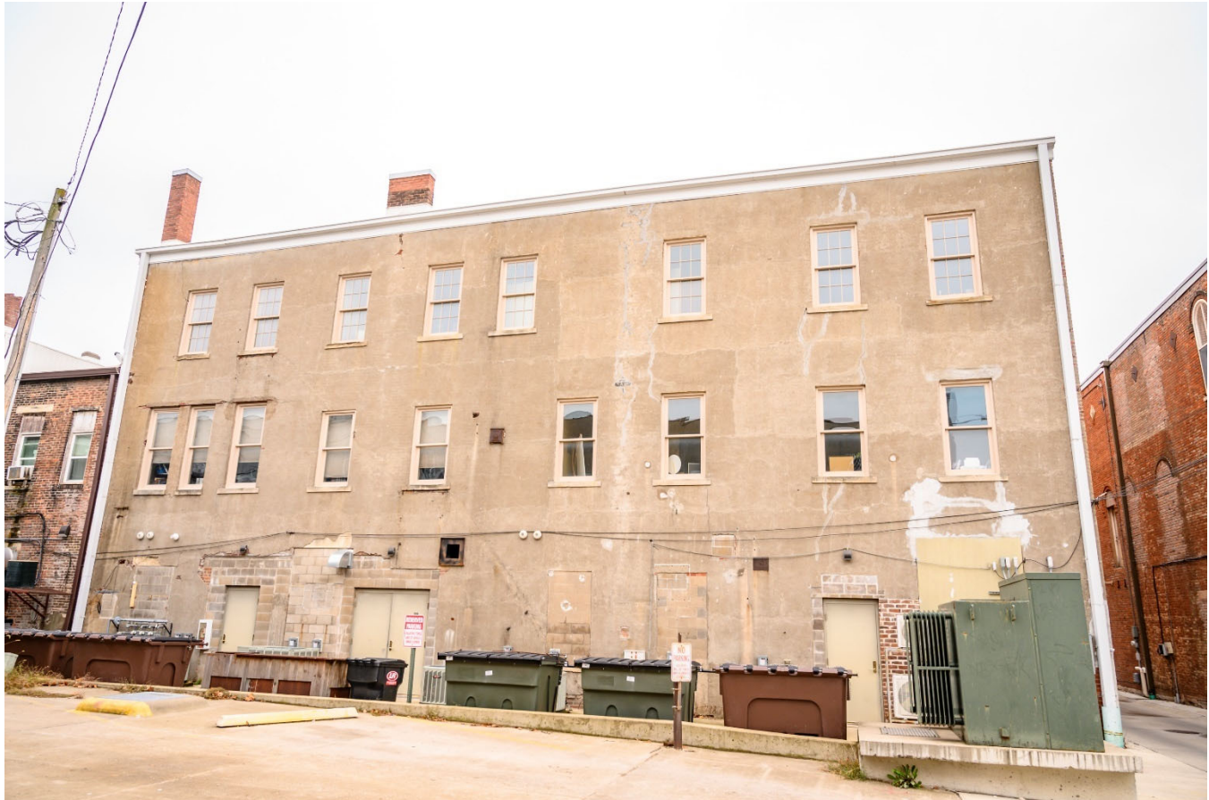
Photograph 44-00368-004. North elevation, looking south (October 2023)
