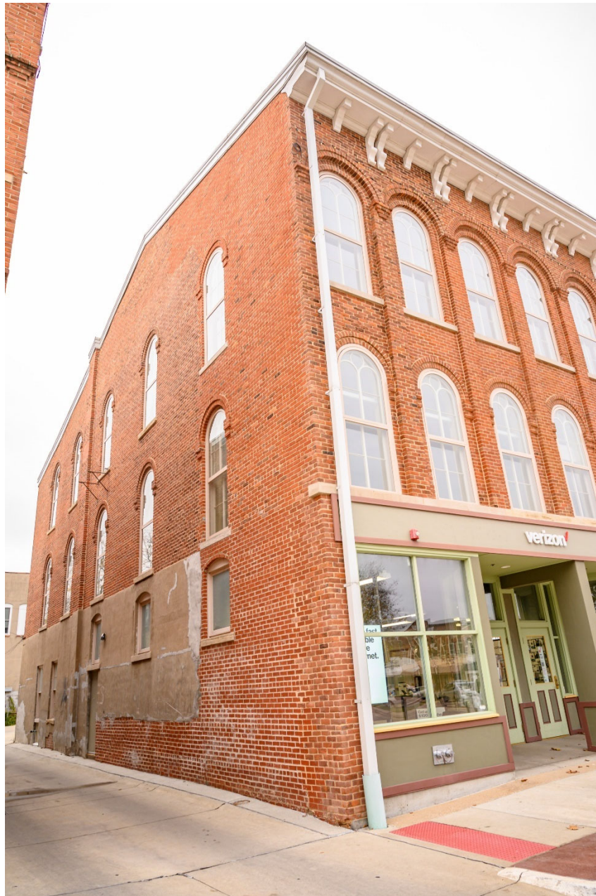
Photograph 44-00368-002. West elevation, looking northeast (October 2023)
