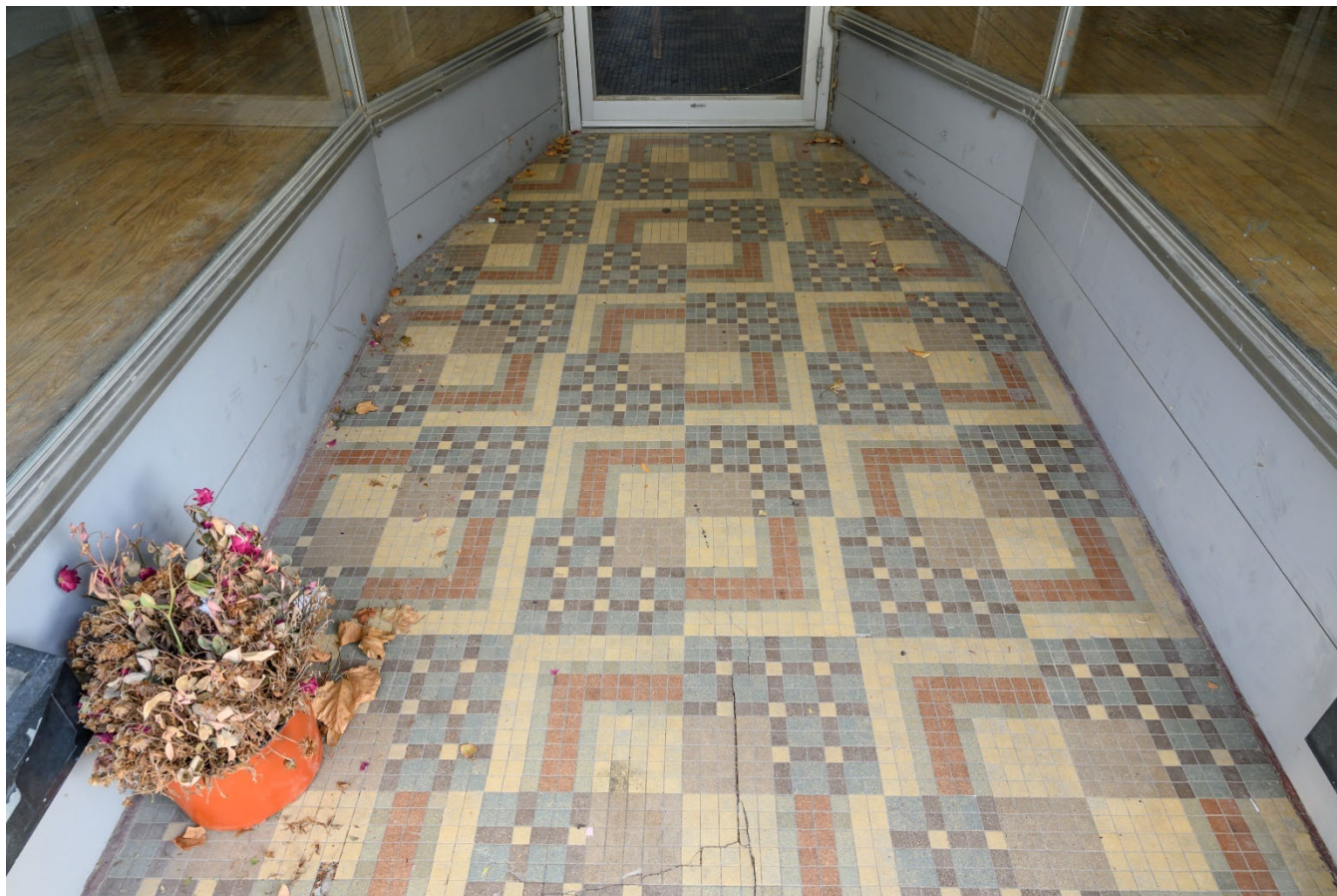
Photograph 44-00370-002. Tile entry in storefront, looking north (October 2023)
