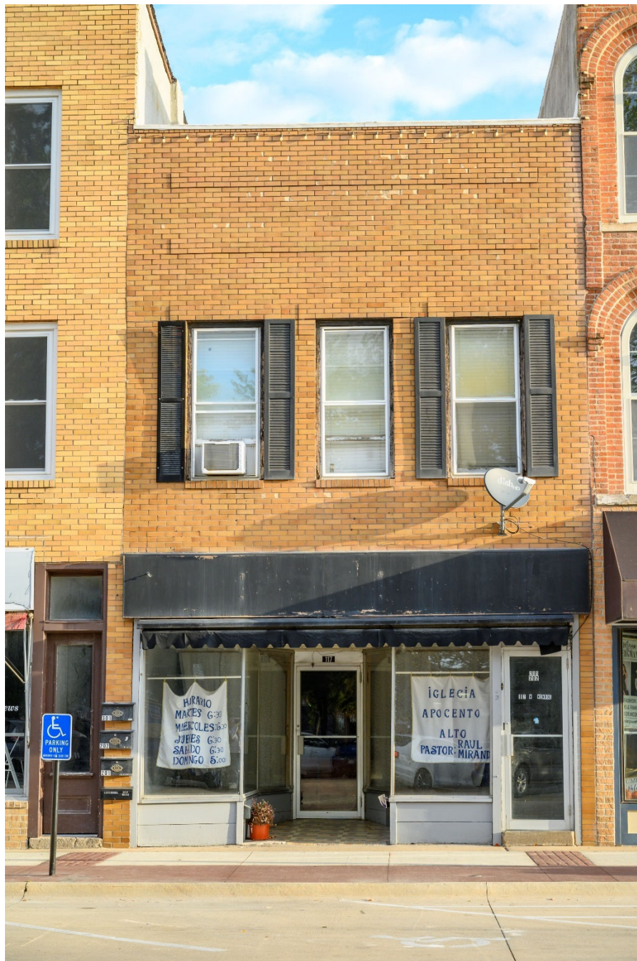
Photograph 44-00370-001. South elevation, looking north (October 2023)
