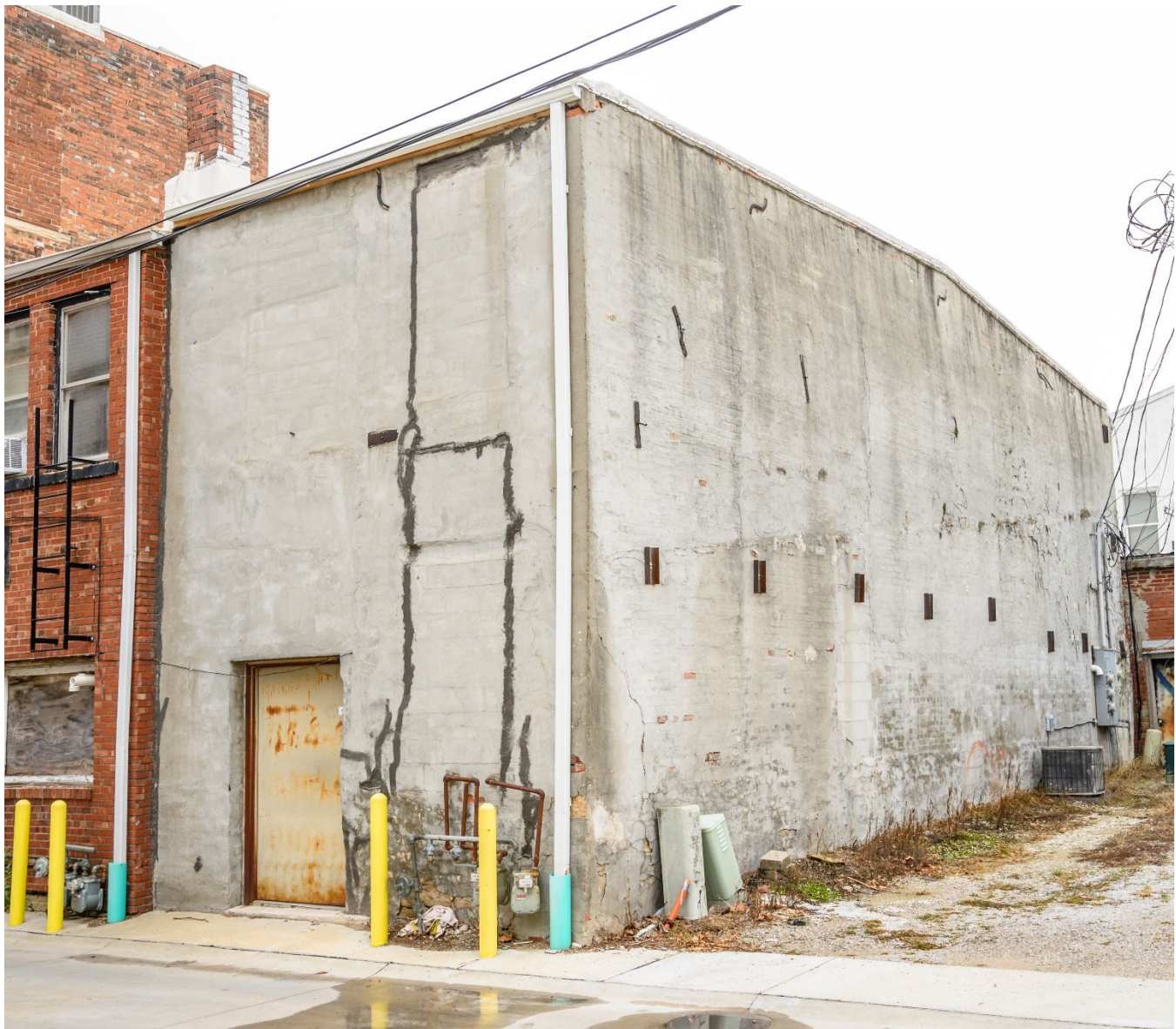
Photograph 44-02263-002. Addition along north elevation to side alley, looking southwest (October 2023)
