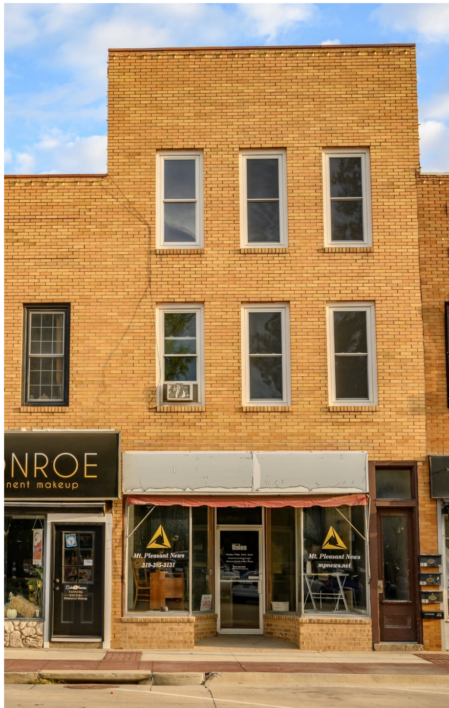
Photograph 44-02263-001. South elevation, looking north (October 2023)
