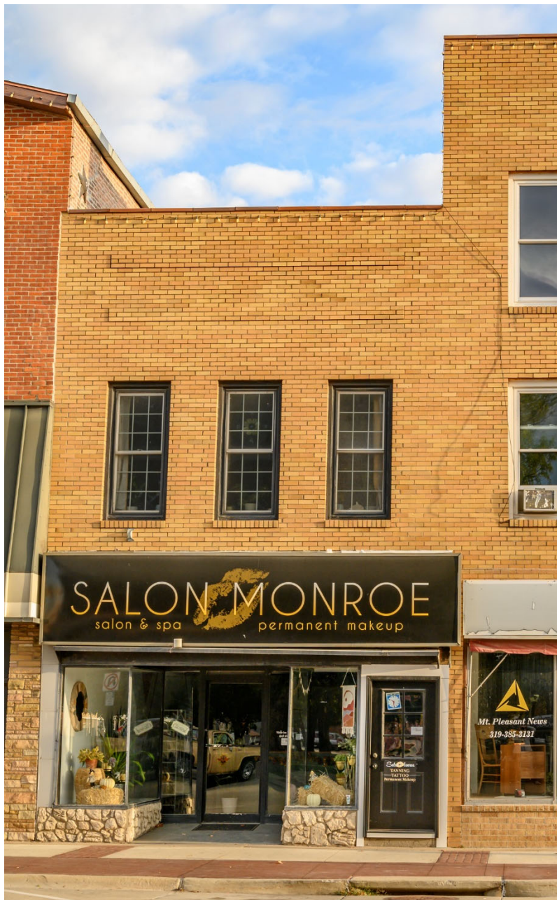
Photograph 44-00371-001. South elevation, looking north (October 2023)
