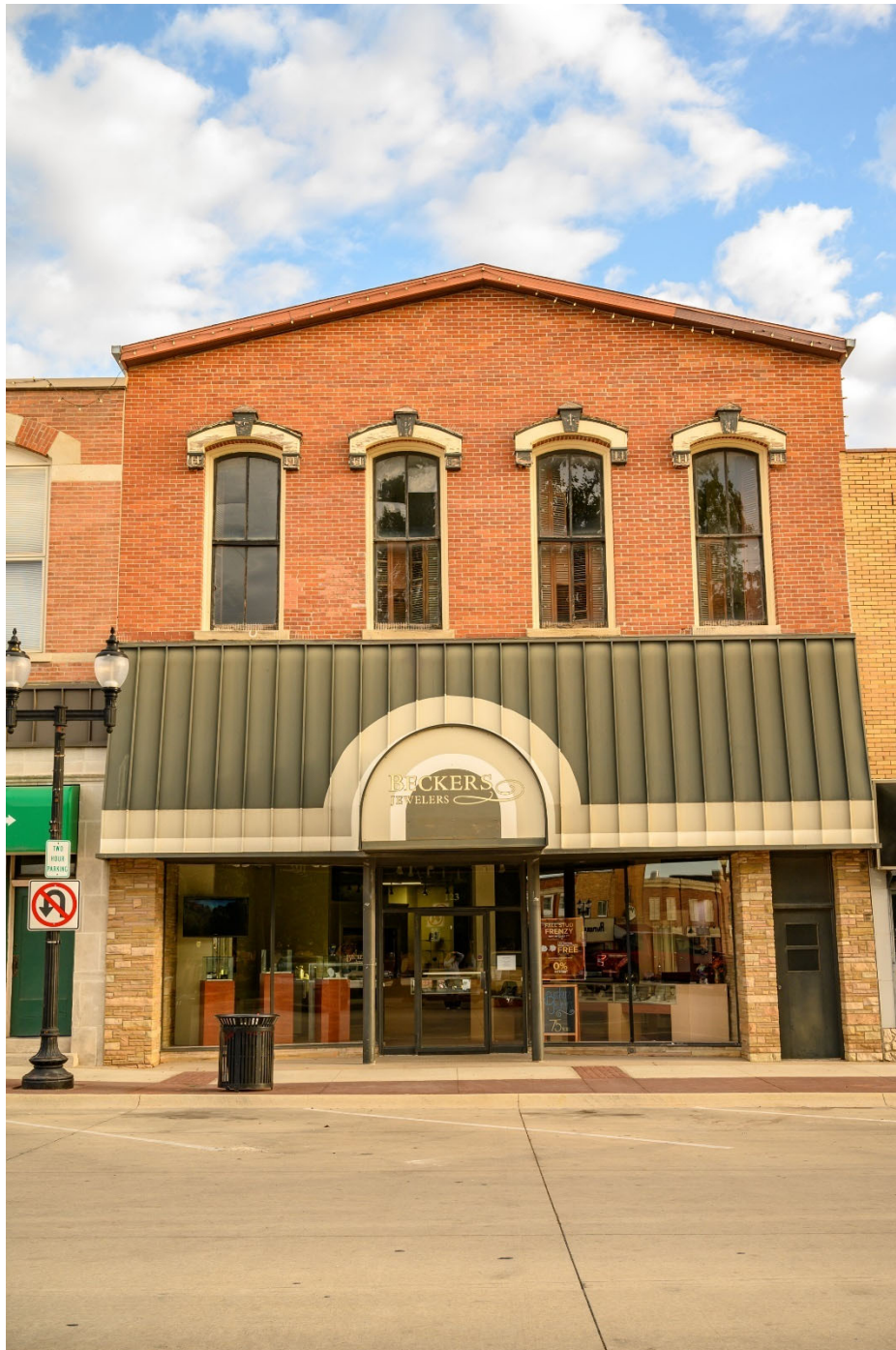
Photograph 44-00372-001. South elevation, looking north (October 2023)
