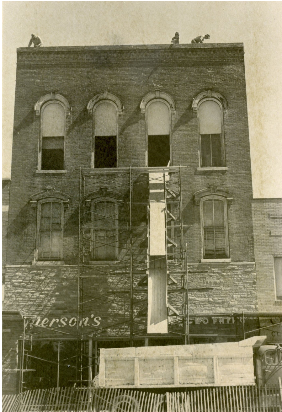
Chute system for removal of third story in 1981 (photo from HCHT Facebook album, also published in Mt Pleasant Journal , June 25, 1981)
