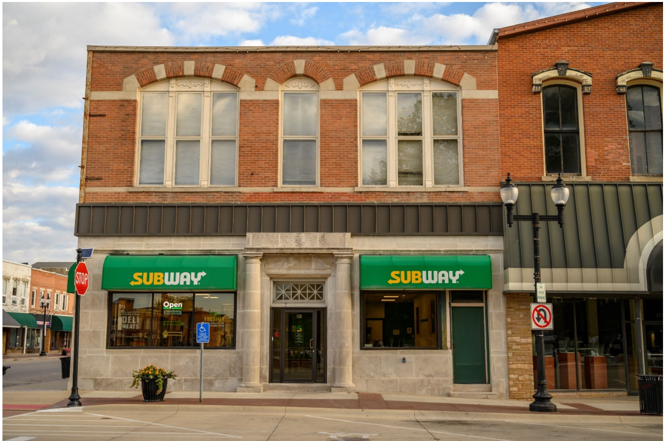
Photograph 44-00373-001. South elevation, looking north (October 2023)
