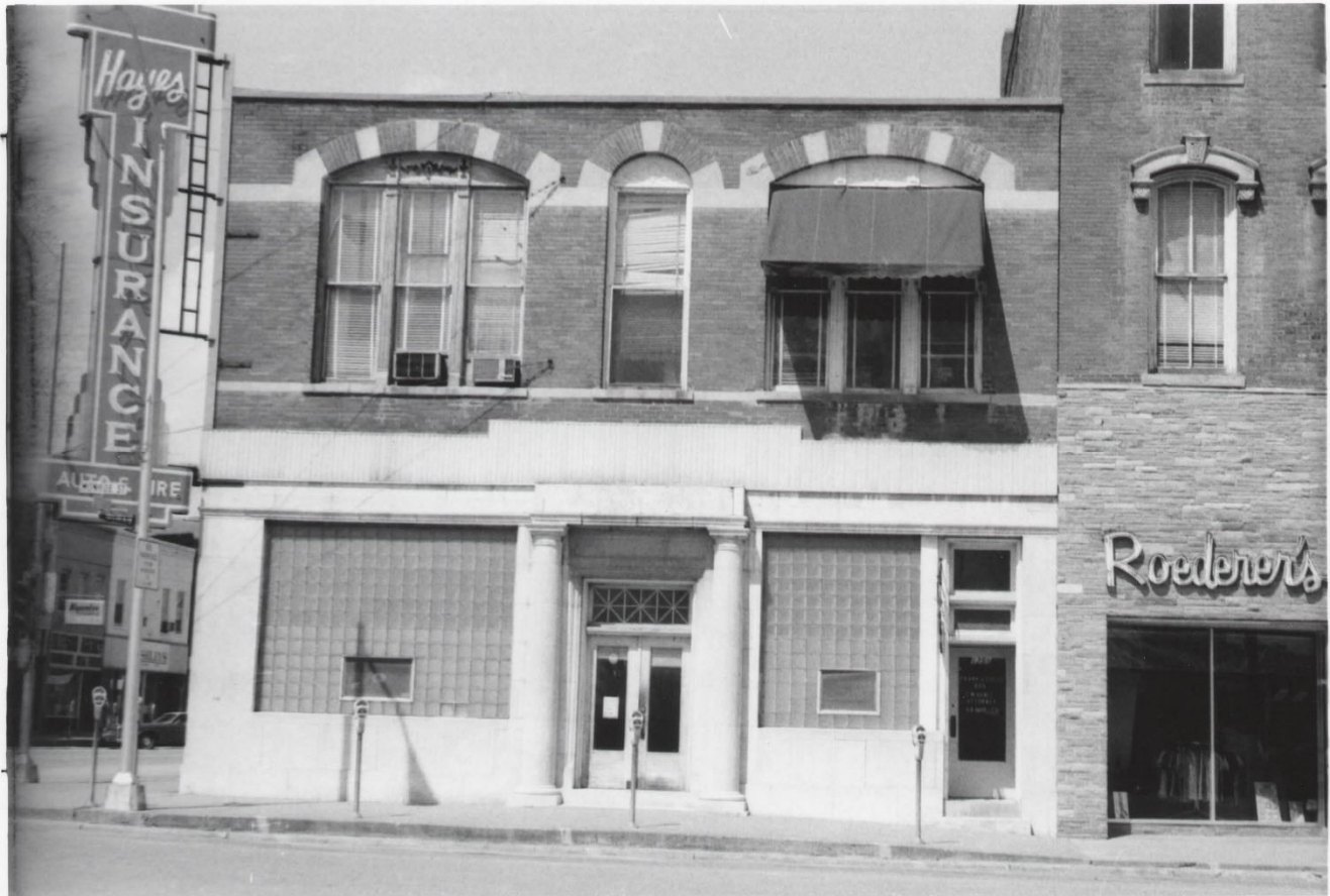
Building in early 1970s (HCHT files)
