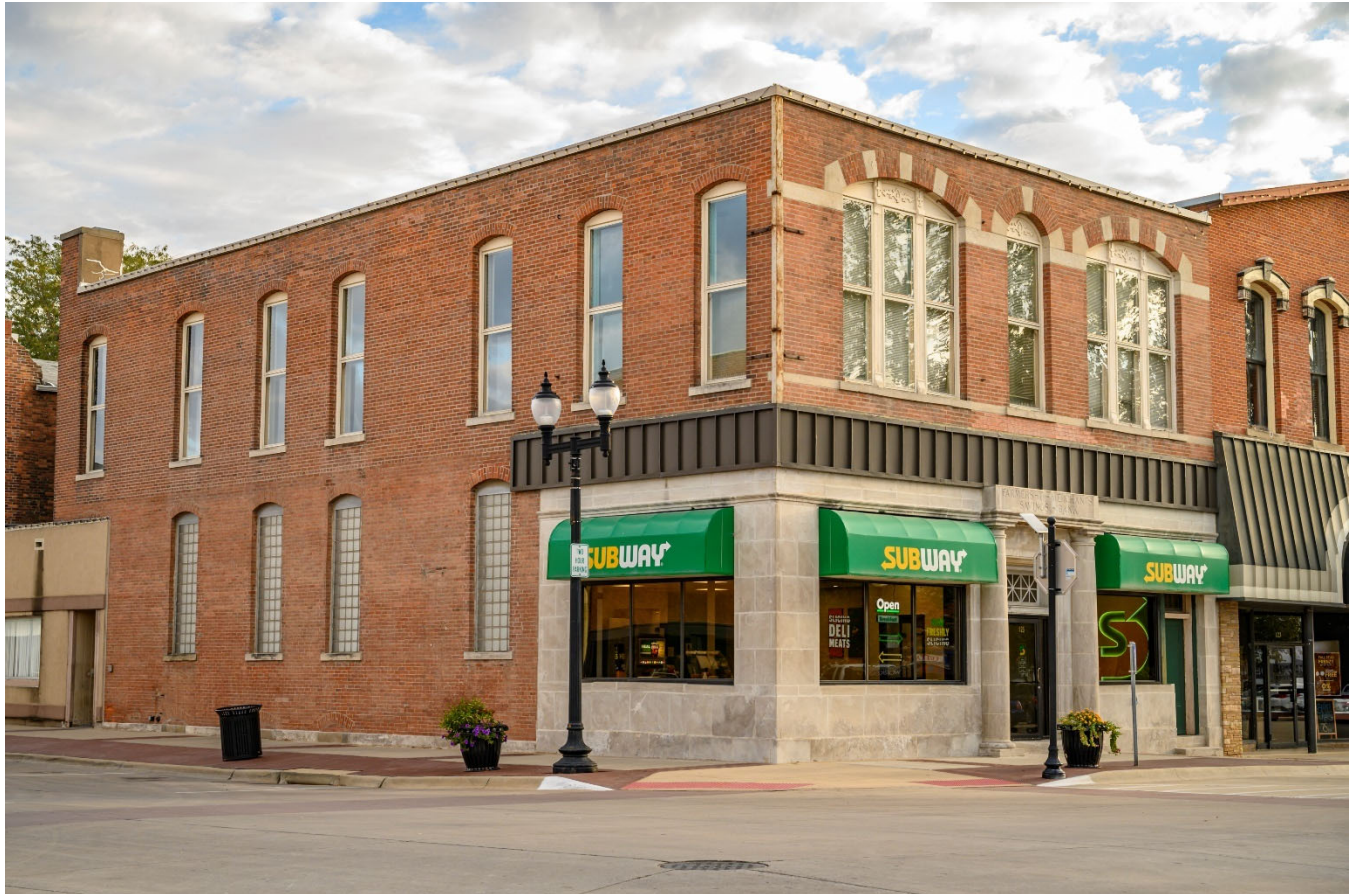
Photograph 44-00373-002. West and south elevations, looking northeast (October 2023)
