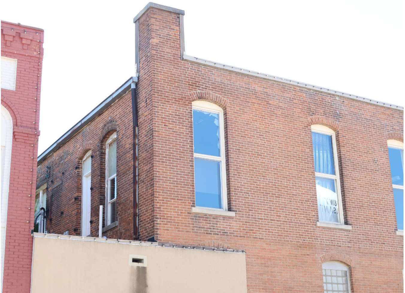
Photograph 44-00373-004. North elevation, looking southeast (June 2024)
