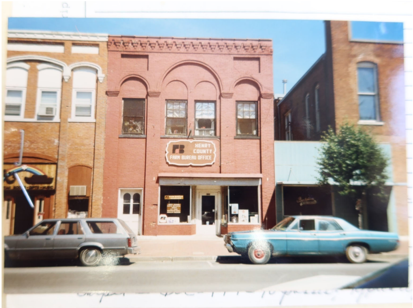
Building in May 1988 (City of Mt Pleasant building permits)
