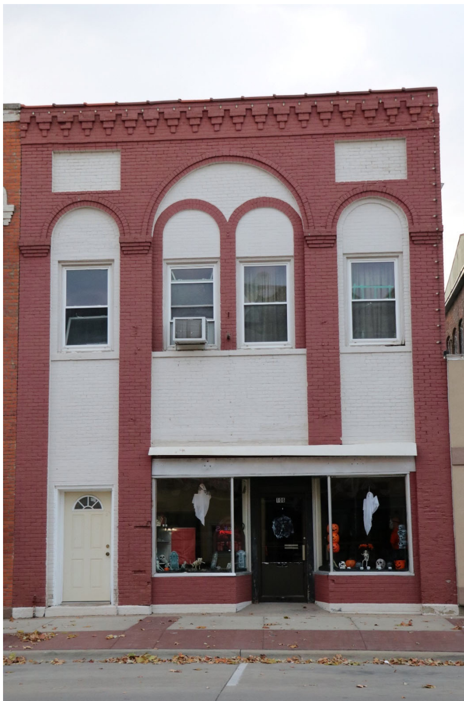
Photograph 44-00186-001. West elevation, looking east (October 2023)
