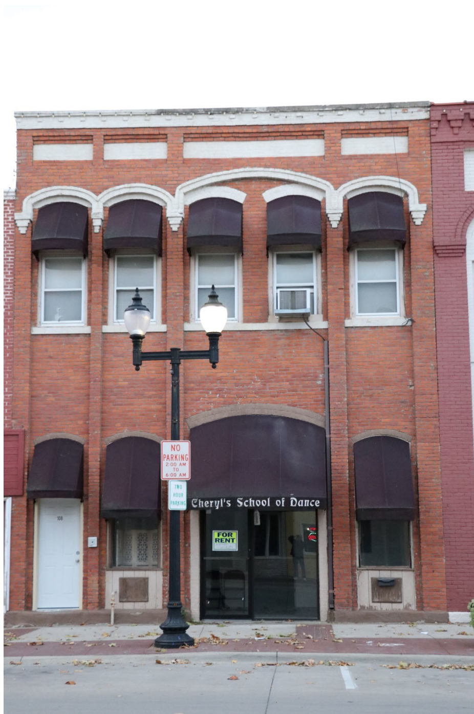
Photograph 44-00187-002. West elevation, looking east (October 2023)
