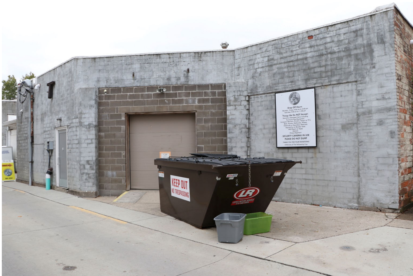
Photograph 44-00191-004. East elevation, looking southwest (October 2023)
