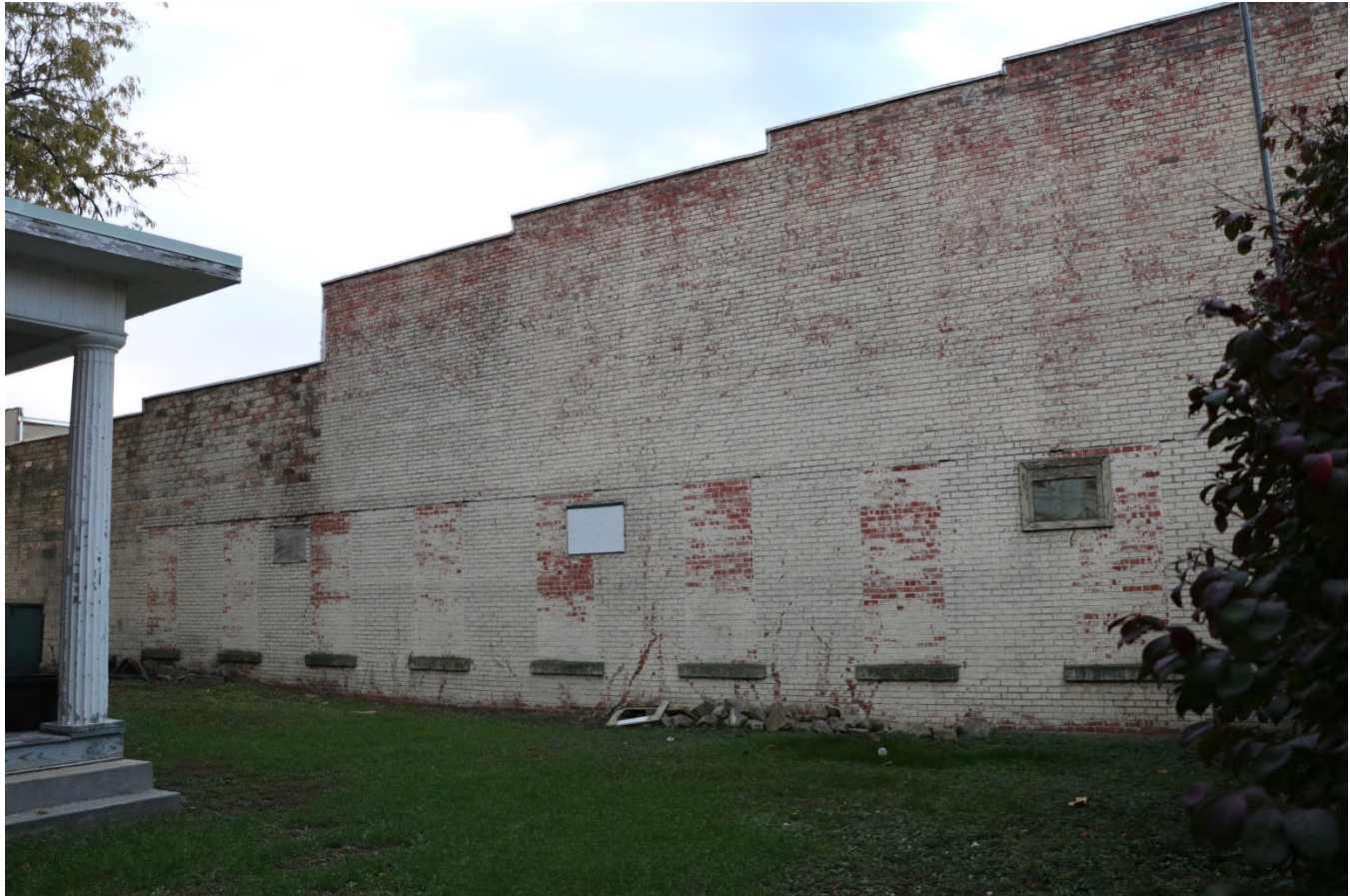
Photograph 44-00191-002. North elevation, looking southeast (October 2023)
