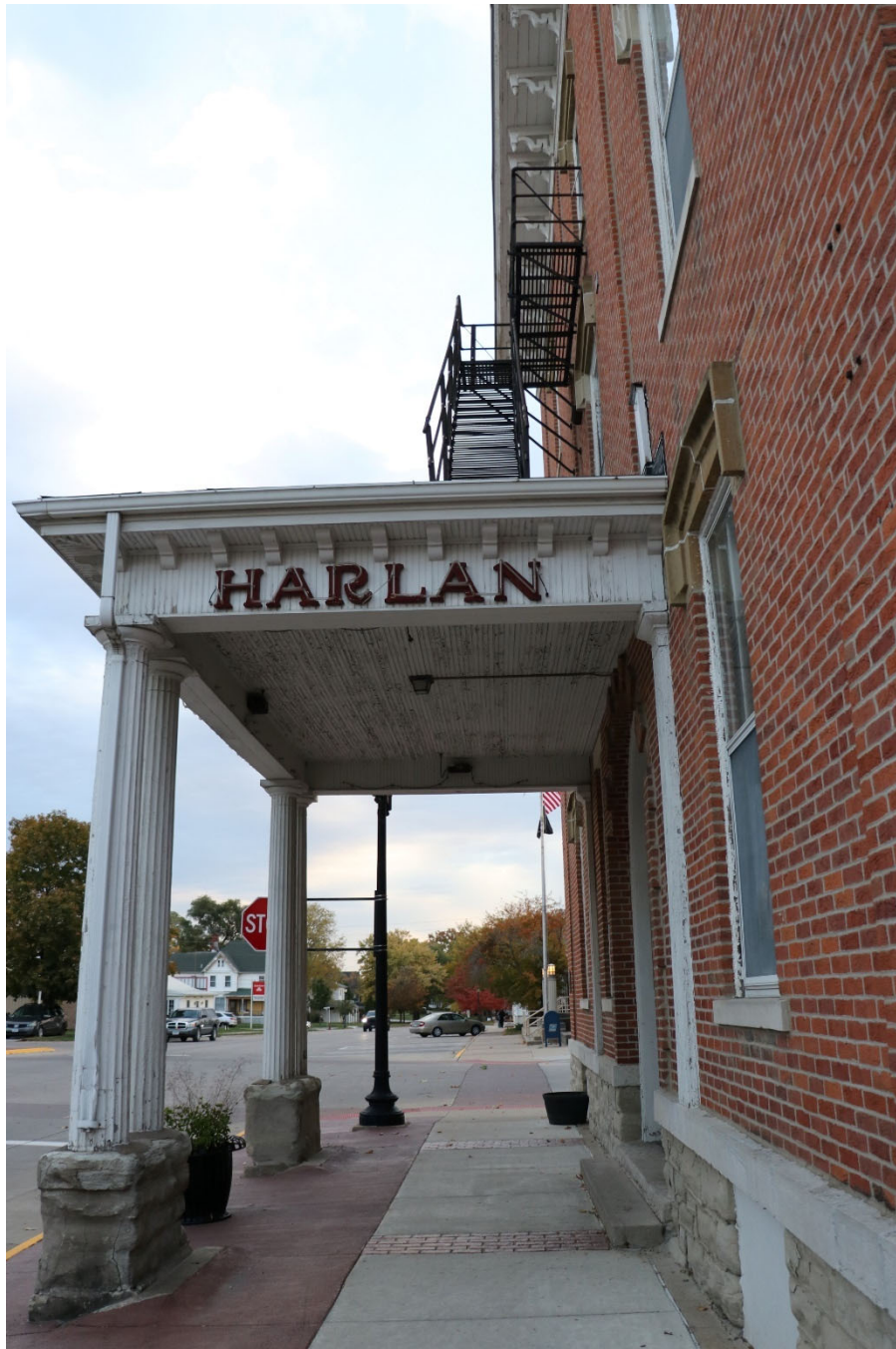
Photograph 44-00196-004. Detail of portico on west elevation, looking north (October 2023)
