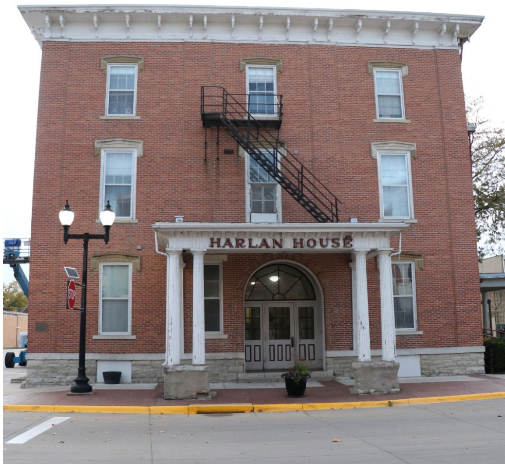
Photograph 44-00196-001. West elevation, looking east (October 2023)
