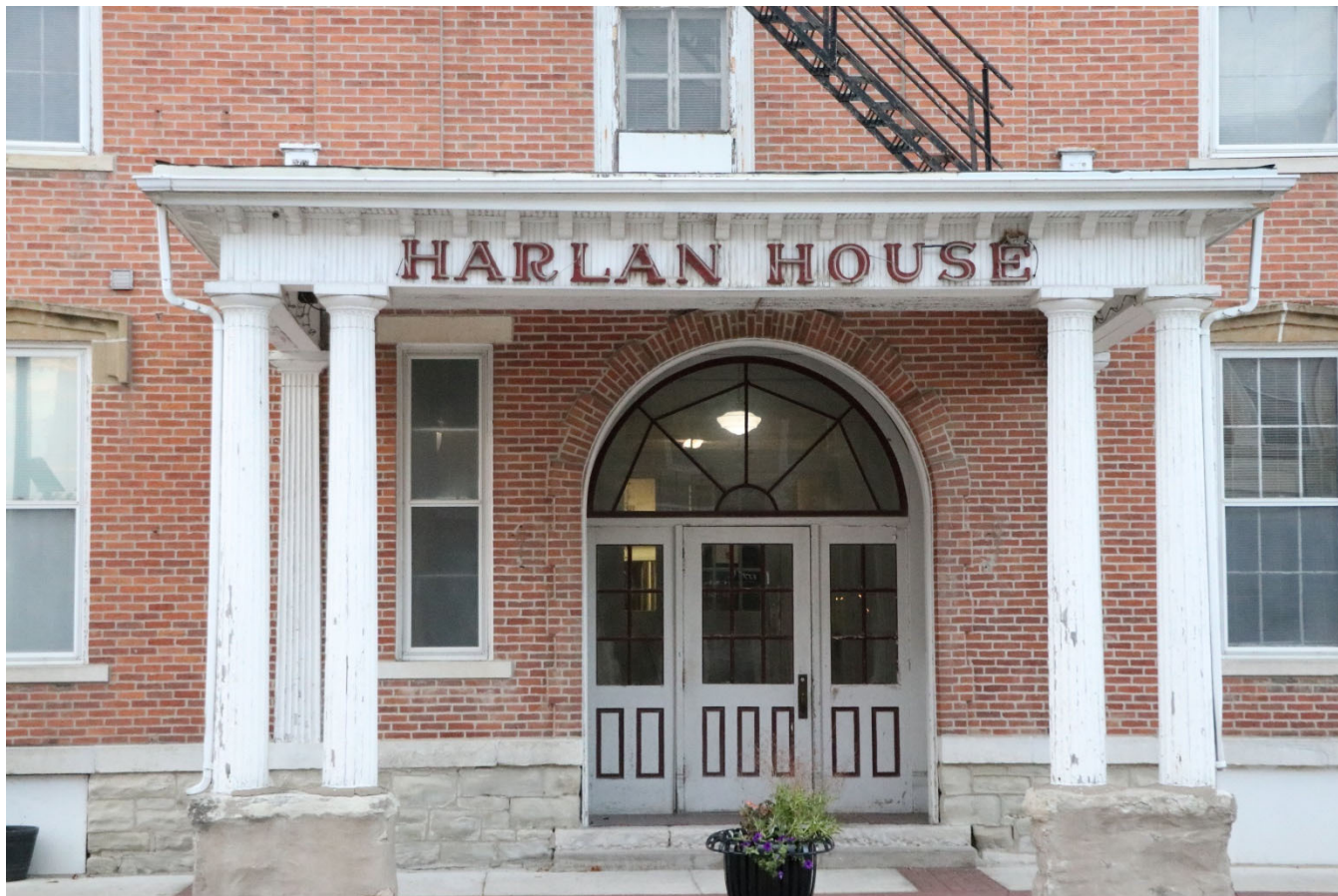
Photograph 44-00196-002. Detail of entry on west elevation, looking east (October 2023)
