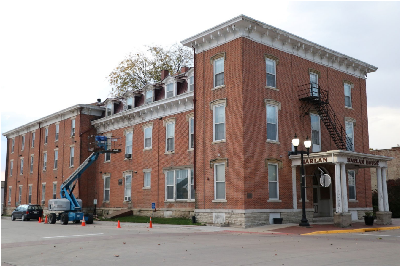
Photograph 44-00196-005. North and west elevations, looking southeast (October 2023)
