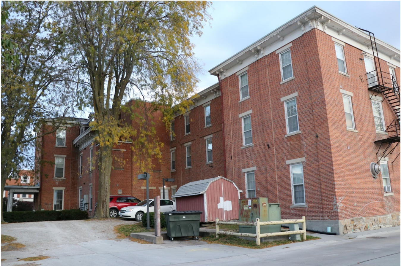
Photograph 44-00196-010. Rear/east portion of south elevation, looking northwest (October 2023)
