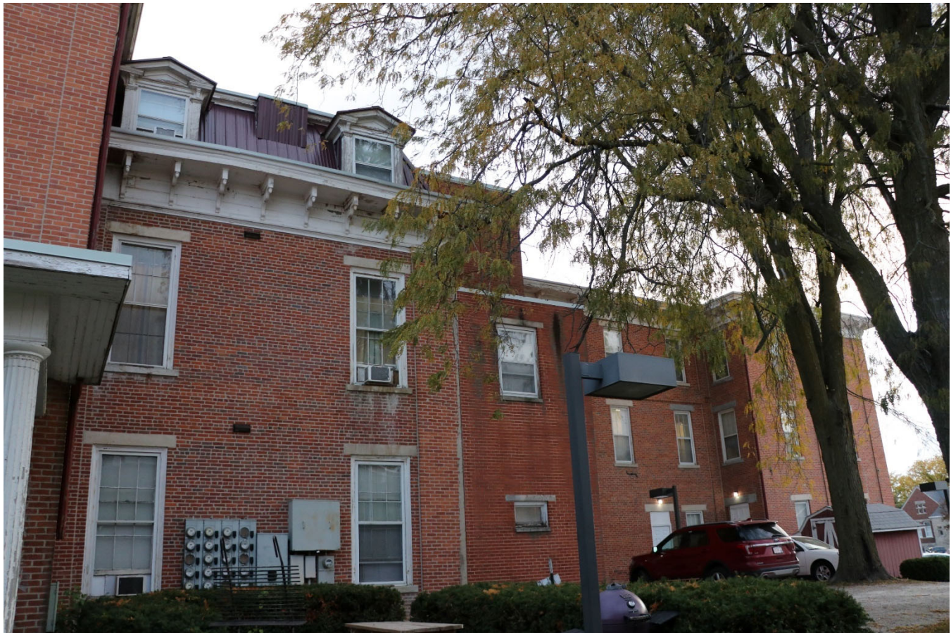
Photograph 44-00196-009. Rear/east portion of south elevation, looking northeast (October 2023)
