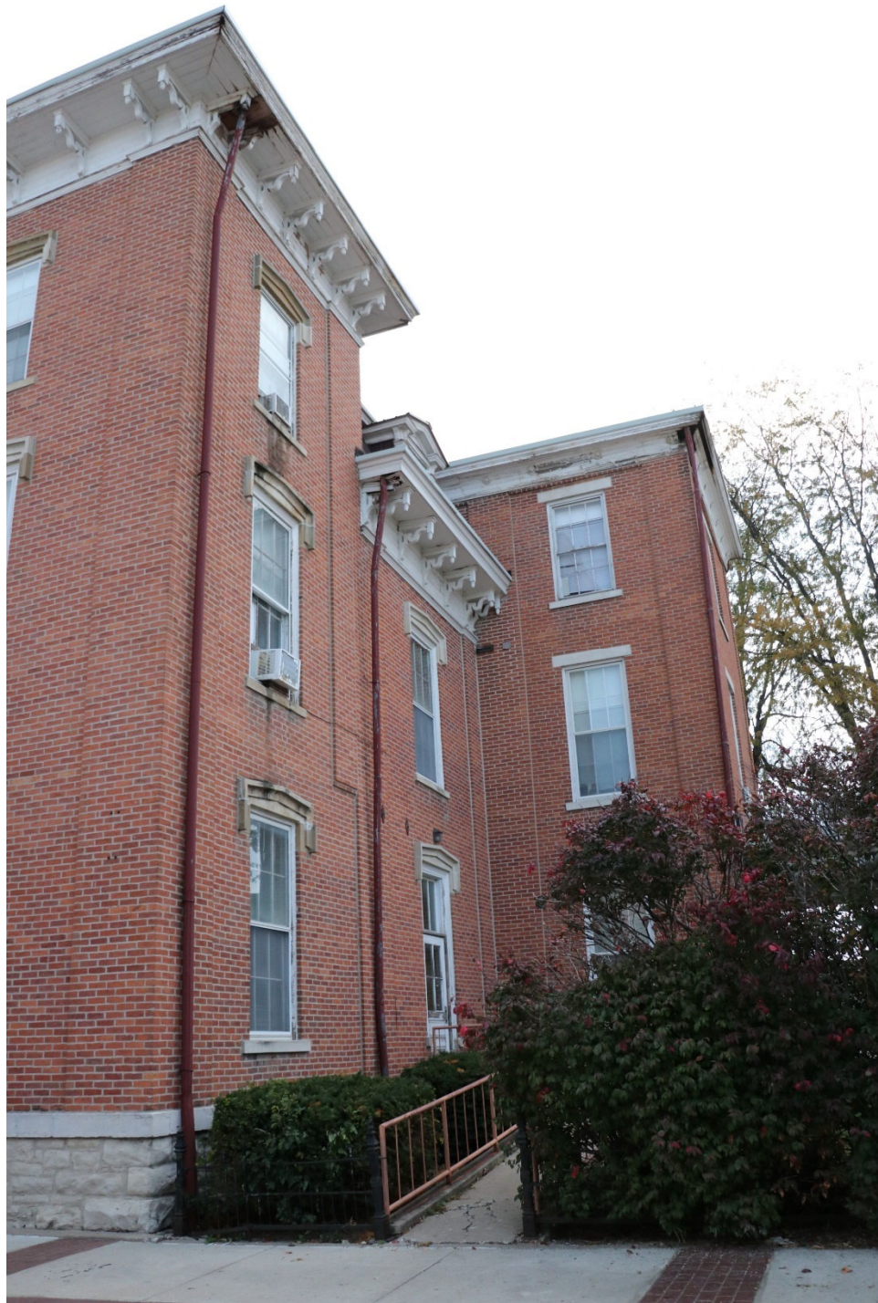
Photograph 44-00196-007. South elevation, looking northeast (October 2023)
