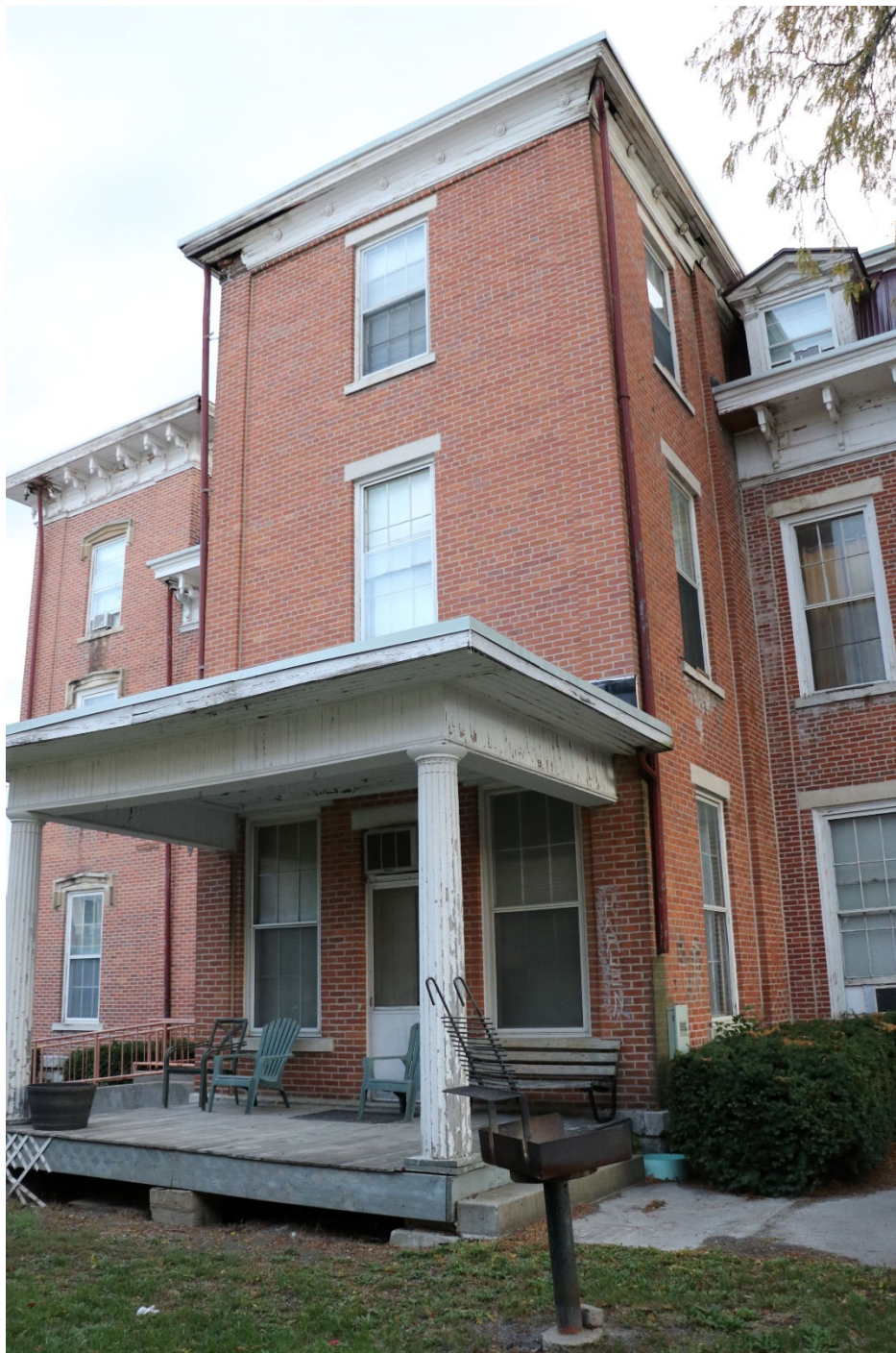
Photograph 44-00196-008. South elevation, looking northwest (October 2023)
