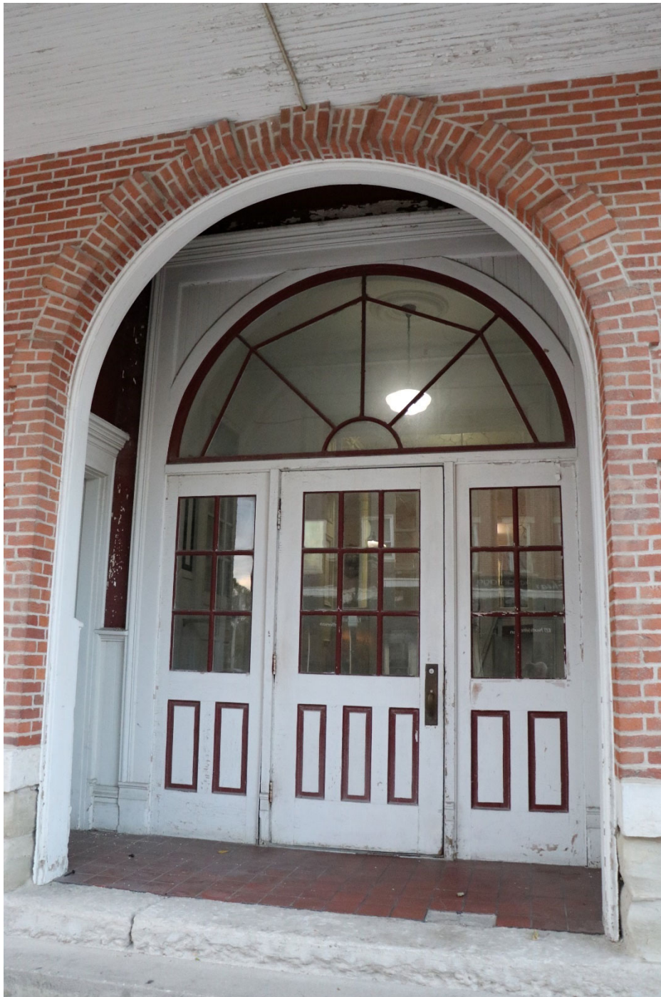
Photograph 44-00196-003. Detail of entry on west elevation, looking east (October 2023)
