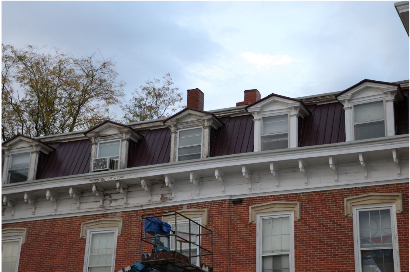
Photograph 44-00196-006. Detail of roof and dormers on north elevation, looking south (October 2023)
