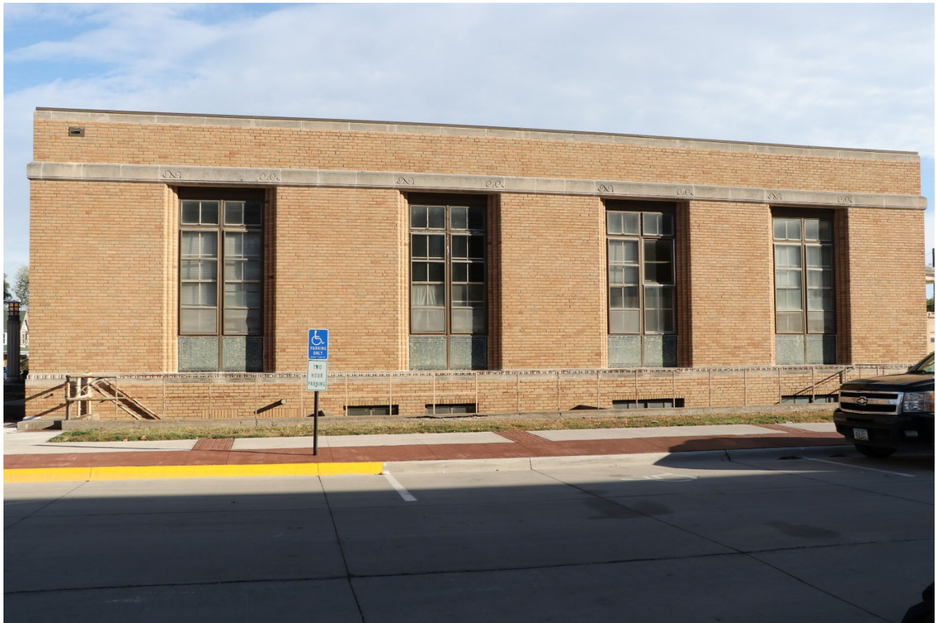
Photograph 44-00786-003. South elevation, looking north (October 2023)
