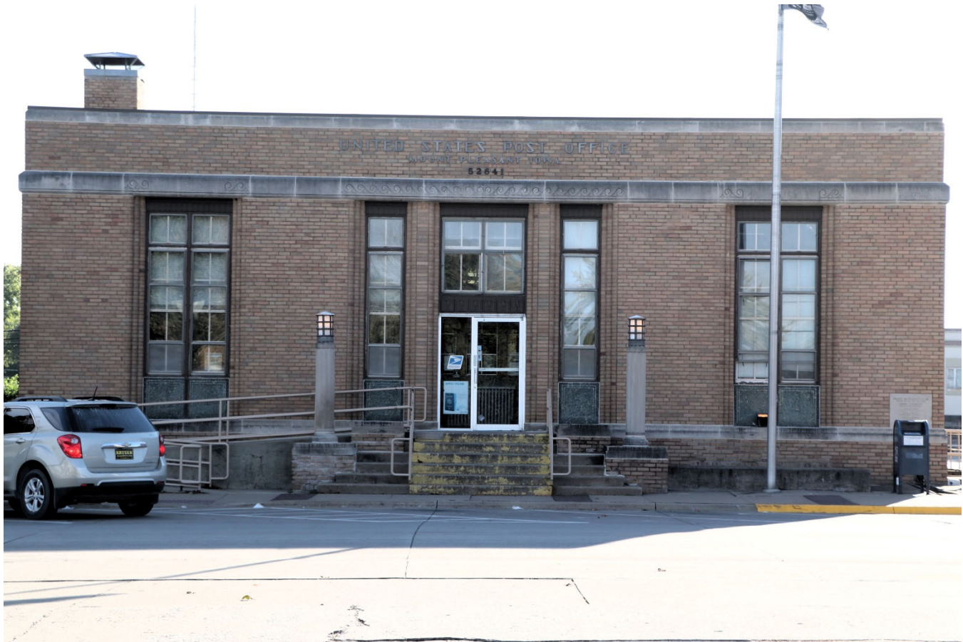
Photograph 44-00786-002. West elevation, looking east (October 2023)
