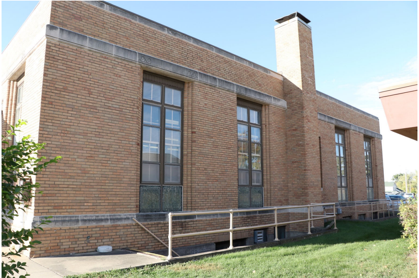
Photograph 44-00786-004. North elevation, looking southwest (October 2023)
