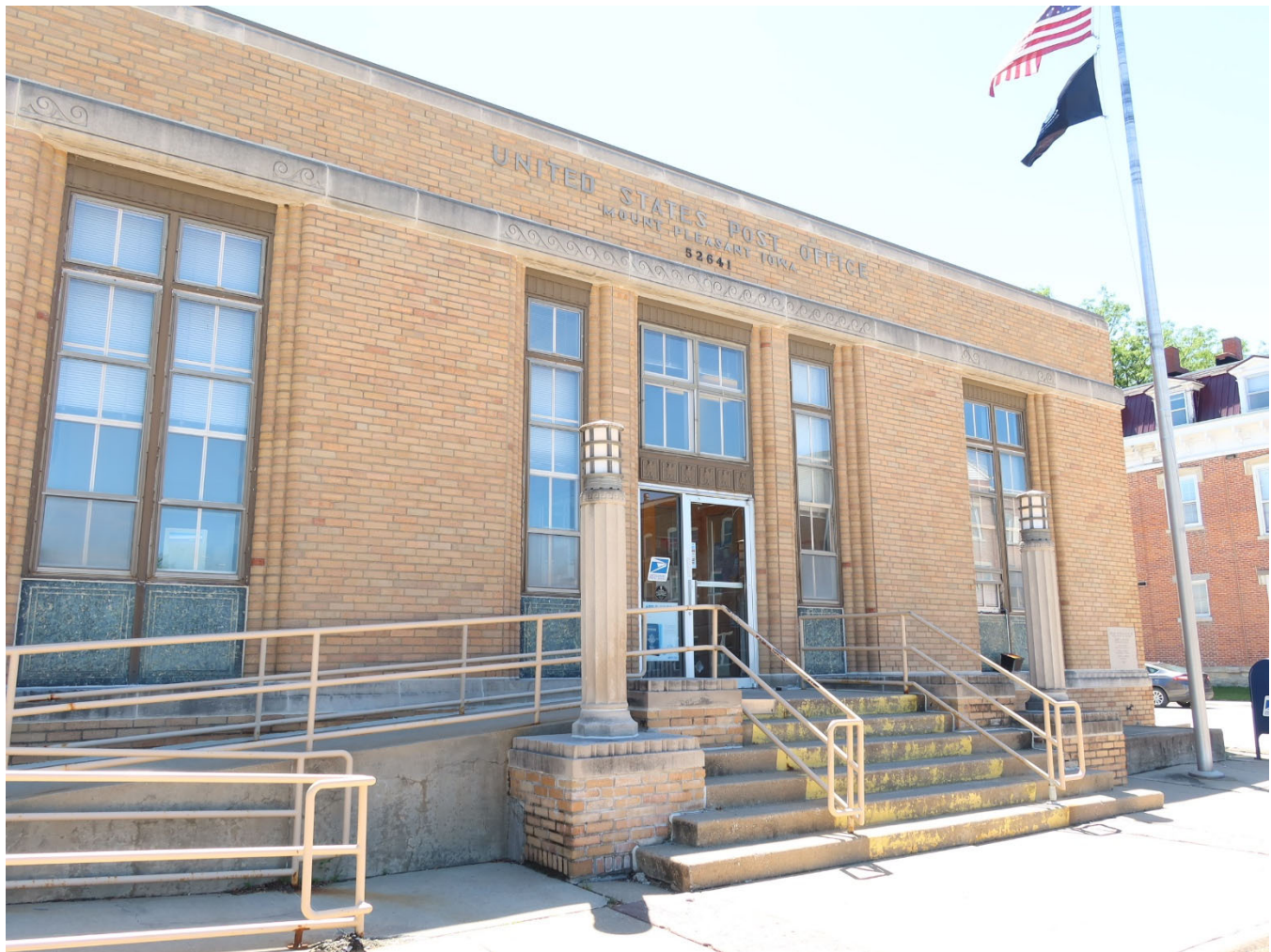
Photograph 44-00786-001. West elevation, looking southeast (June 2024)
