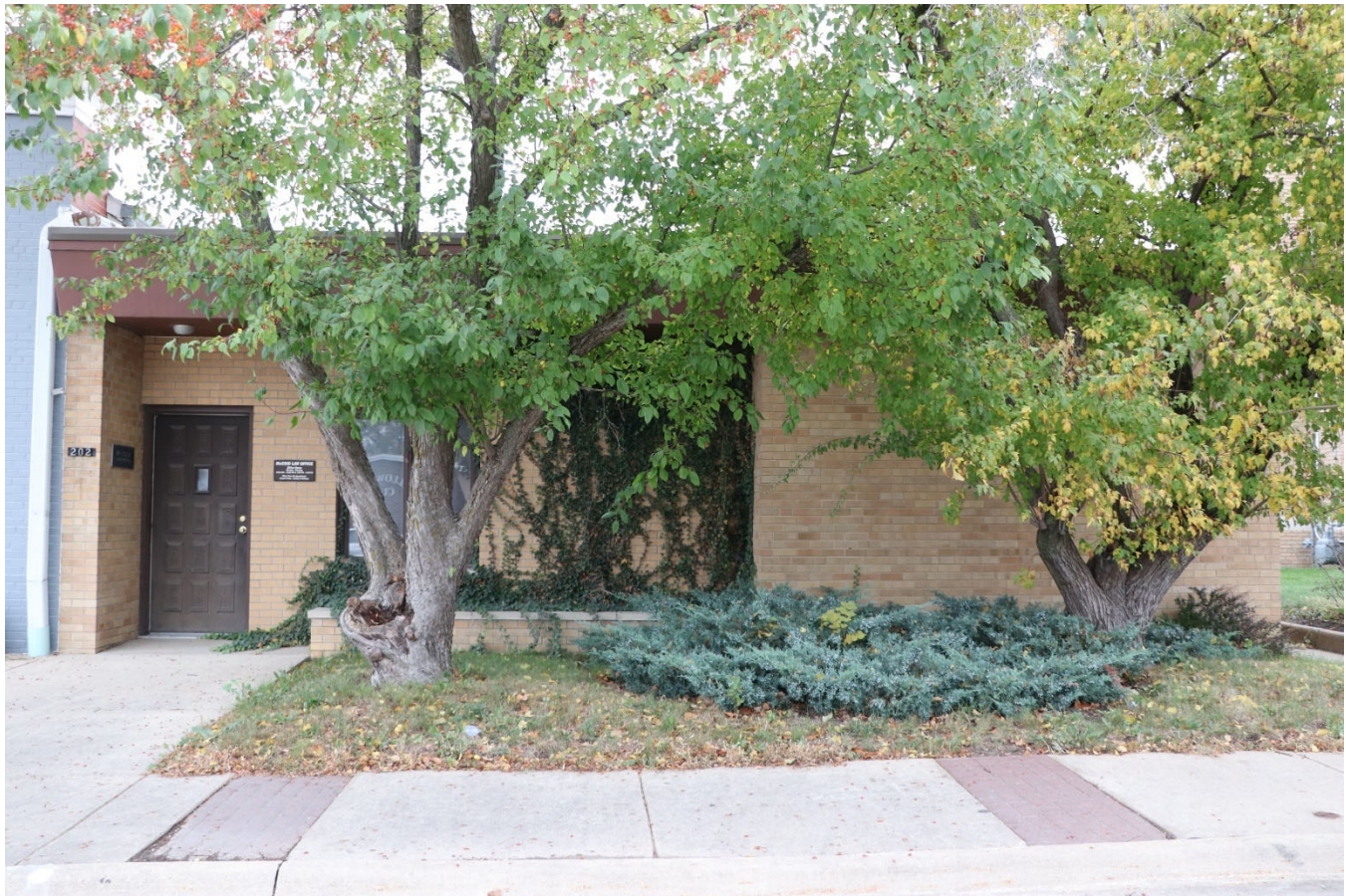
Photograph 44-02243-001. West elevation, looking east (October 2023)
