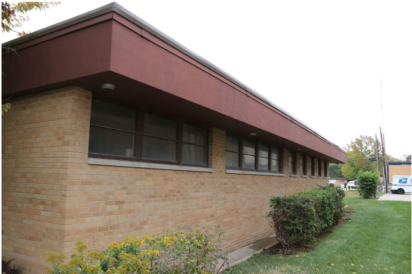
Photograph 44-02243-002. South elevation, looking northeast (October 2023)
