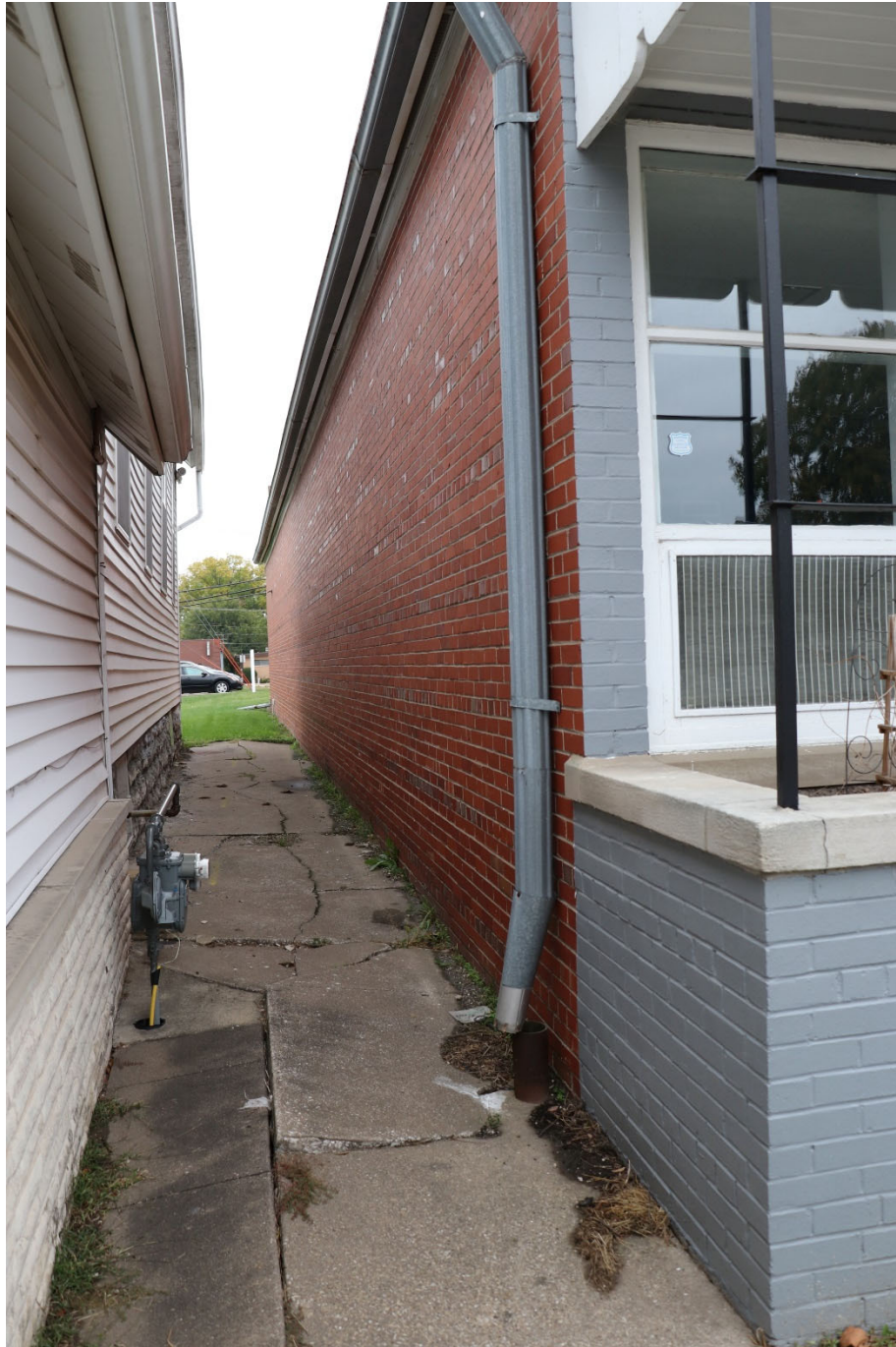
Photograph 44-02244-002. North elevation, looking southeast (October 2023)
