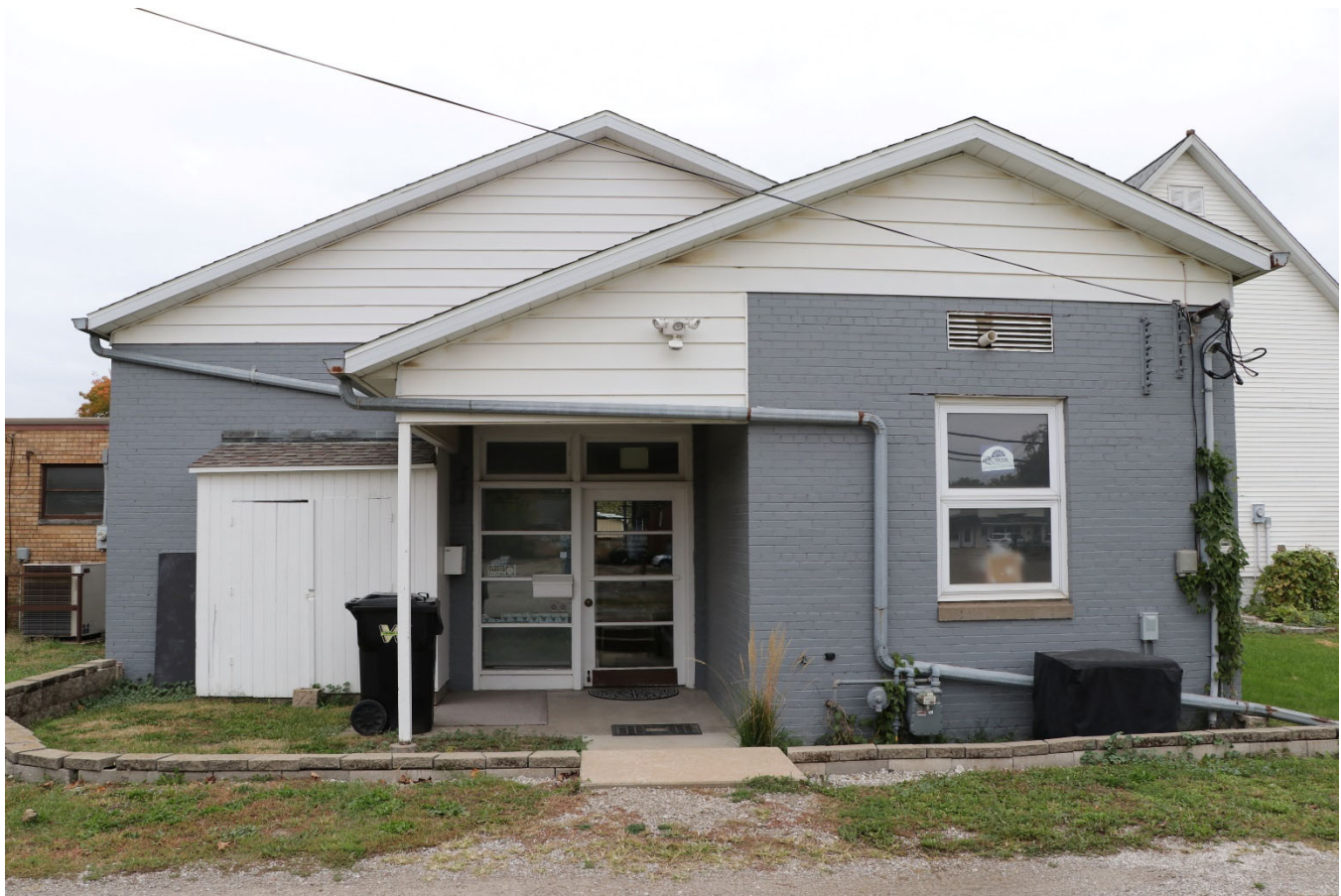
Photograph 44-02244-004. East elevation, looking west (October 2023)
