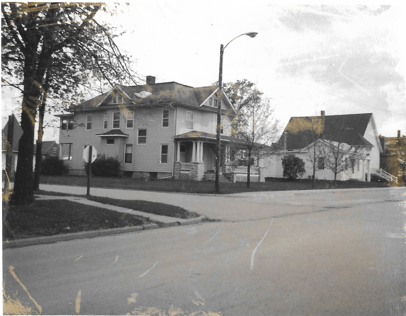
East side of 200 block of N. Jefferson in 1971 prior to move of house at corner to south of town (HCHT Facebook album)
