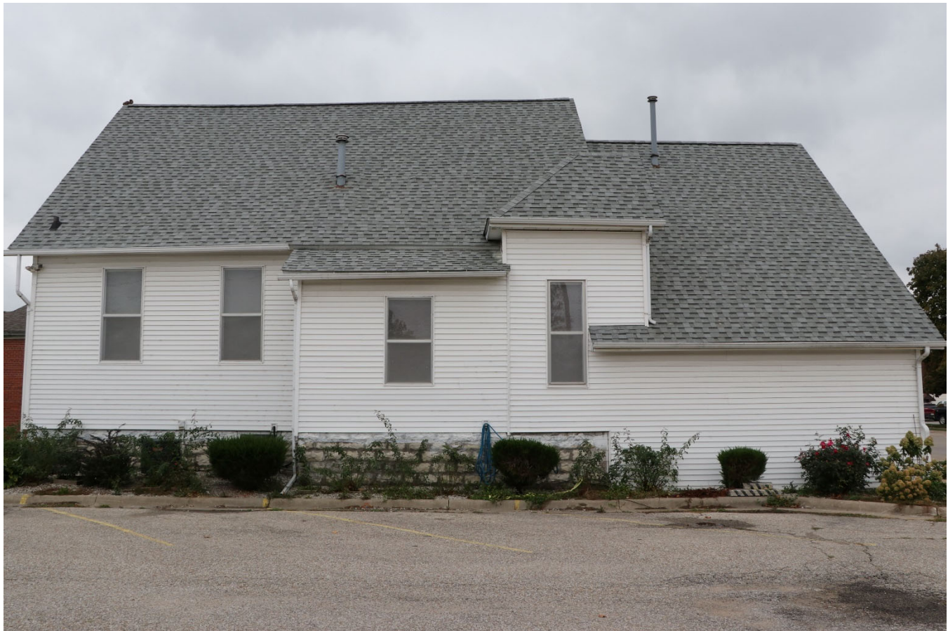
Photograph 44-02245-002. North elevation, looking south (October 2023)
