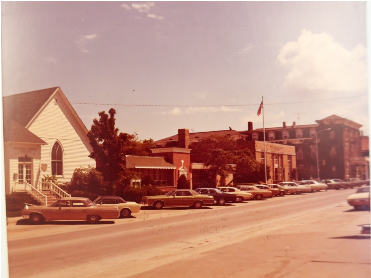
Church at left on east side of 200 block in 1974 (Dyall set, HCHS binder, Mt Pleasant library)
