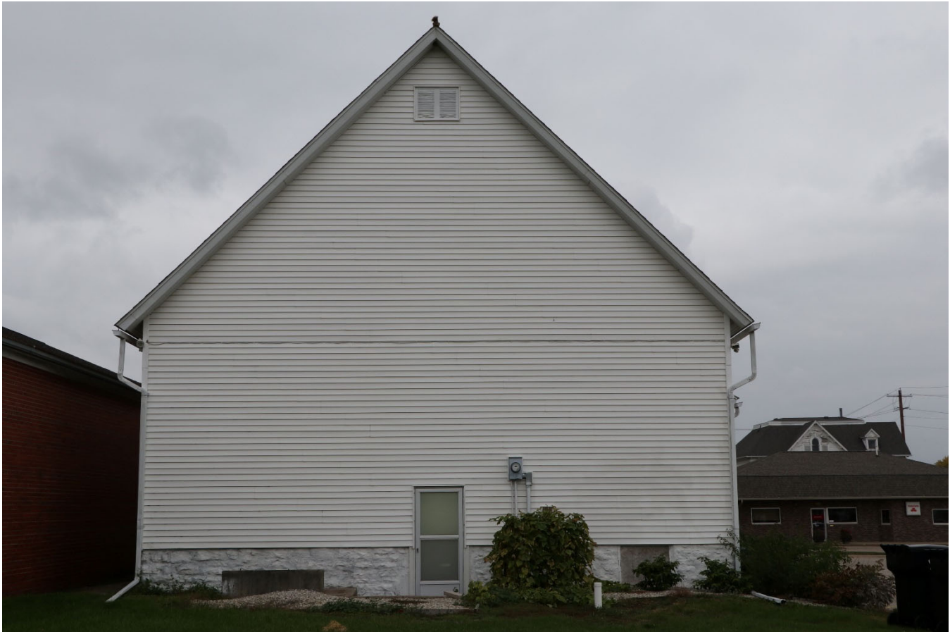
Photograph 44-02245-004. East elevation, looking west (October 2023)
