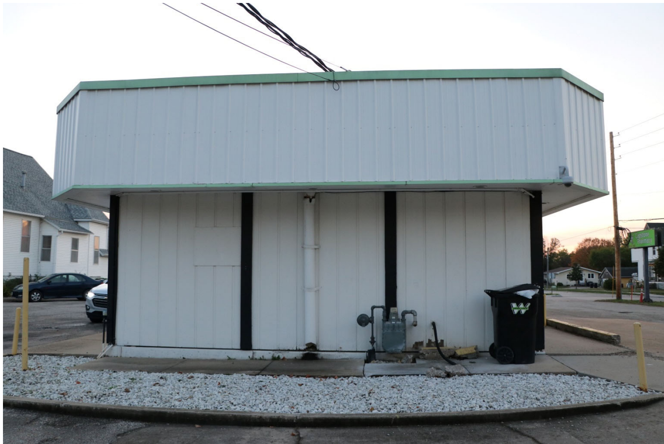
Photograph 44-02246-004. East elevation, looking west (October 2023)
