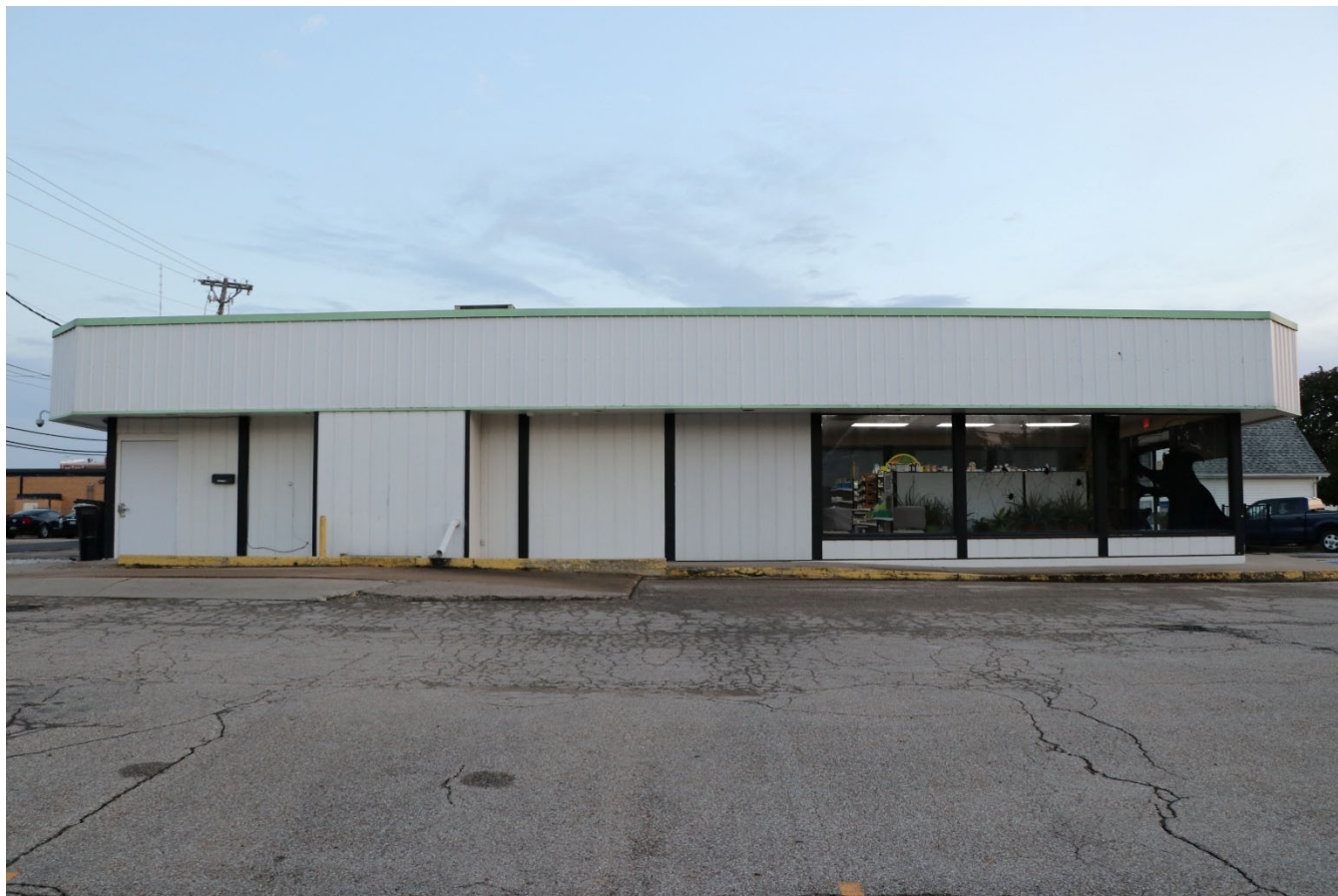
Photograph 44-02246-003. North elevation, looking south (October 2023)
