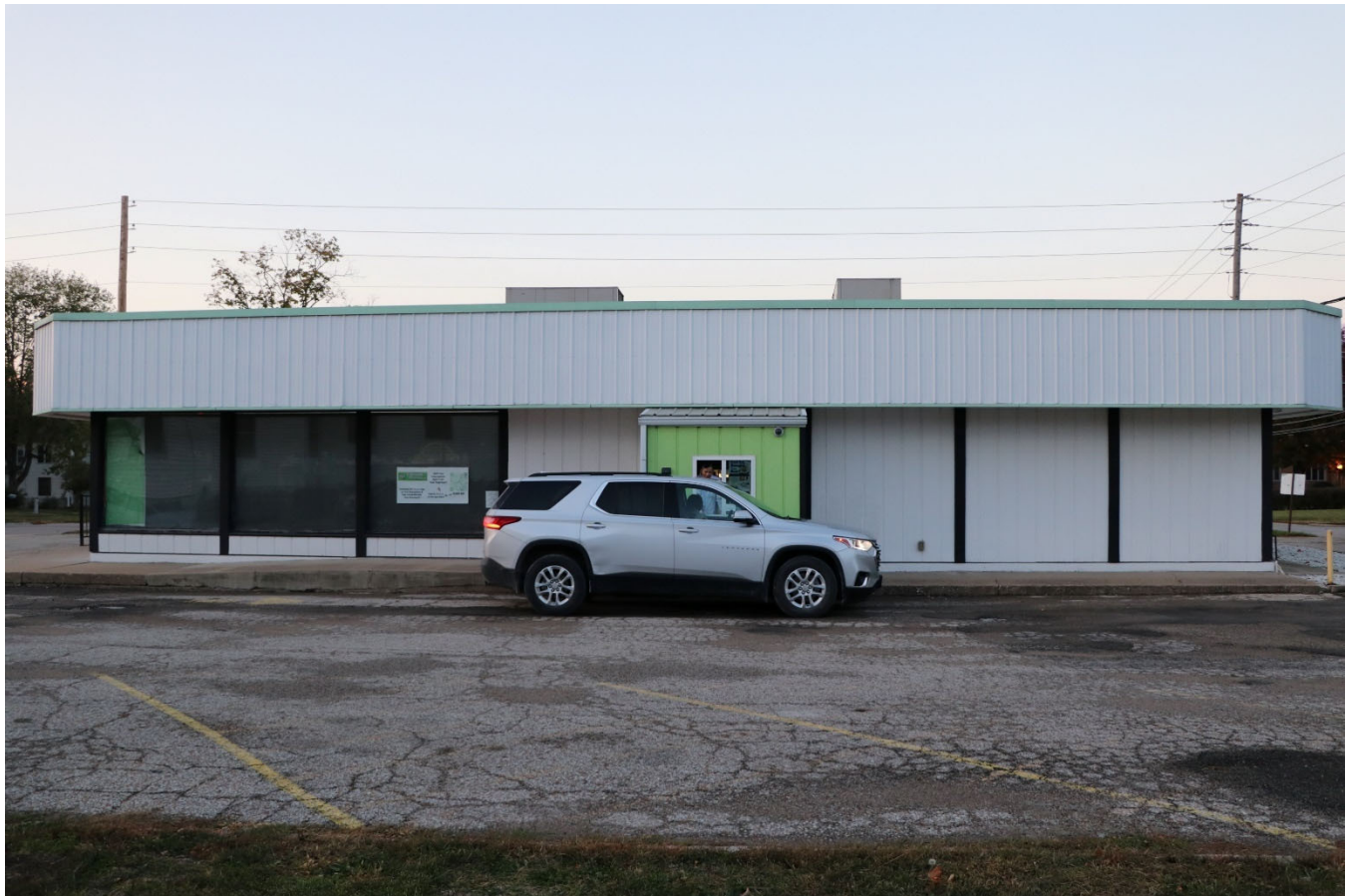
Photograph 44-02246-002. South elevation, looking north (October 2023)
