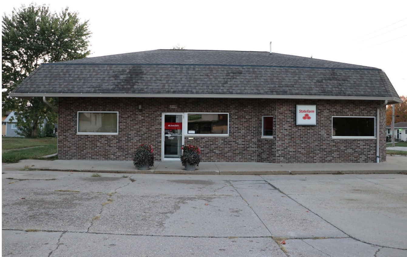
Photograph 44-02249-001. East elevation, looking west (October 2023)
