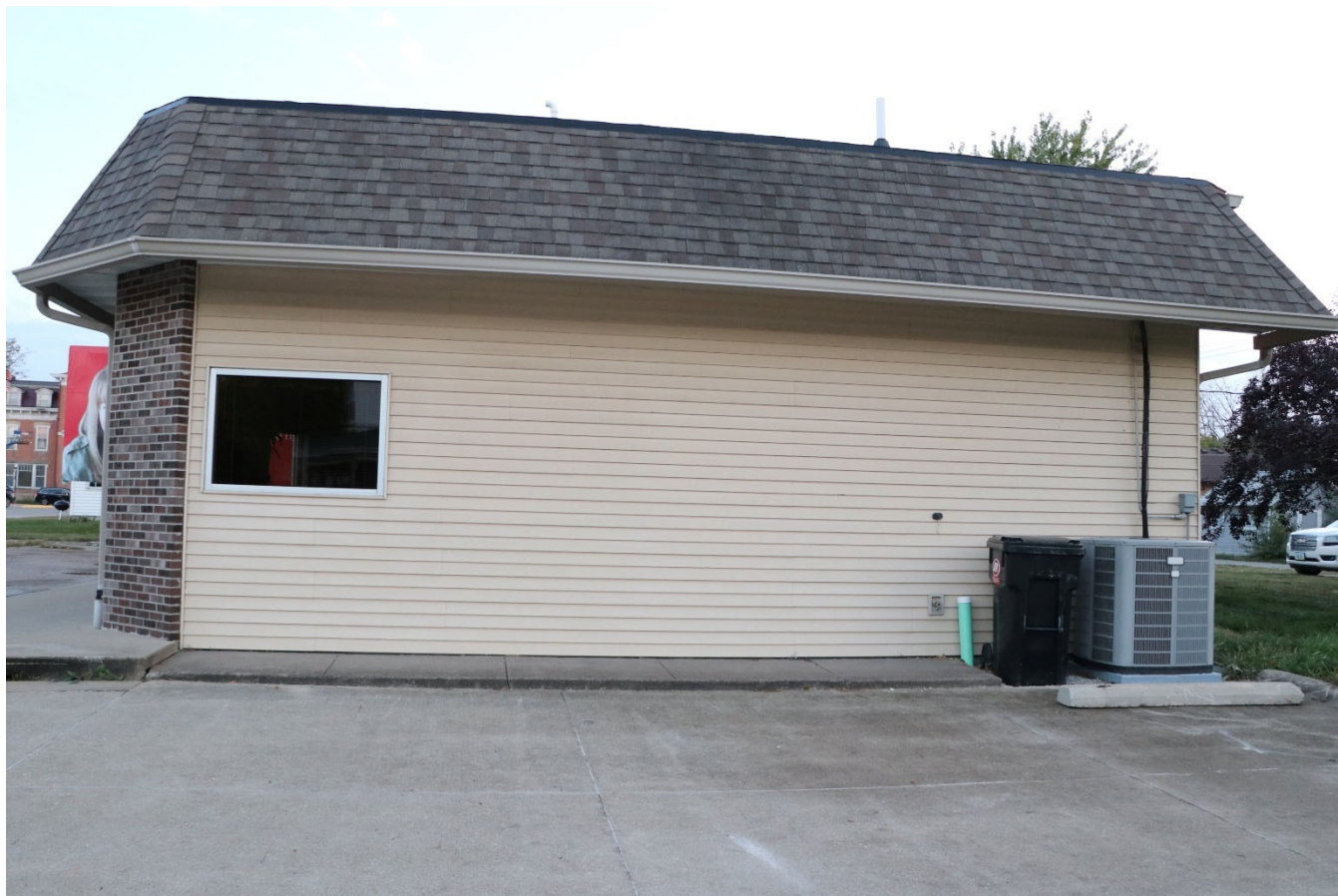
Photograph 44-02249-002. North elevation, looking south (October 2023)
