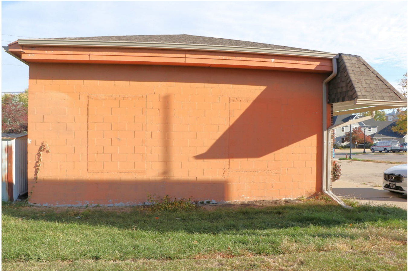
Photograph 44-02249-003. South elevation, looking north (October 2023)
