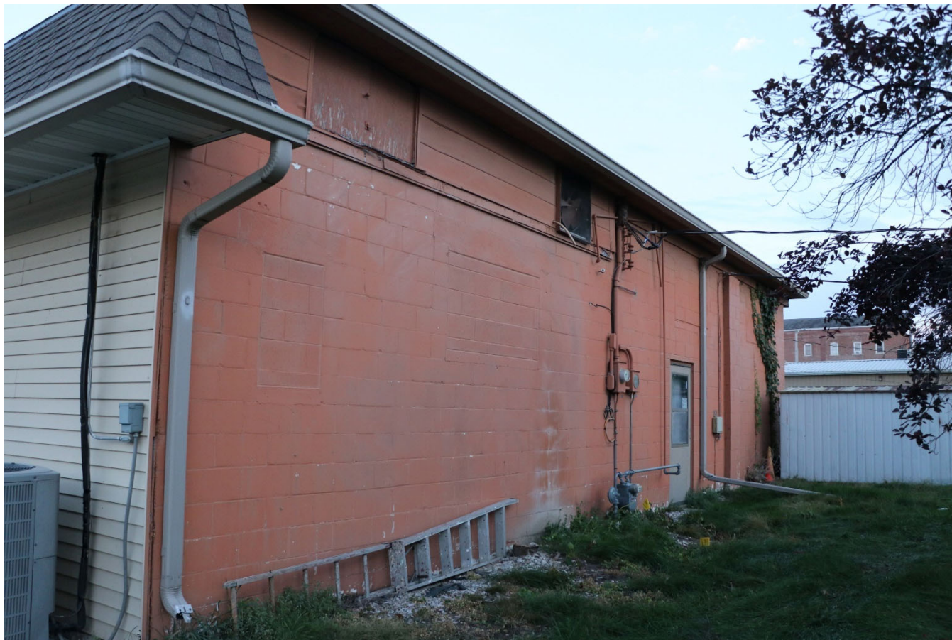
Photograph 44-02249-004. West elevation, looking southeast (October 2023)
