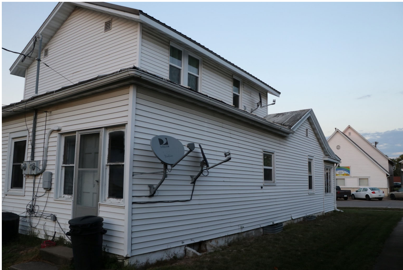
Photograph 44-02248-002. North elevation, looking southwest (October 2023)
