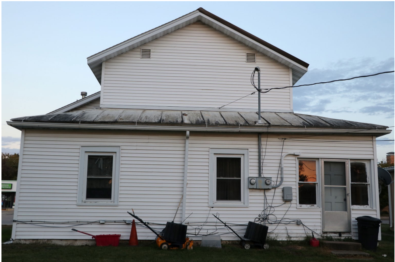
Photograph 44-02248-004. West elevation, looking east (October 2023)
