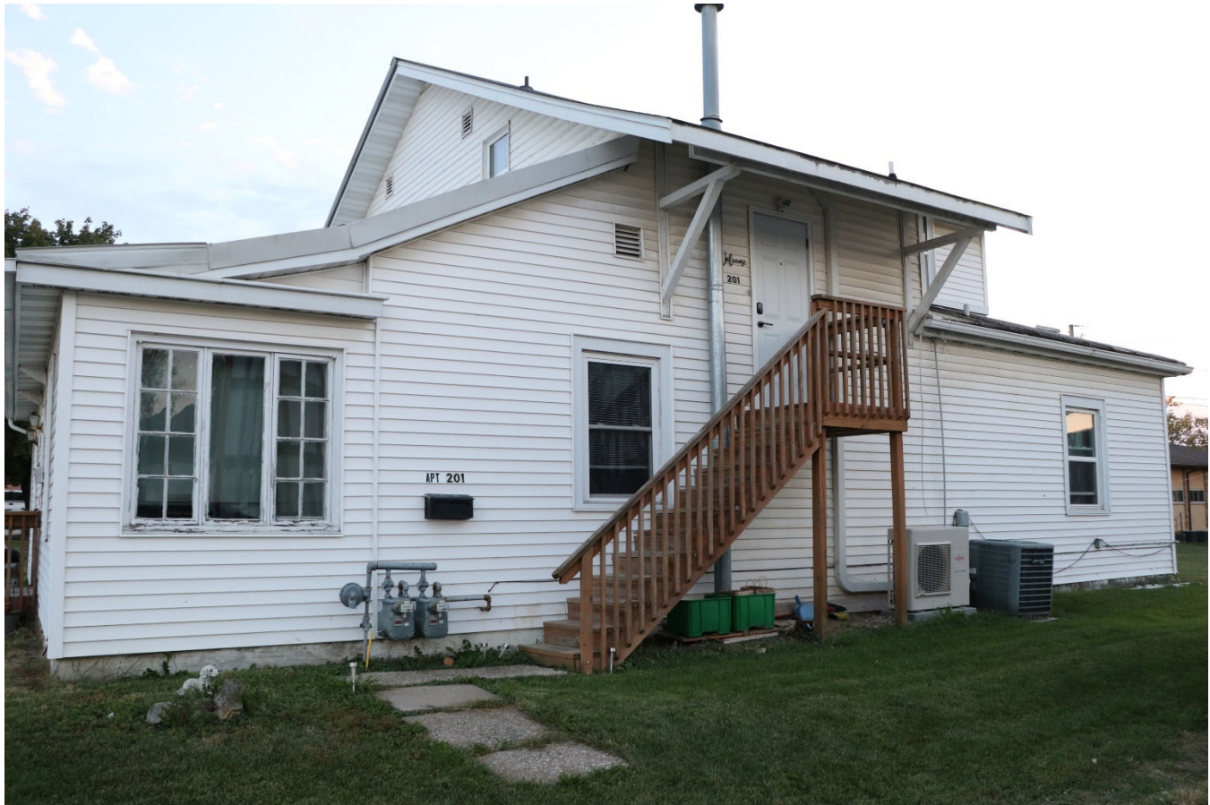
Photograph 44-02248-003. South elevation, looking north (October 2023)
