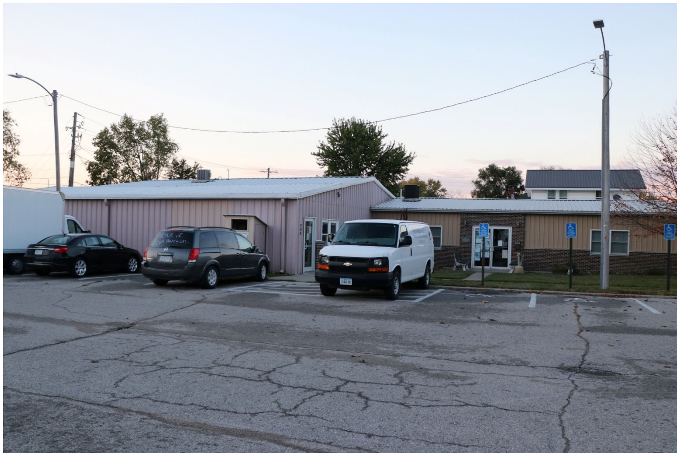
Photograph 44-02247-003. South elevation, looking north (October 2023)
