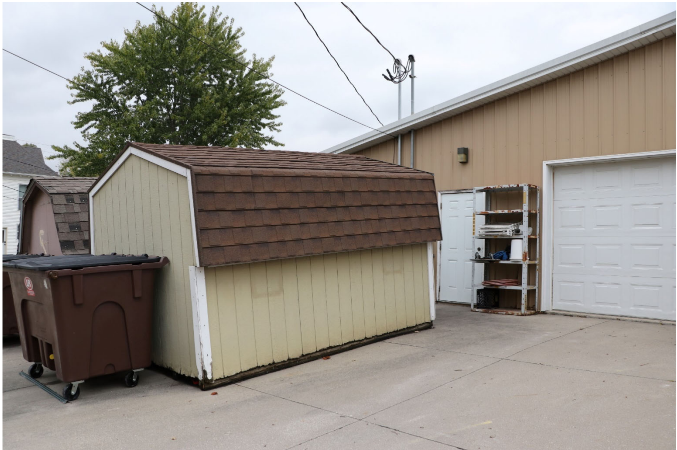
Photograph 44-02247-005. Sheds along west elevation, looking northeast (October 2023)
