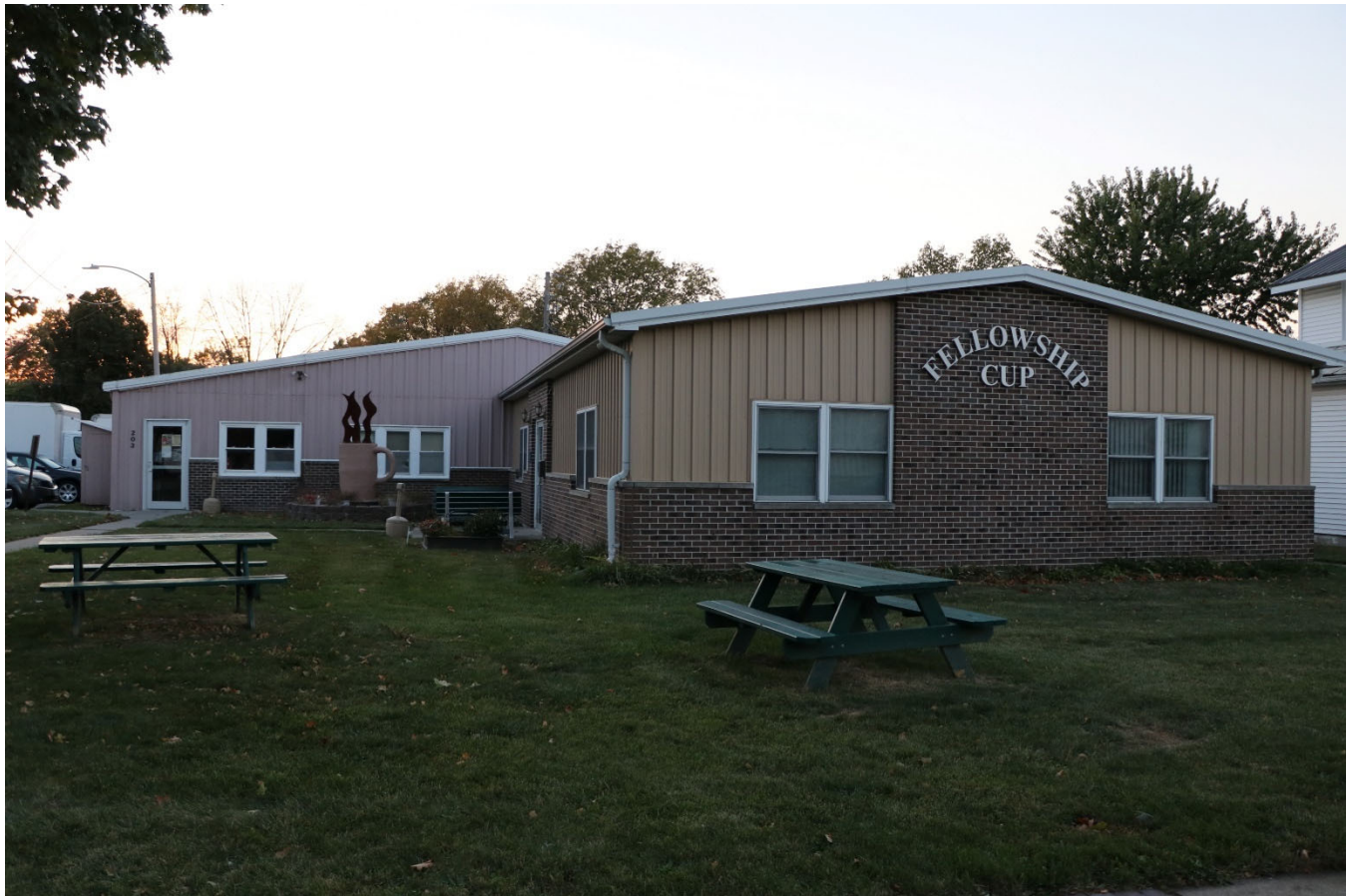
Photograph 44-02247-001. East elevation, looking west (October 2023)
