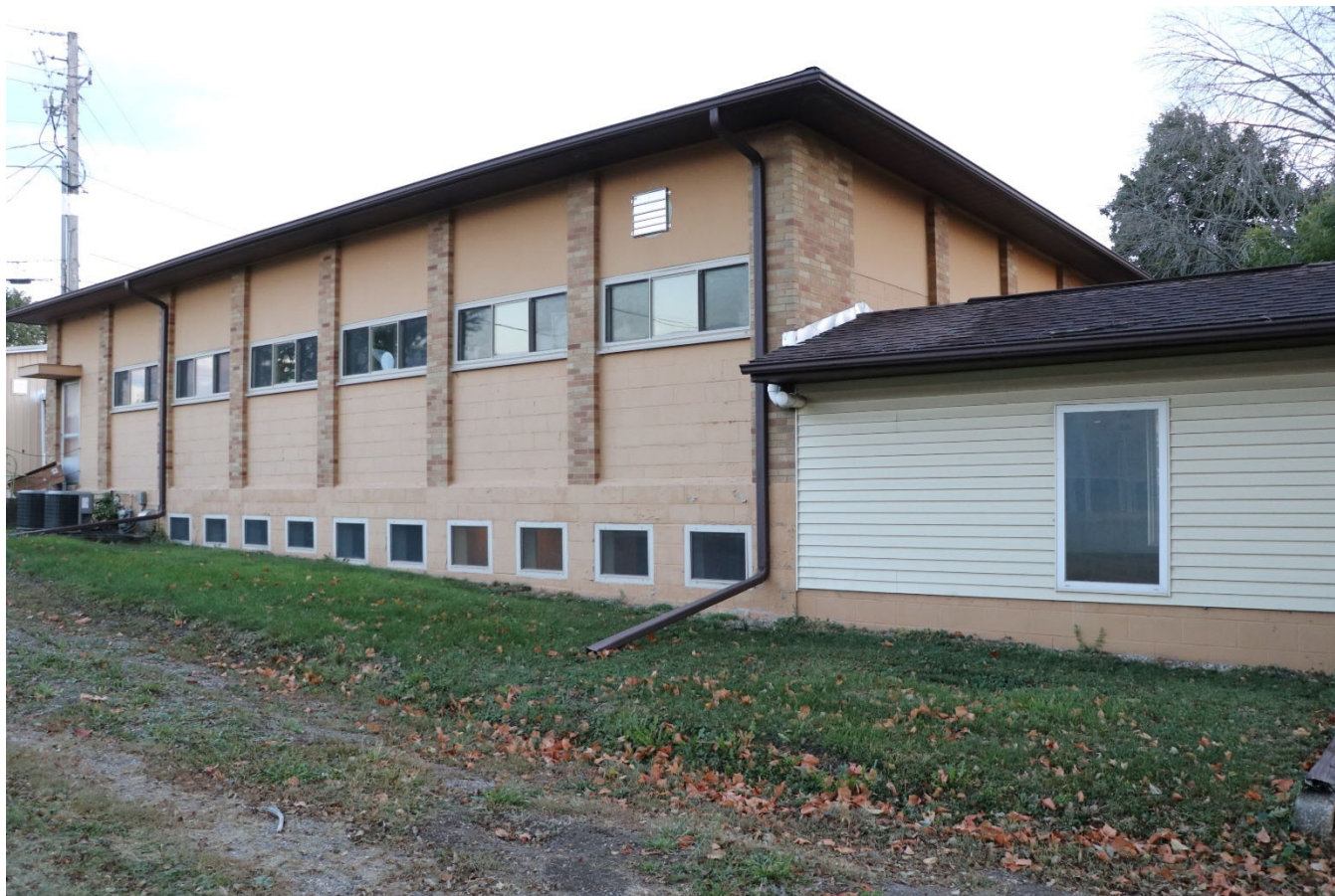
Photograph 44-02253-003. North elevation, looking southeast (October 2023)
