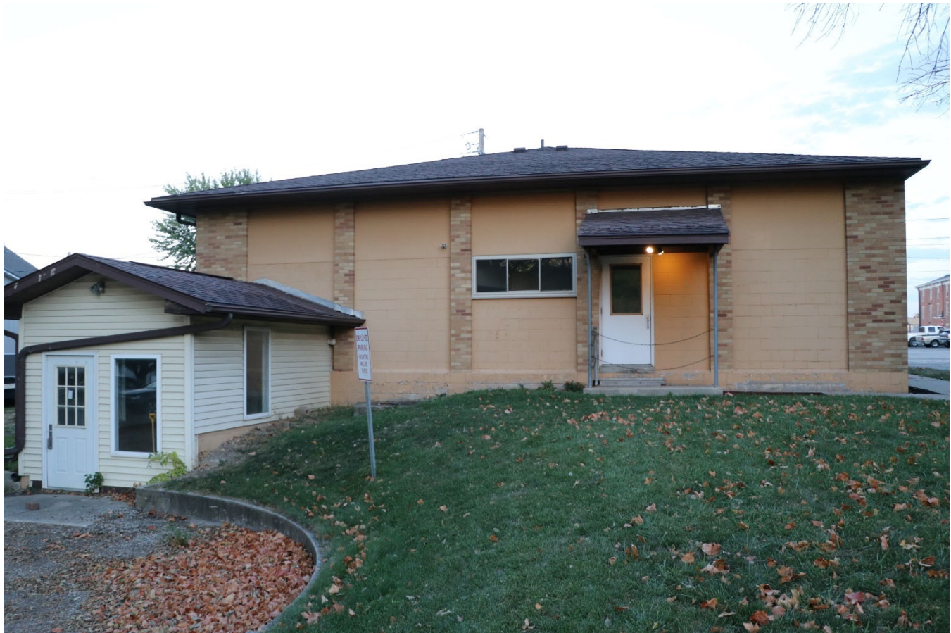
Photograph 44-02253-004. West elevation, looking east (October 2023)
