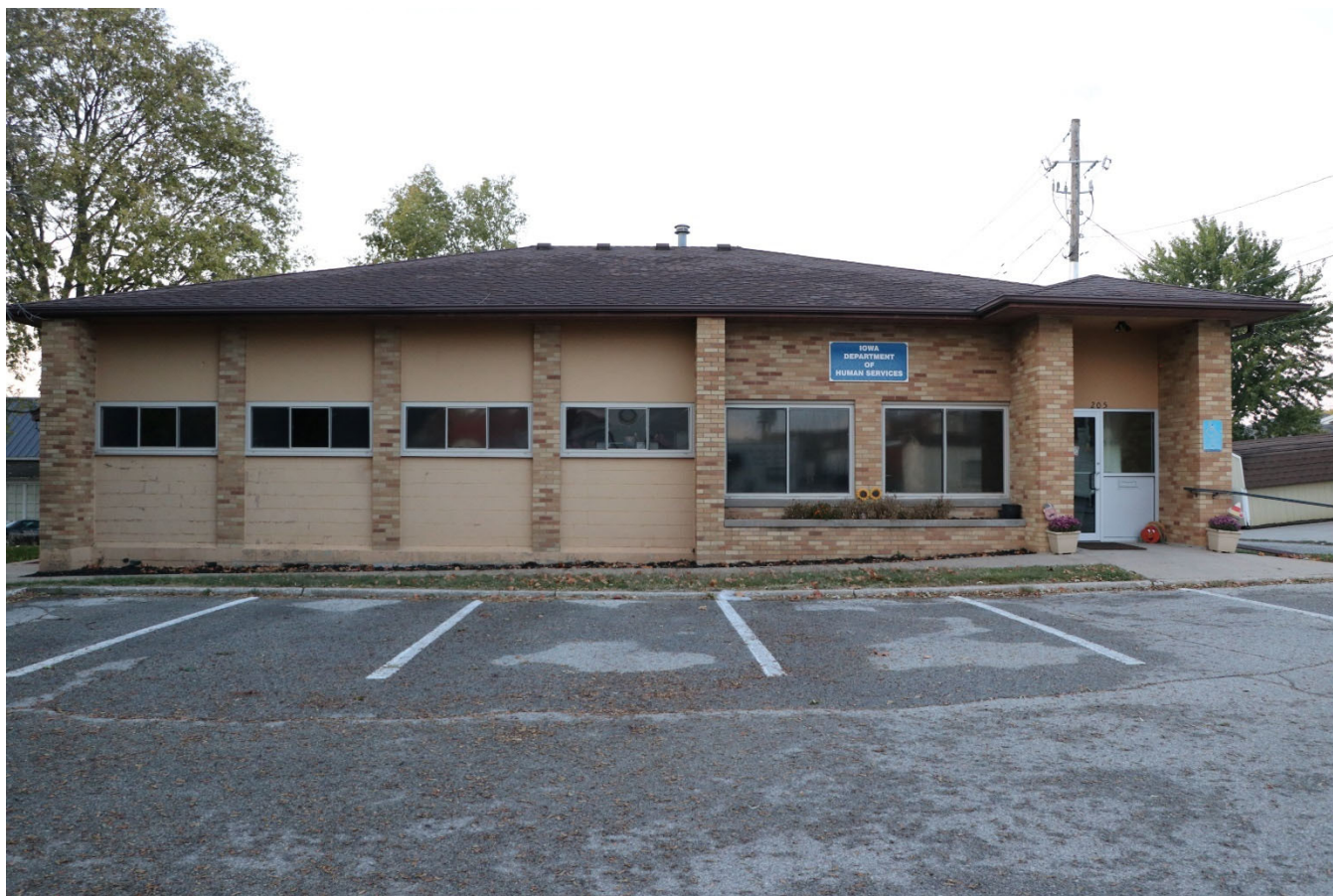
Photograph 44-02253-001. South elevation, looking north (October 2023)
