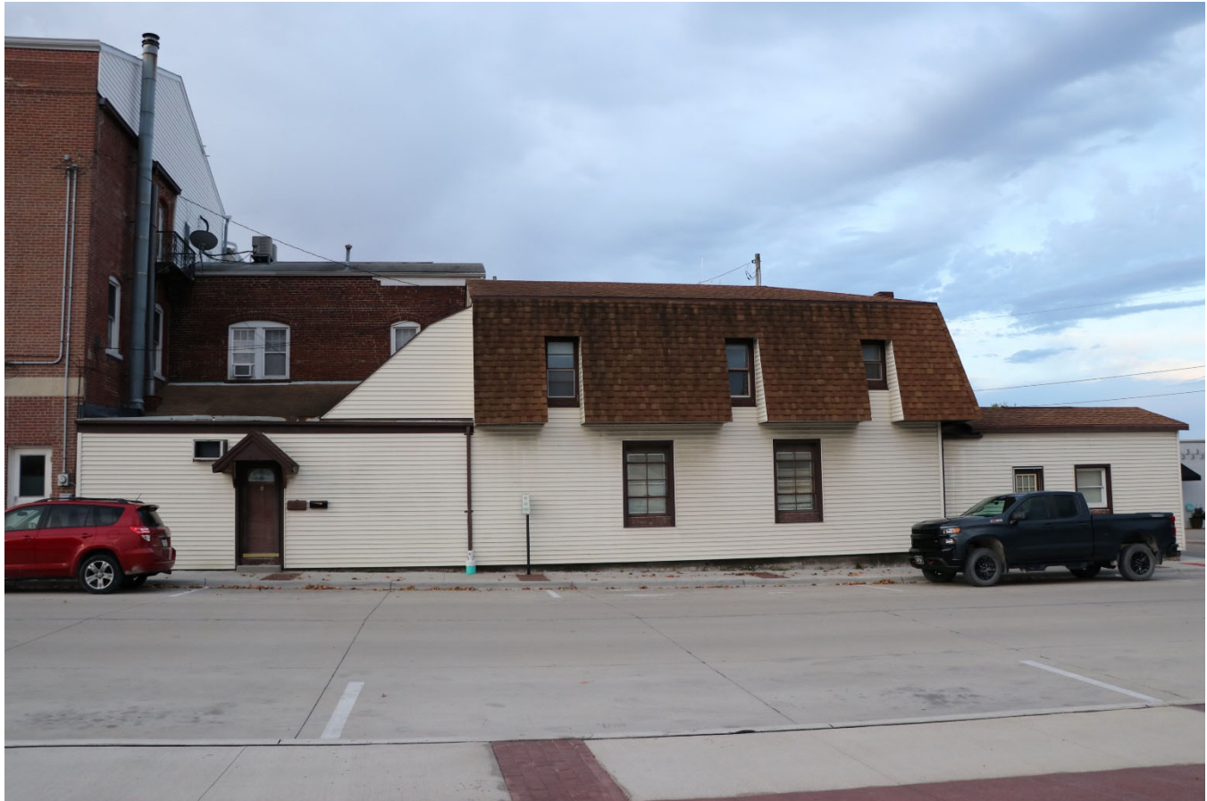
Photograph 44-00199-003. North elevation, looking south (October 2023)
