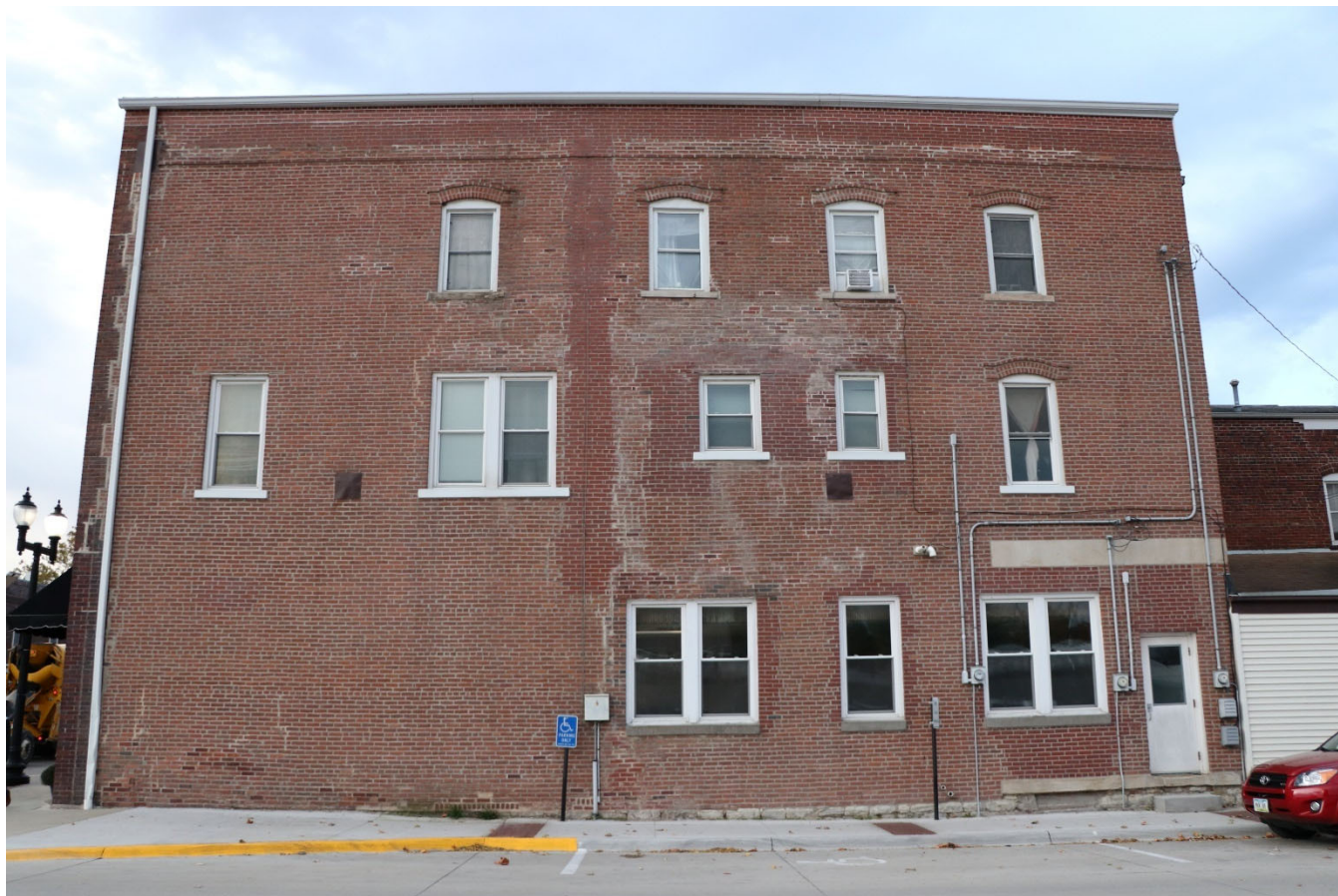
Photograph 44-00199-002. North elevation, looking south (October 2023)
