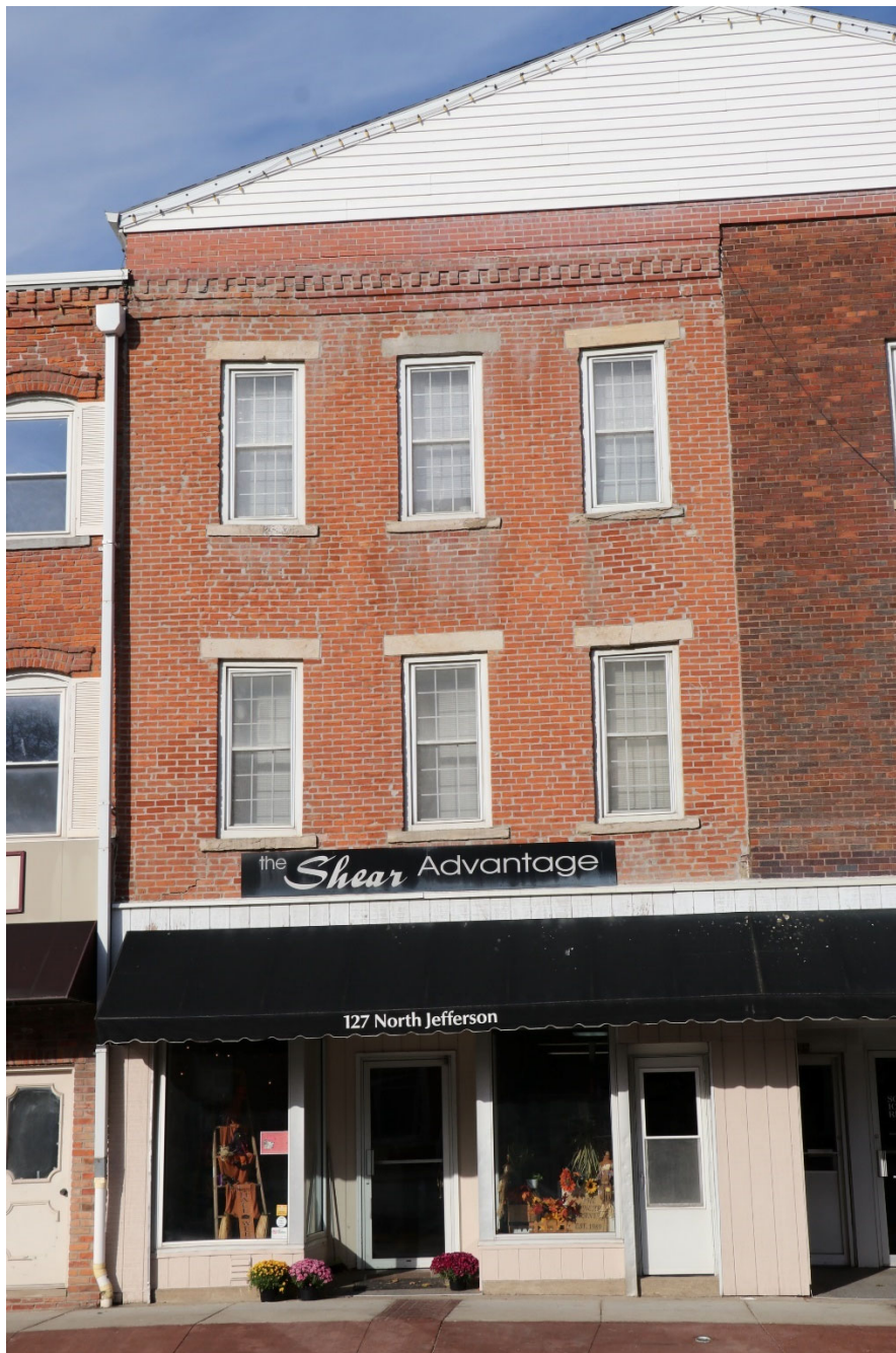
Photograph 44-02242-001. East elevation, looking west (October 2023)
