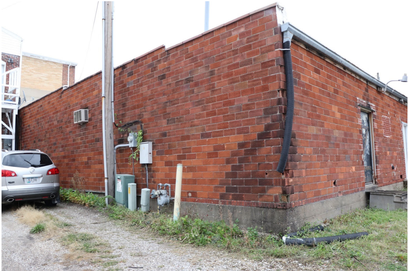
Photograph 44-00198-003. North and west elevations, looking southeast (October 2023)
