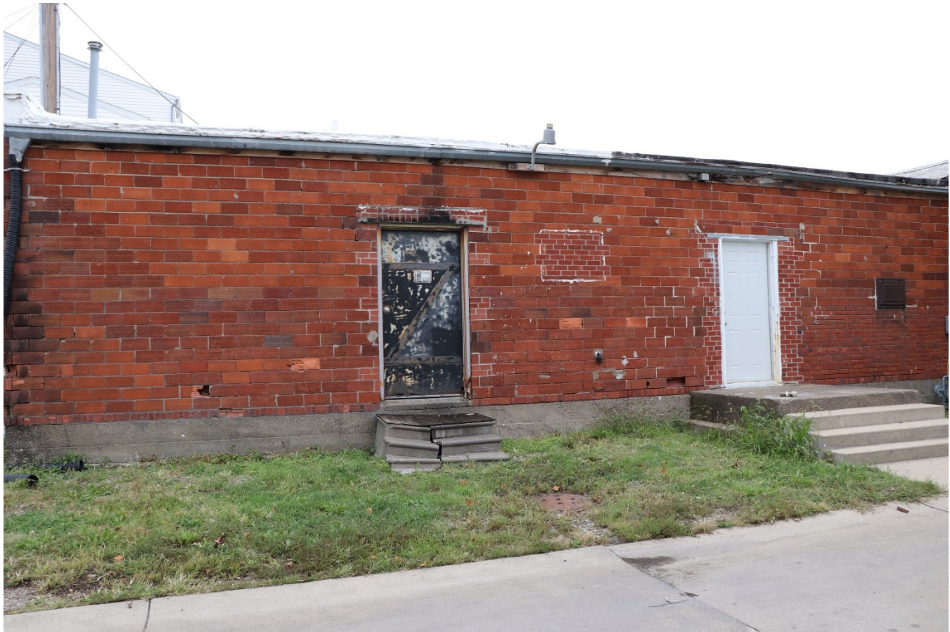
Photograph 44-00198-002. South elevations, looking north (October 2023)
