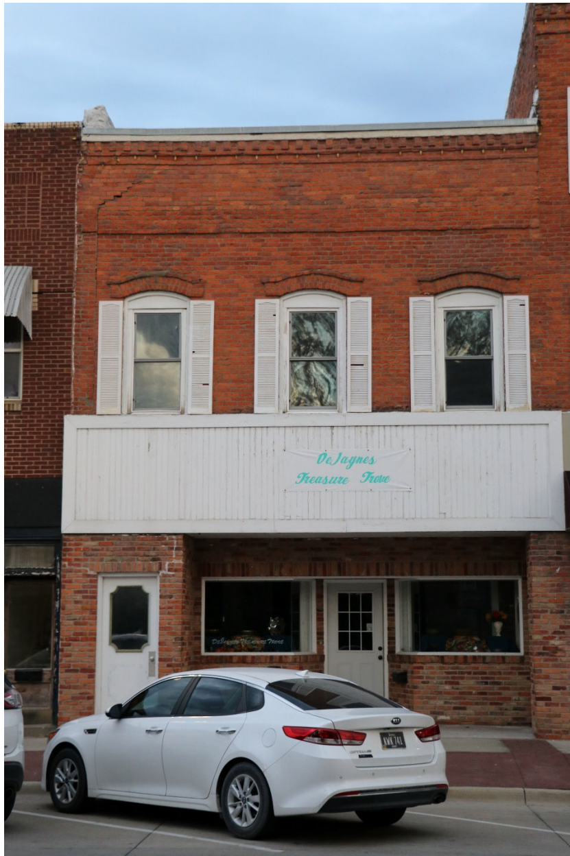
Photograph 44-00197-001. East elevation, looking west (October 2023)
