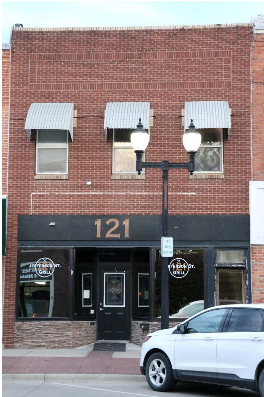
Photograph 44-00195-001. East elevation, looking west (October 2023)
