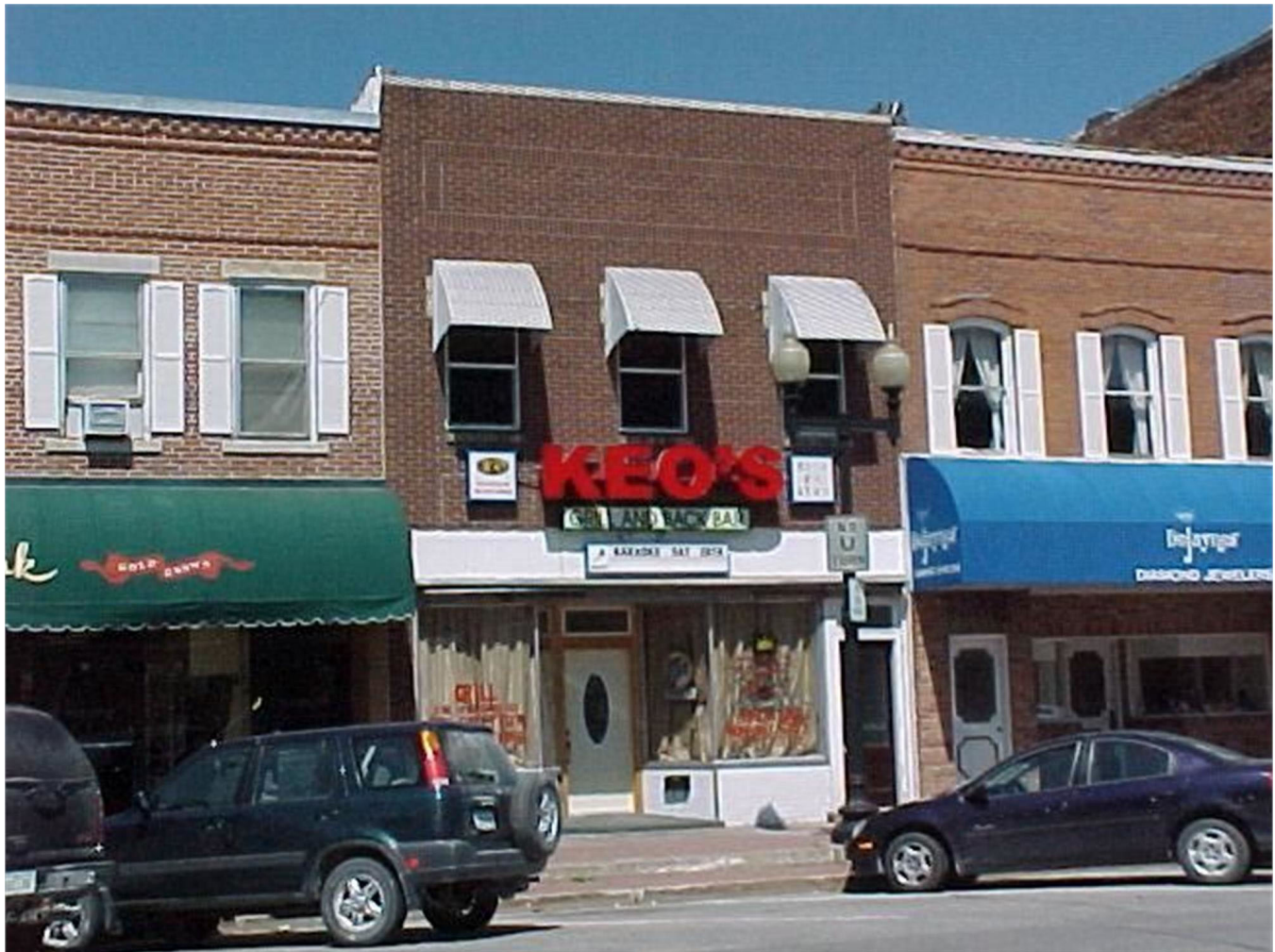
Building prior to 2006 storefront remodel
