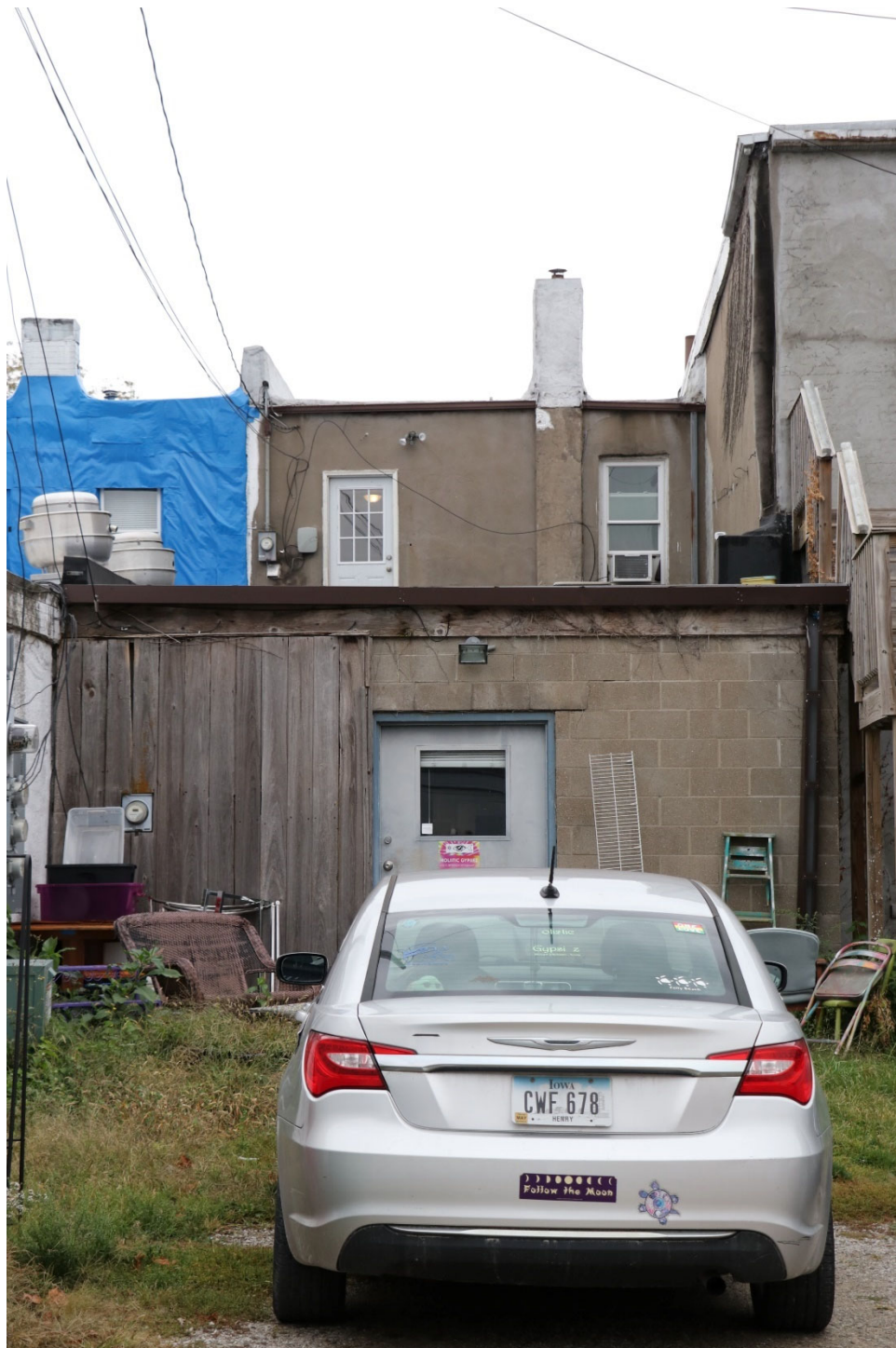
Photograph 44-00194-002. West elevation, looking east (October 2023)
