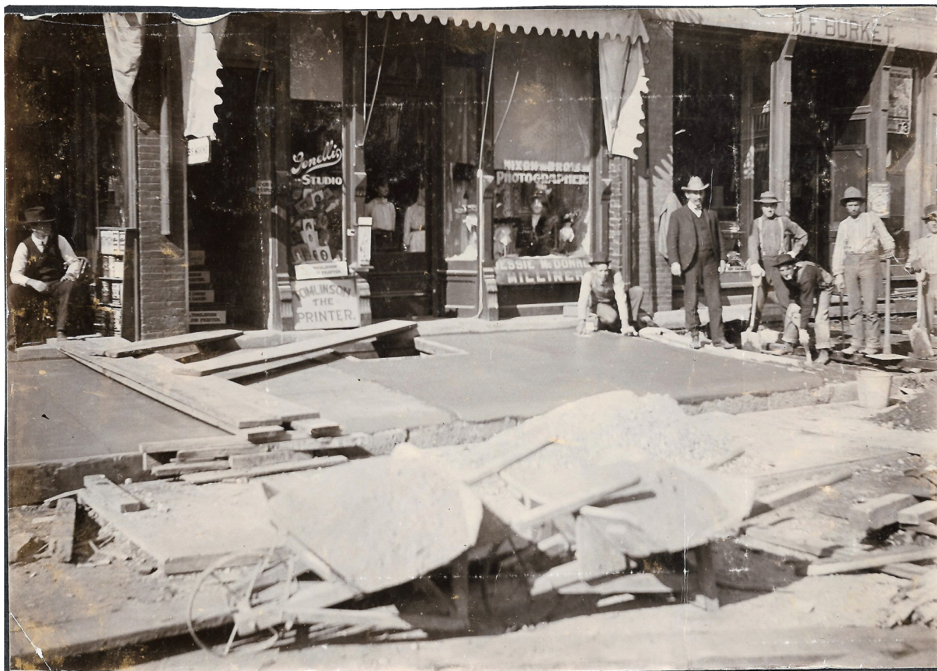
Partial south storefront, center stairs, and north storefront (Nixon Bros) around 1903 during sidewalk improvements (HCHT Facebook album)
