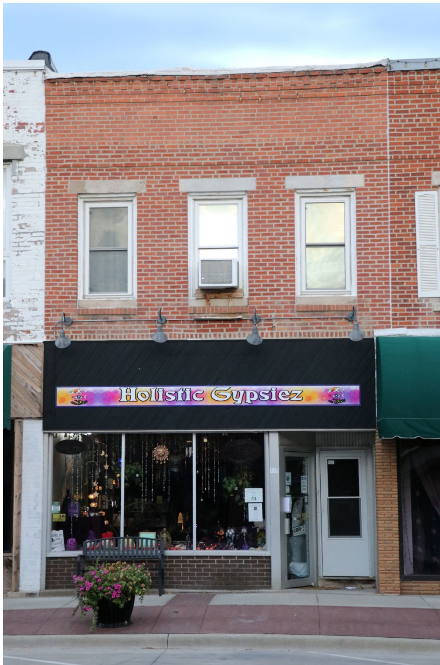
Photograph 44-00193-001. East elevation, looking west (October 2023)
