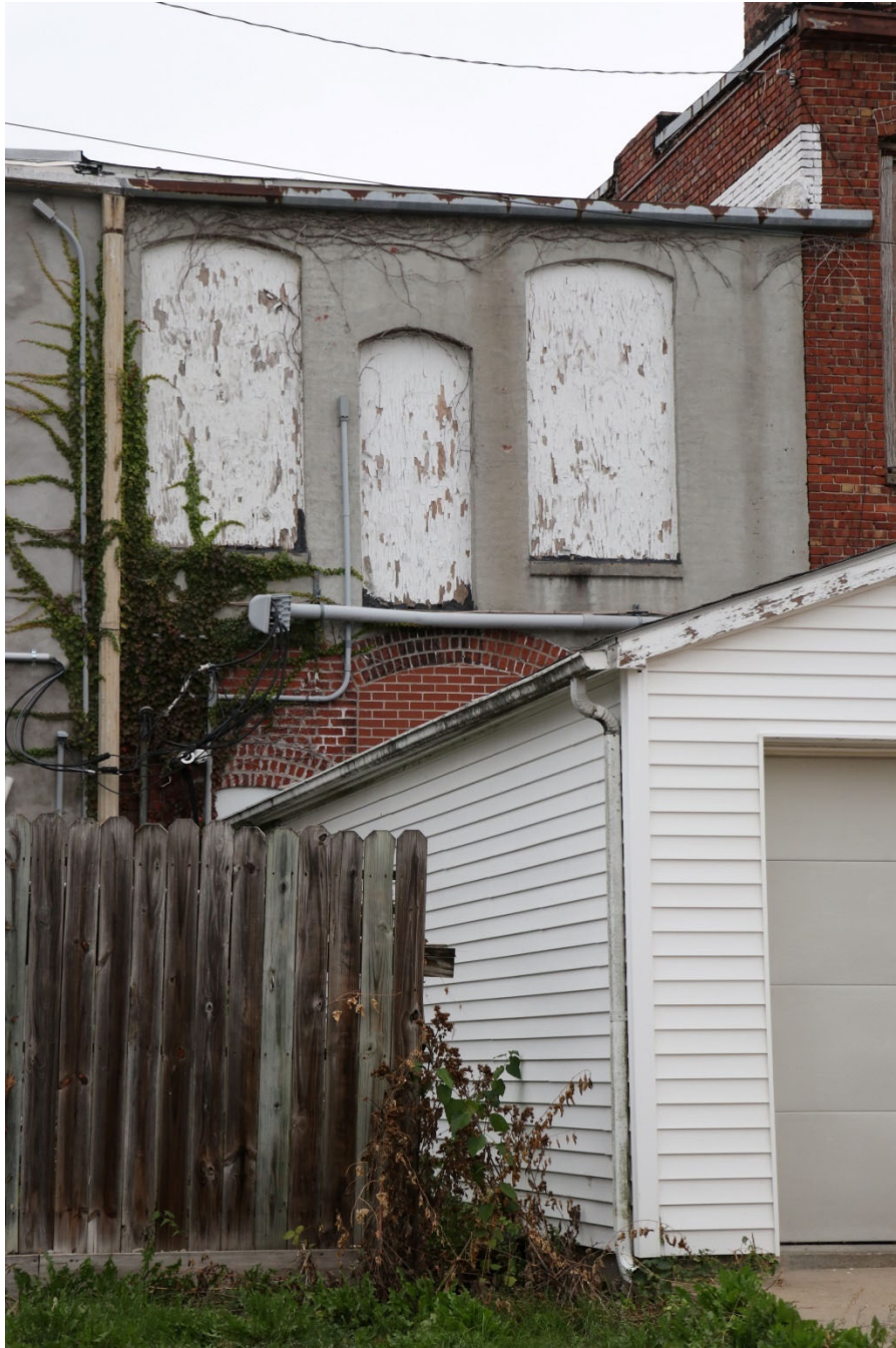
Photograph 44-00192-002. West elevation, looking southeast (October 2023)
