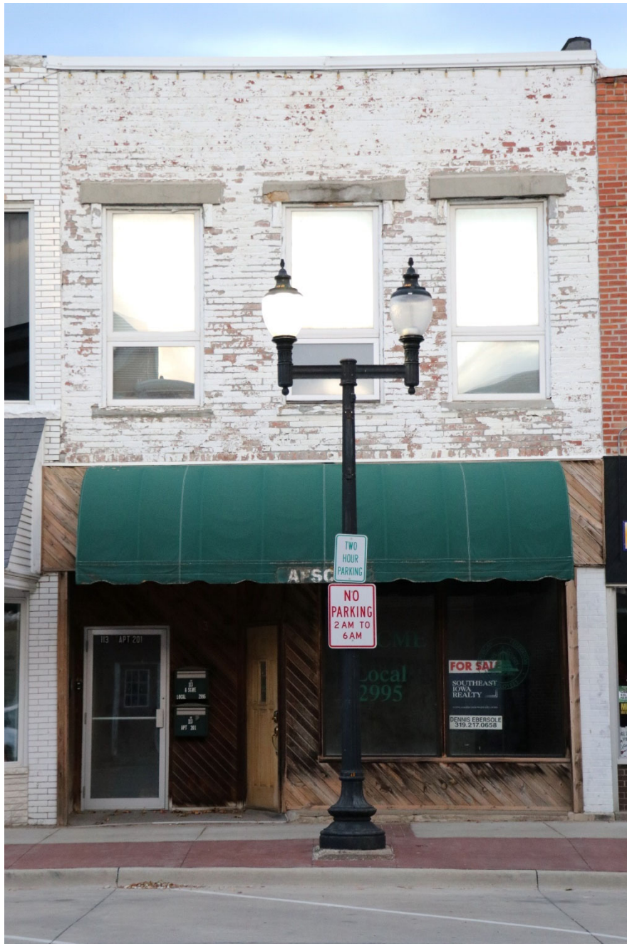
Photograph 44-00192-001. East elevation, looking west (October 2023)
