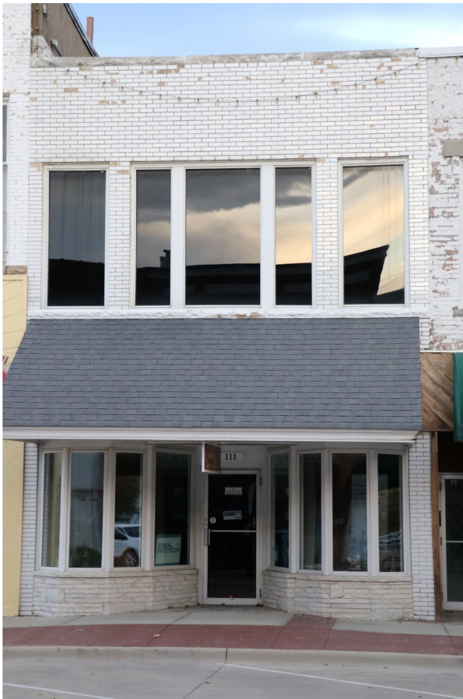
Photograph 44-00190-001. East elevation, looking west (October 2023)
