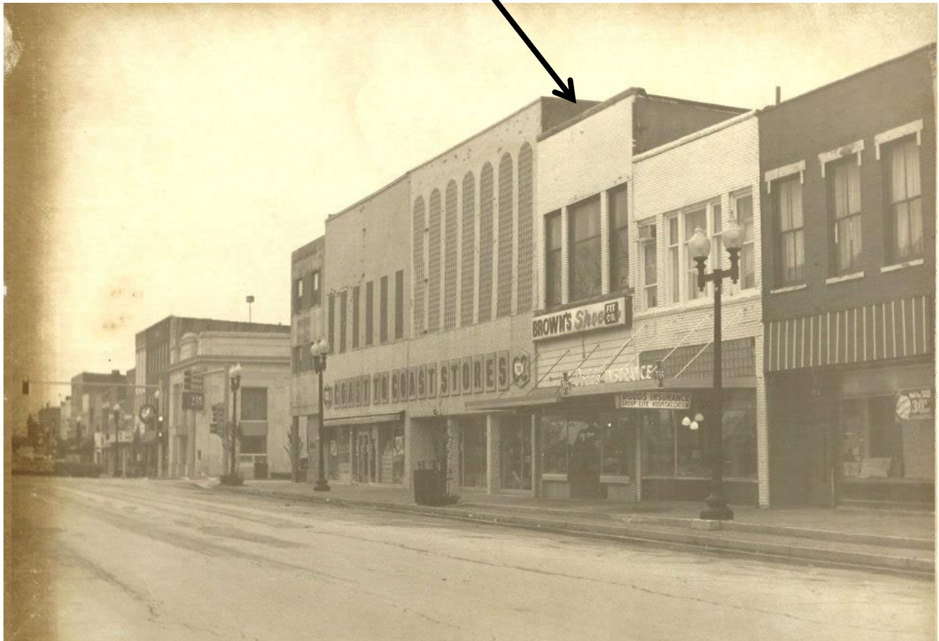
West side of 100 block of N Jefferson St in 1980s, looking southwest (HCHT Facebook album)
