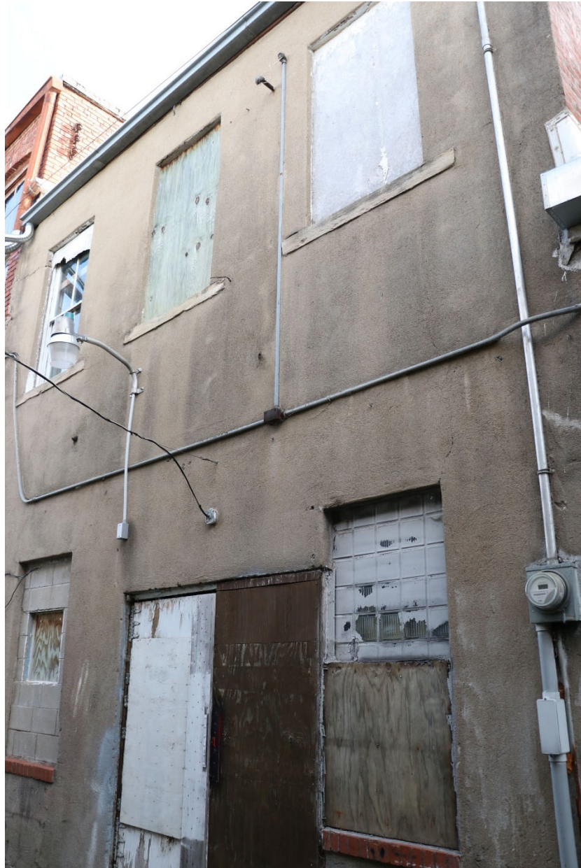
Photograph 44-00188-001. West elevation, looking northeast (October 2023)
