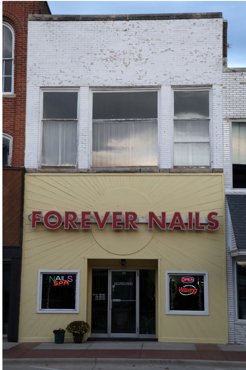
Photograph 44-00188-001. East elevation, looking west (October 2023)
