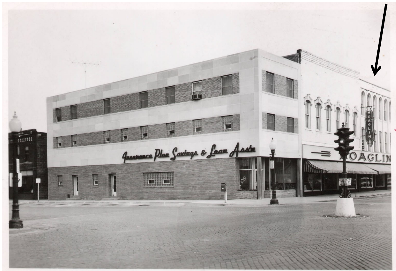
Building around 1955 (HCHT files)
