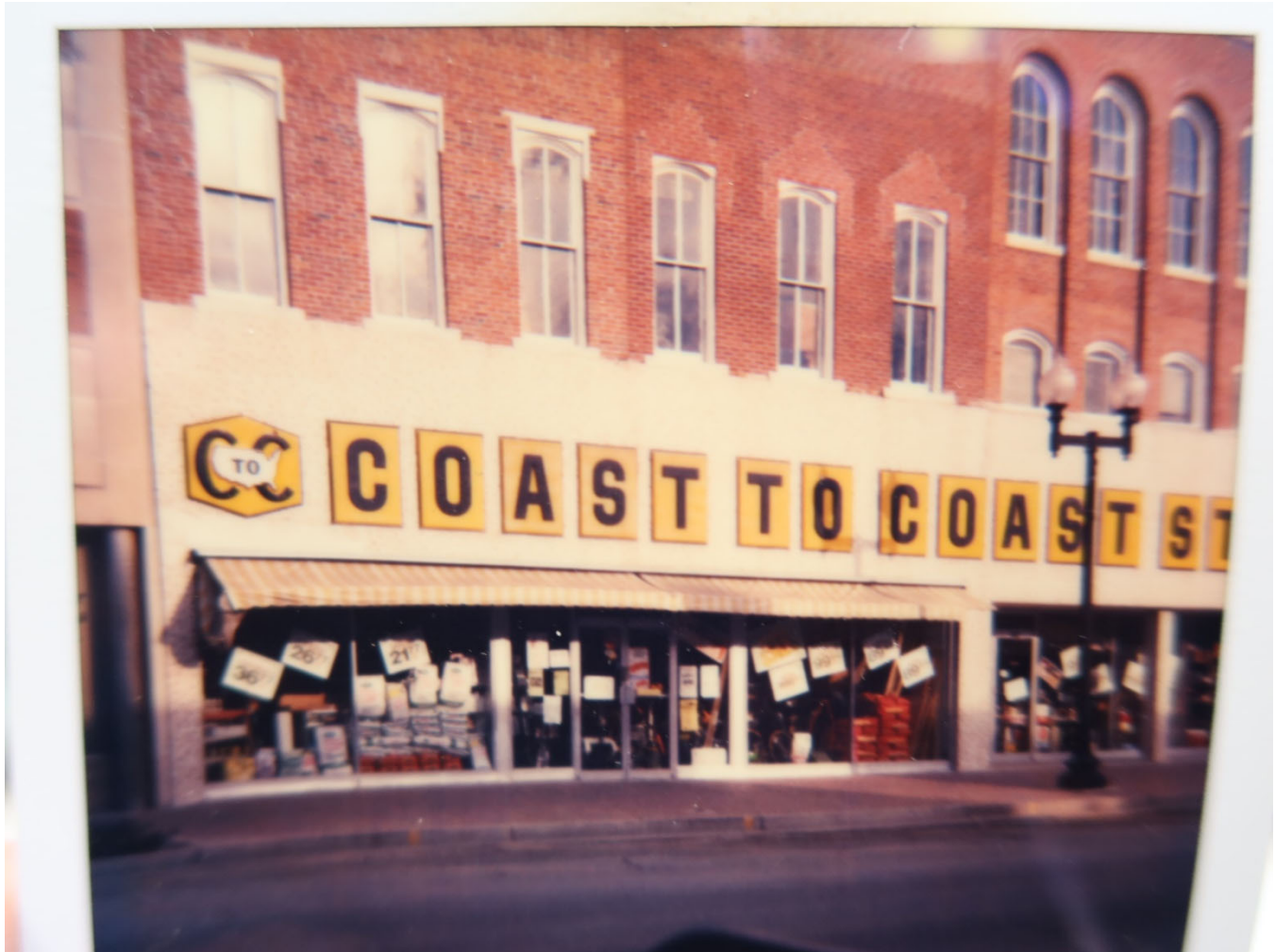
Building at right in June 1983 (City of Mt Pleasant building permits)
