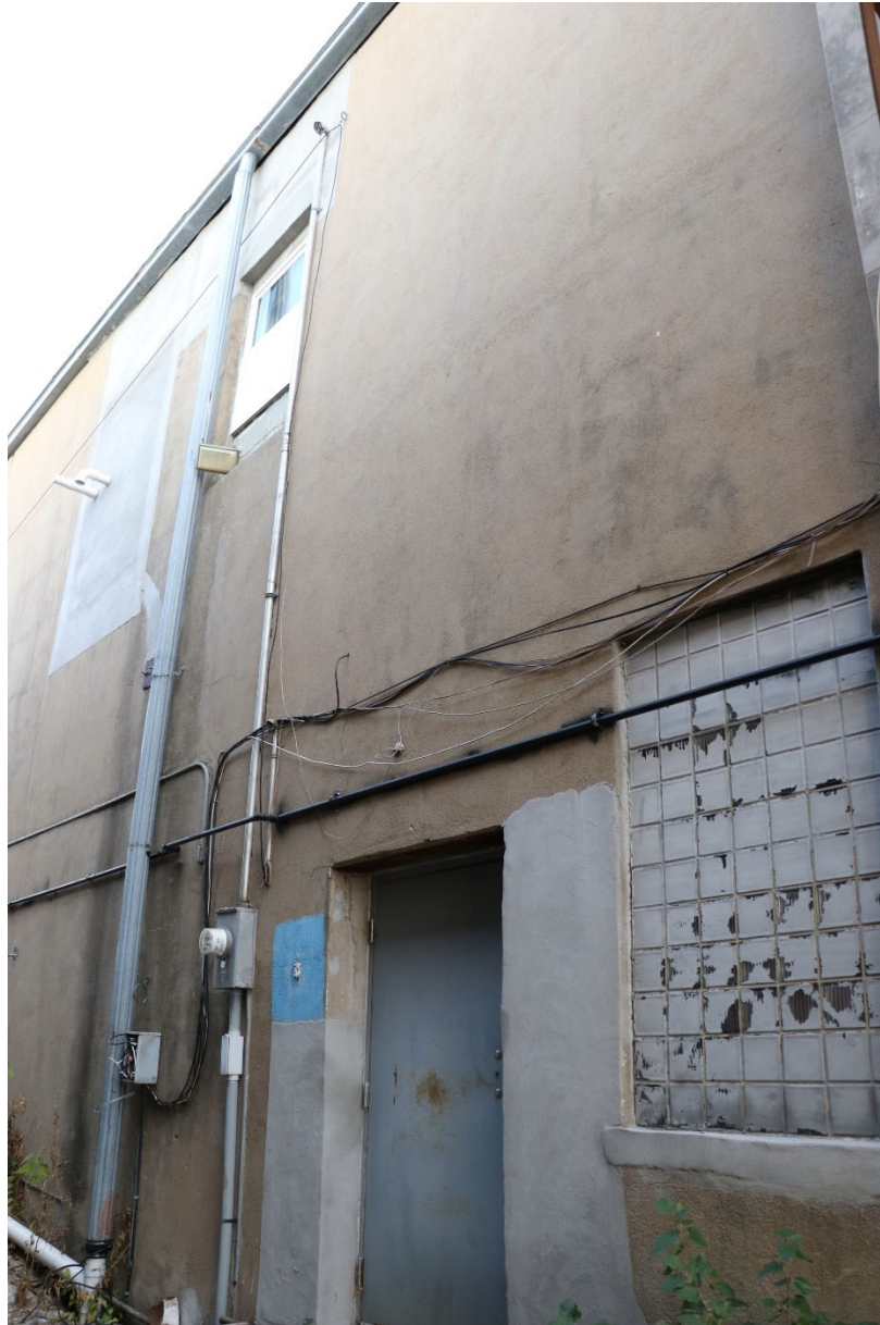
Photograph 44-00185-002. West elevation, looking northeast (October 2023)
