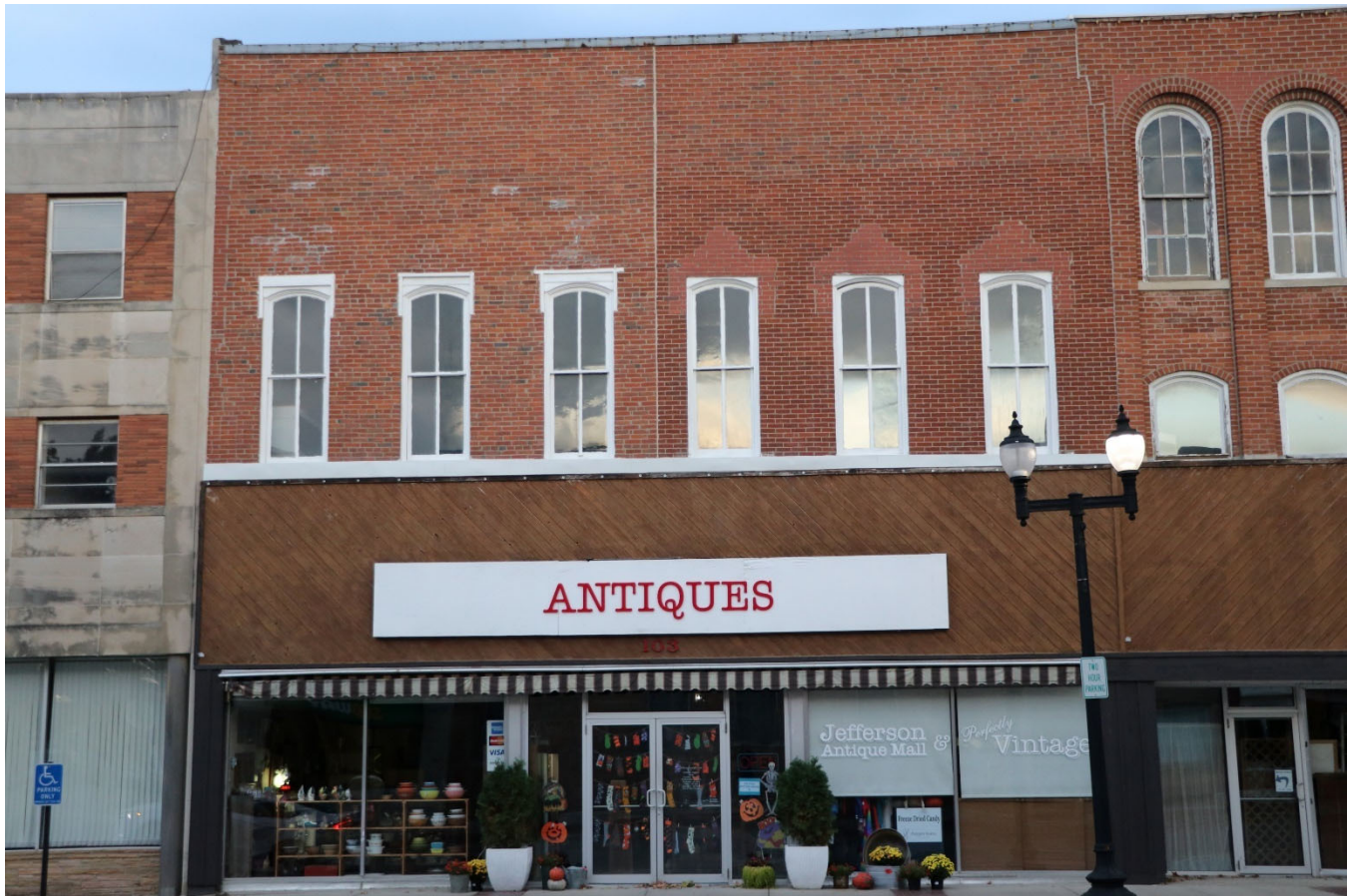
Photograph 44-00185-001. East elevation, looking west (October 2023)
