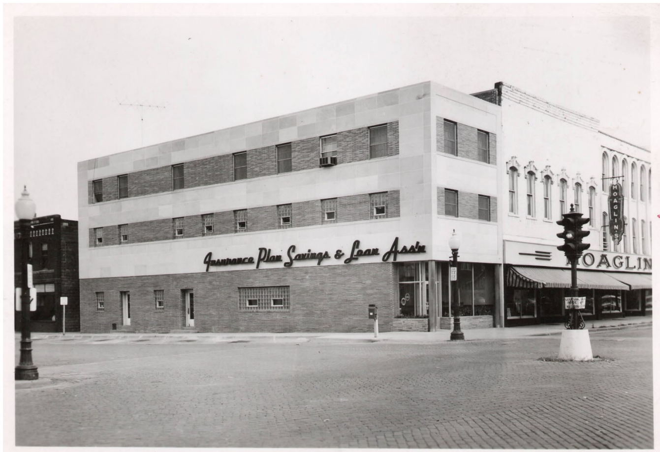
Building around 1955 (HCHT files)
