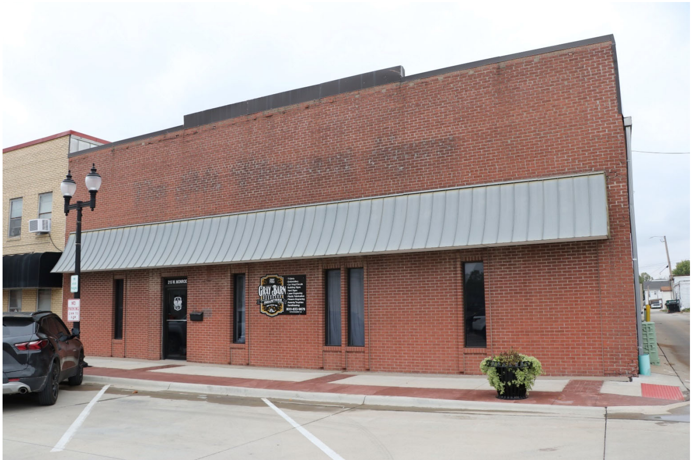
Photograph 44-00375-001. South elevation, looking northwest (October 2023)
