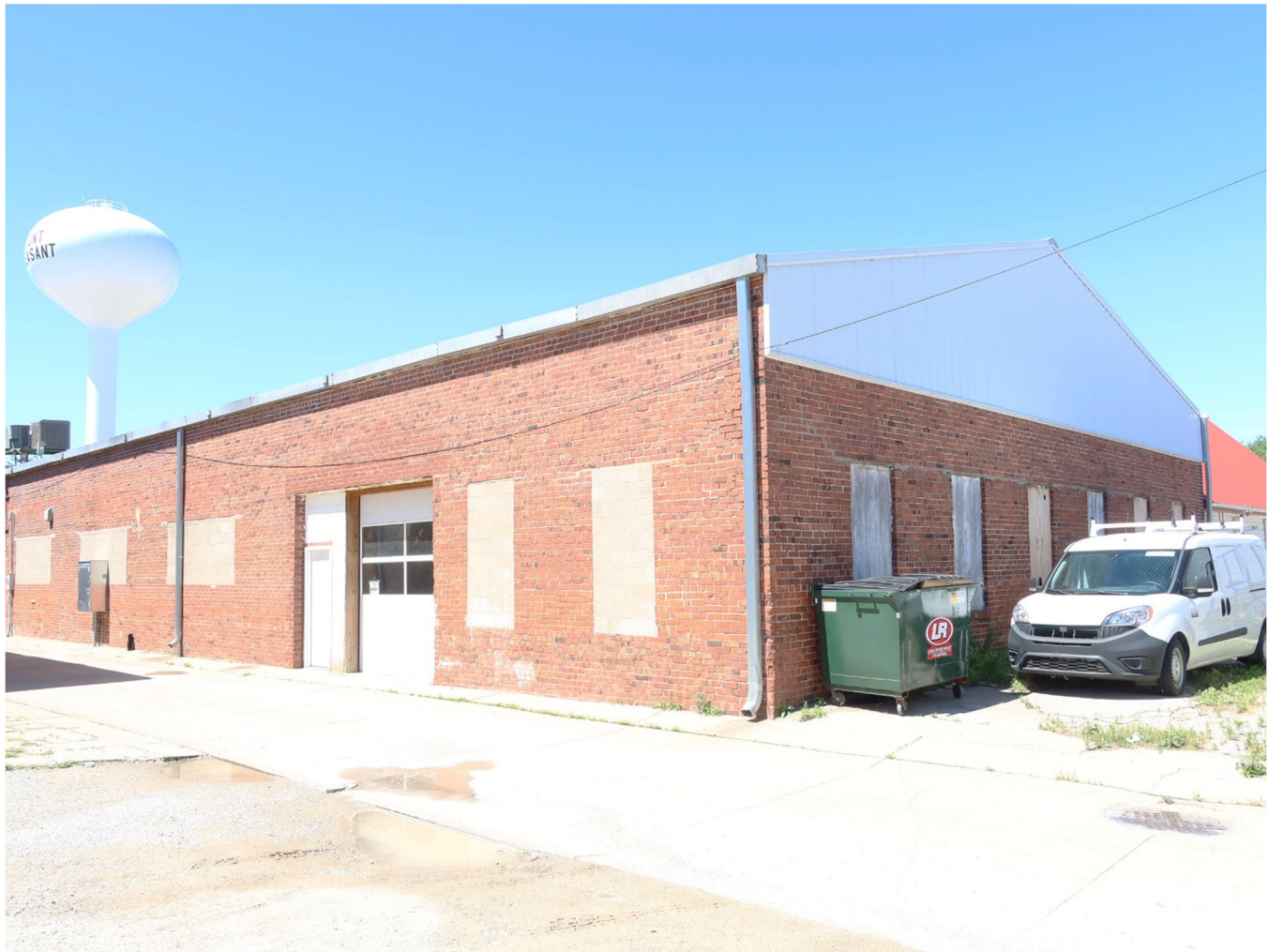
Photograph 44-00375-004. East and north (rear) elevations, looking southwest (June 2024)
