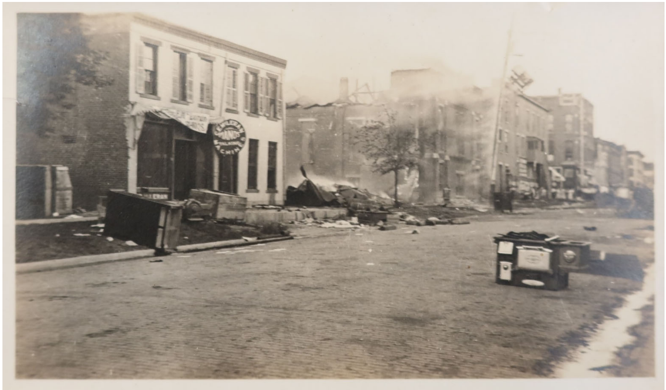
Damage on W. Monroe after June 17, 1914 fire, McLeran Building at left (HCHS binder, Mt Pleasant Public Library)
