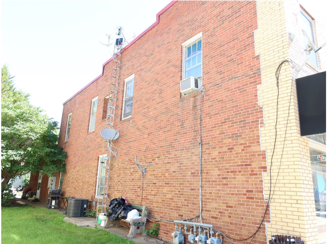
Photograph 44-00376-004. West elevation, looking northeast (June 2024)
