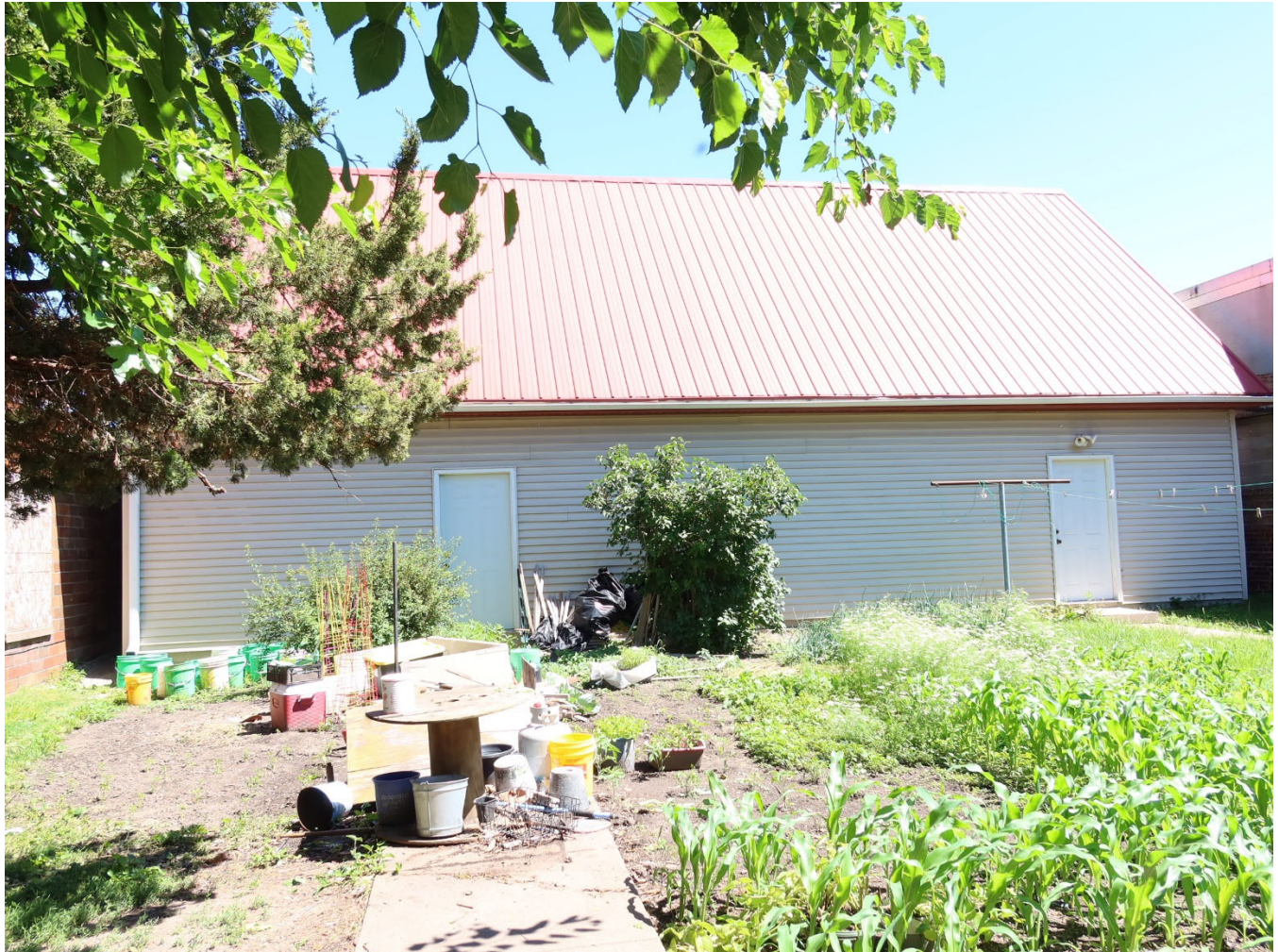
Photograph 44-00376-007. South elevation of garage, looking north (June 2024)
