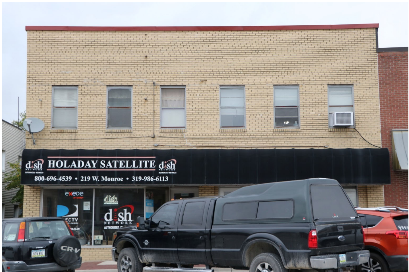
Photograph 44-00376-001. South elevation, looking north (October 2023)
