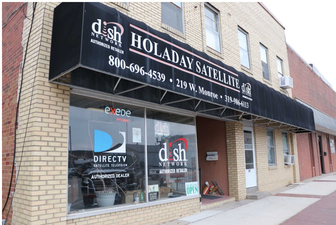
Photograph 44-00376-002. Storefront on south elevation, looking northeast (October 2023)
