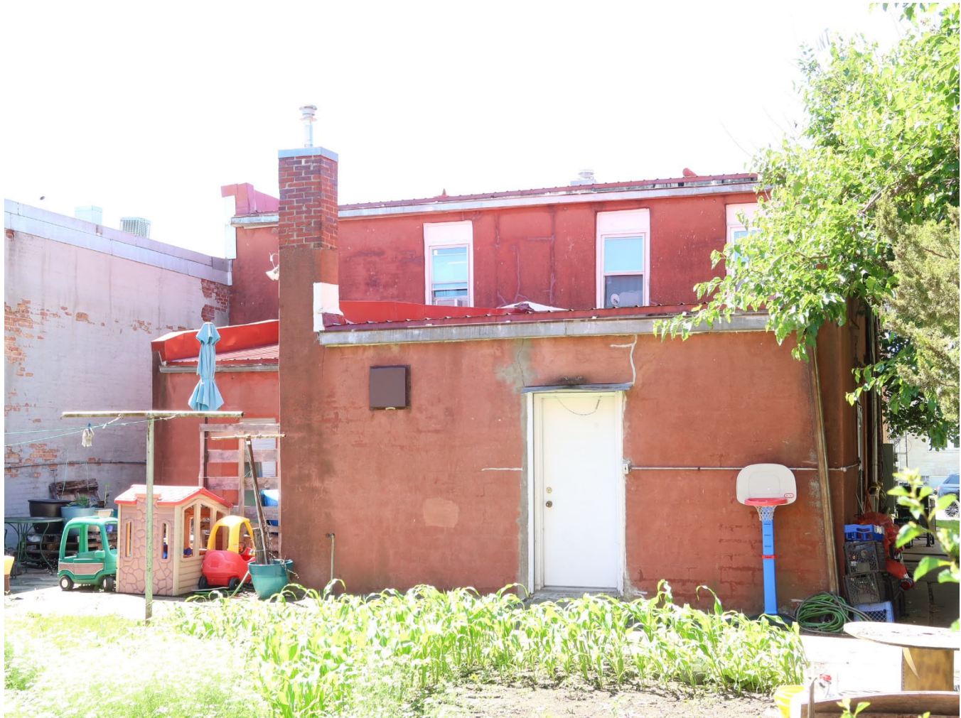
Photograph 44-00376-005. North elevation, looking south (June 2024)
