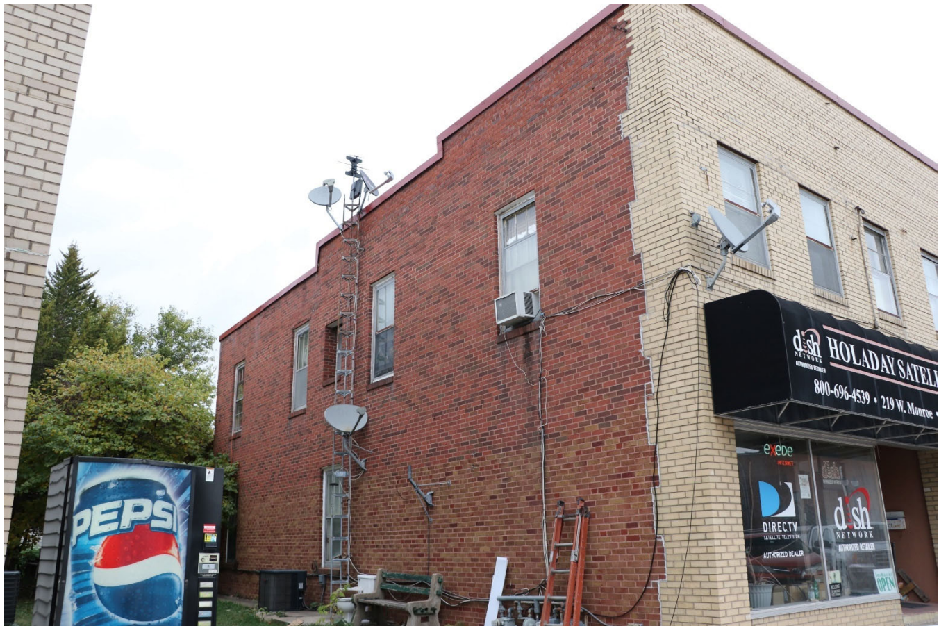
Photograph 44-00376-003. West elevation, looking northeast (October 2023)
