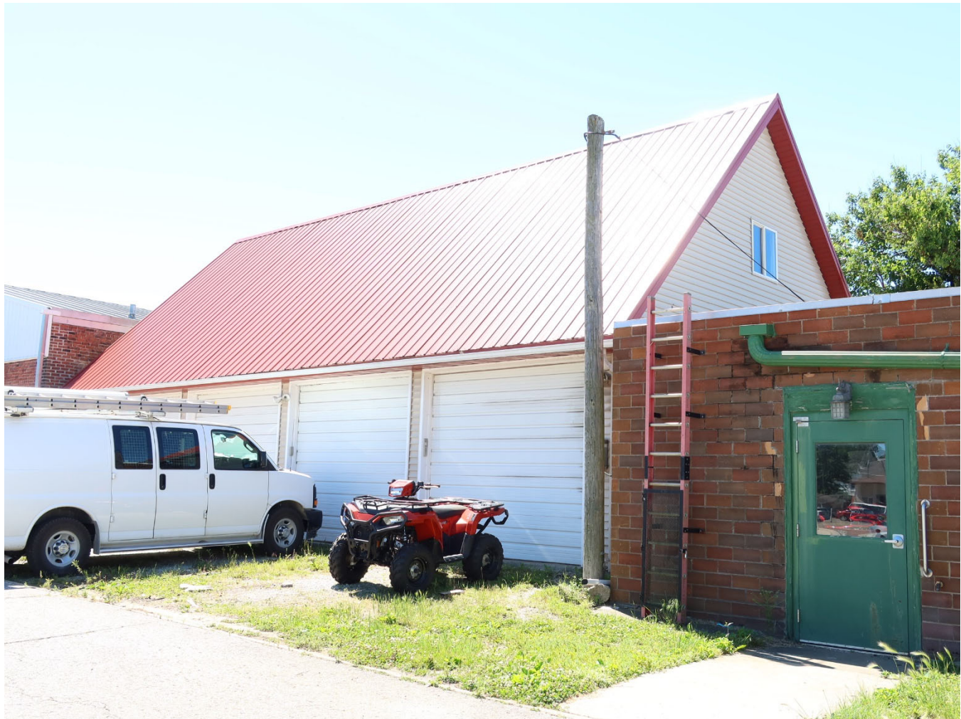
Photograph 44-00376-006. North and west elevations of garage, looking southeast (June 2024)
