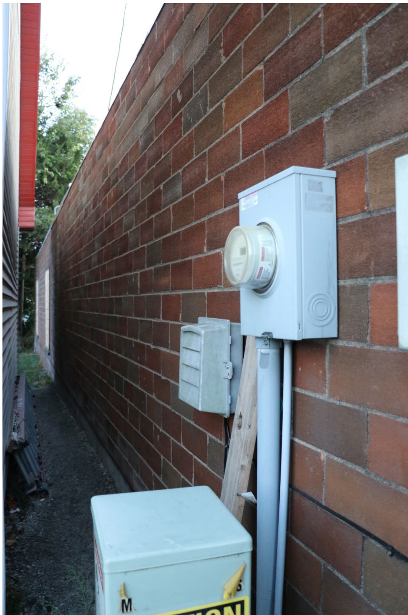
Photograph 44-02239-005. East elevation, looking southwest (October 2023)
