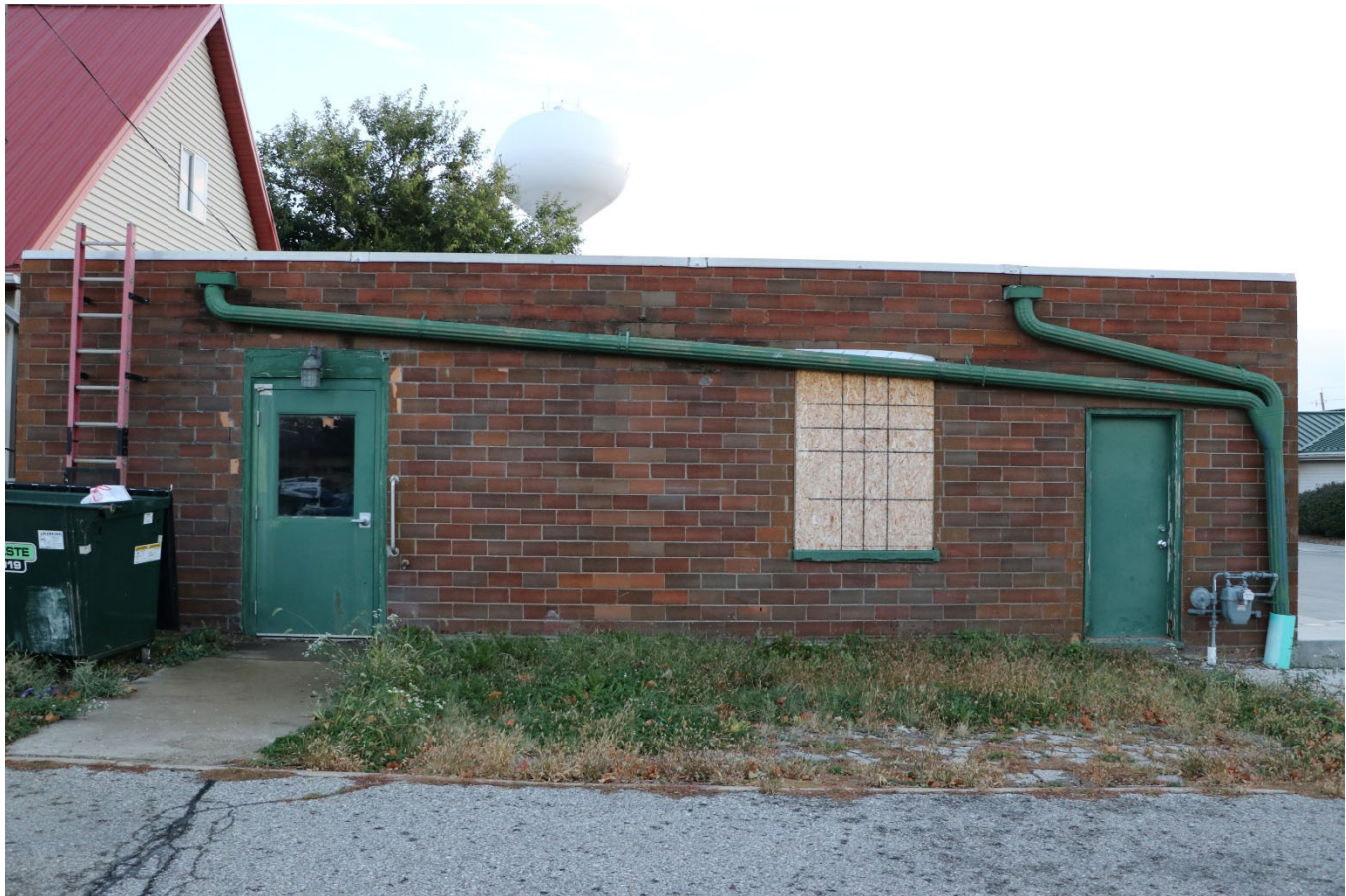
Photograph 44-02239-002. North elevation, looking south (October 2023)
