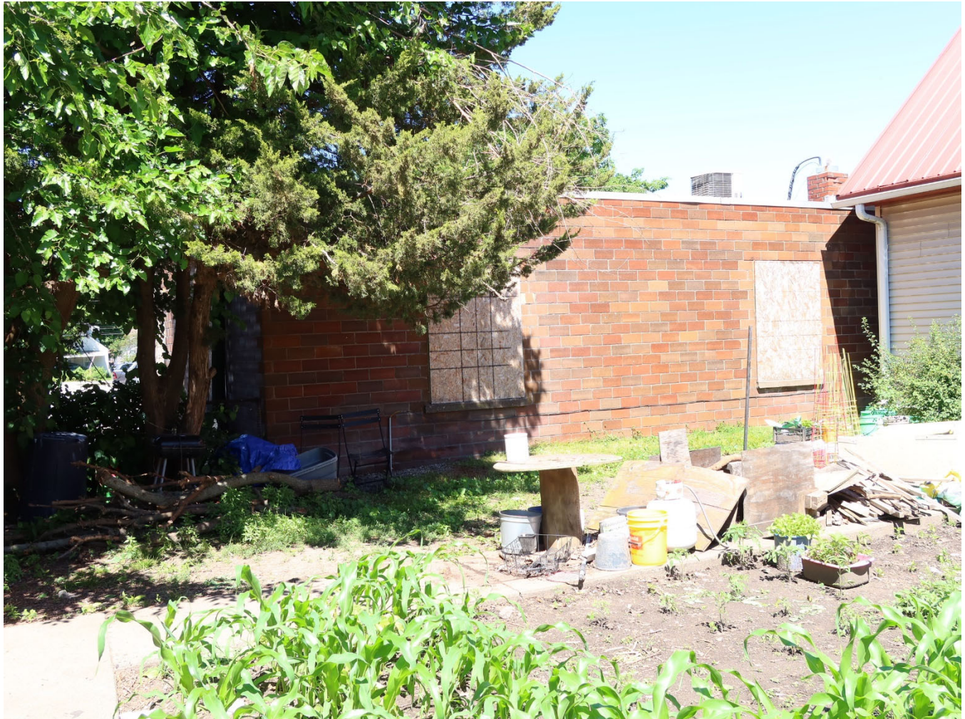
Photograph 44-02239-004. East elevation, looking west (June 2024)
