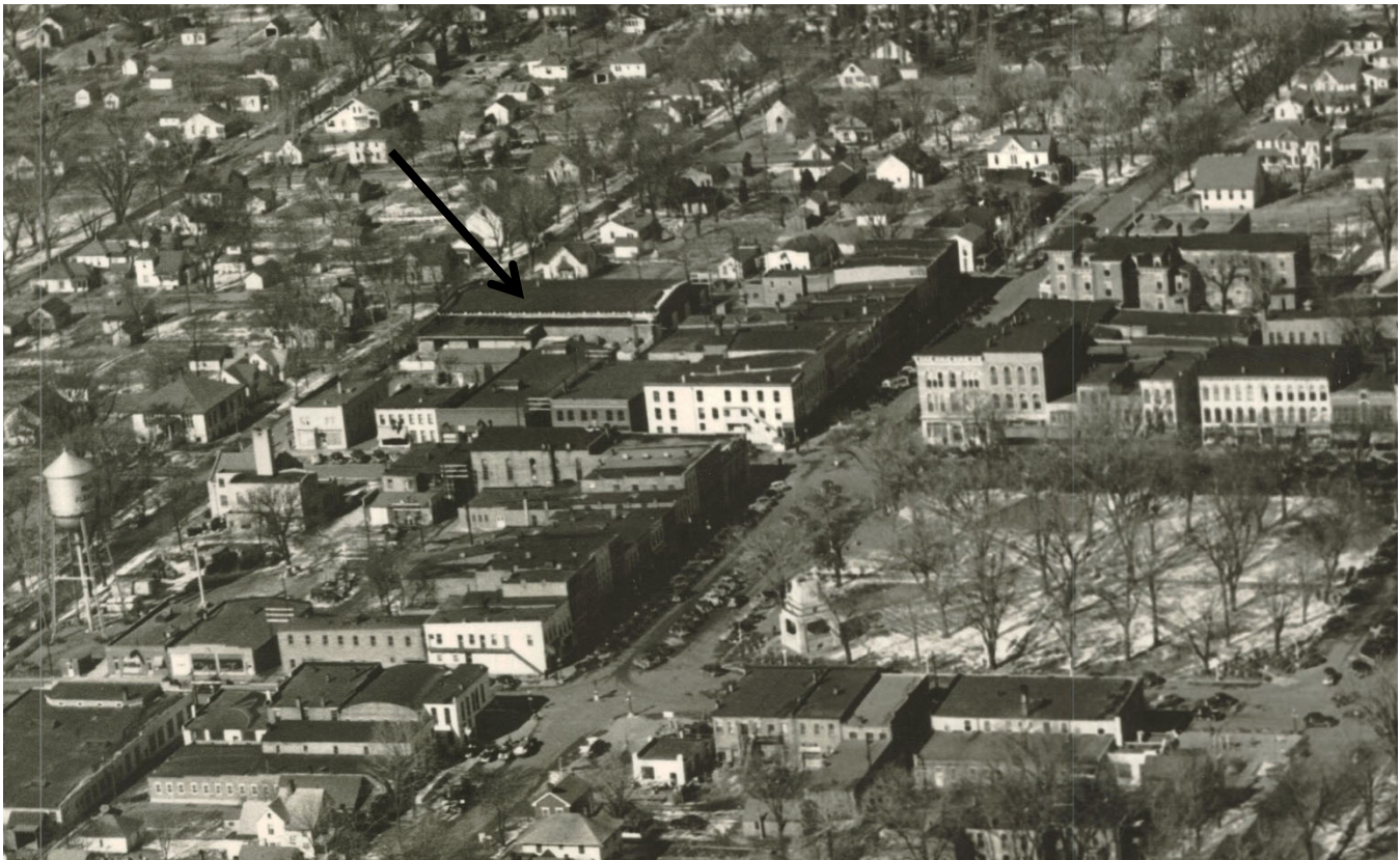
Earlier lumber company buildings on site
