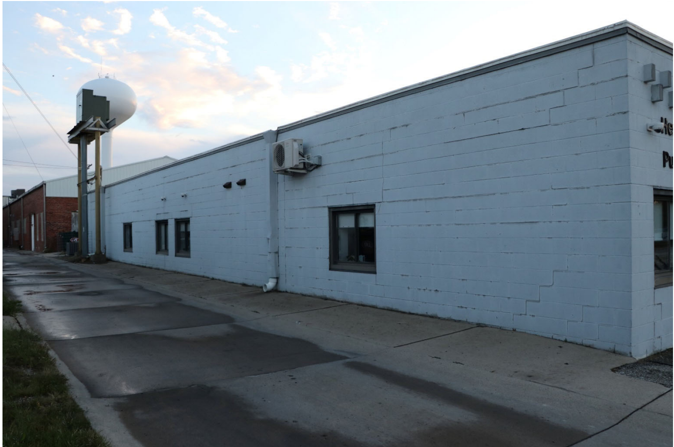
Photograph 44-00180-003. East elevation, looking southwest (October 2023)
