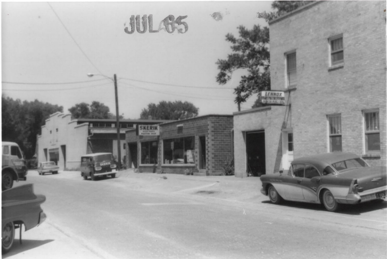
Earlier lumber company building at north end of 100 block of N. Jackson St in July 1965 (HCHT collection)
