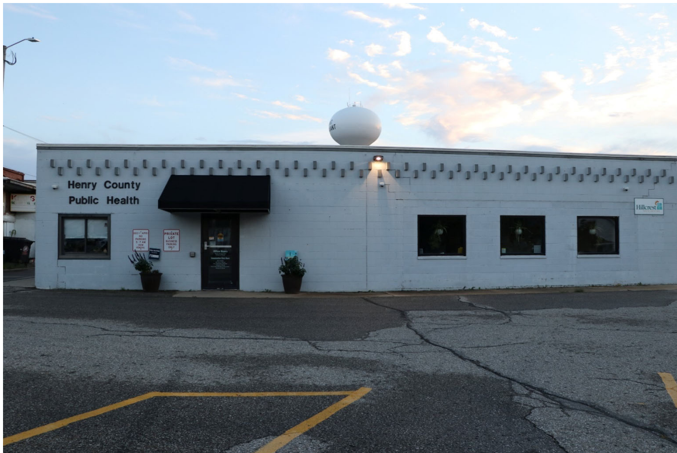
Photograph 44-00180-002. North elevation, looking south (October 2023)
