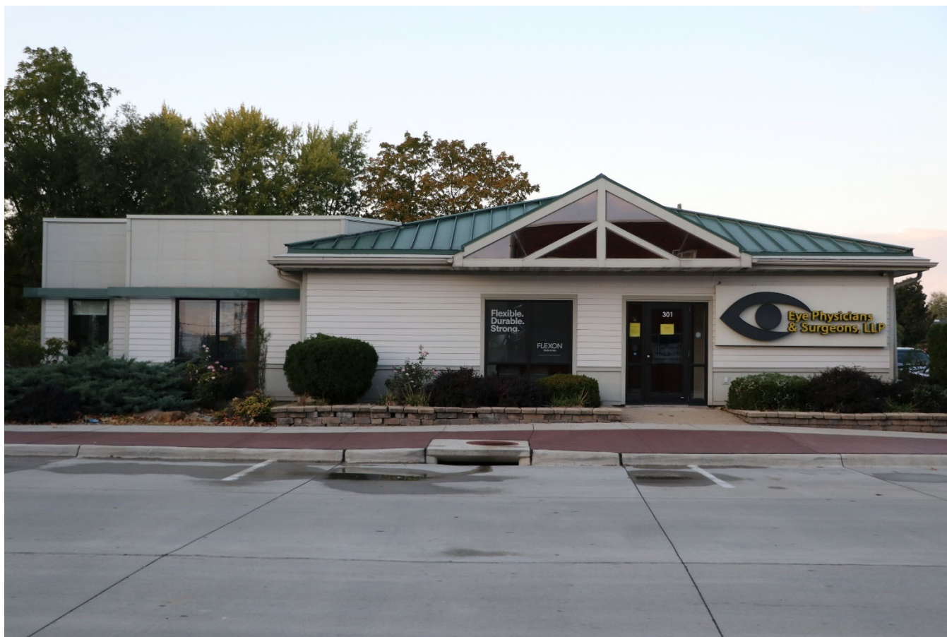
Photograph 44-02265-001. South elevation, looking north (October 2023)
