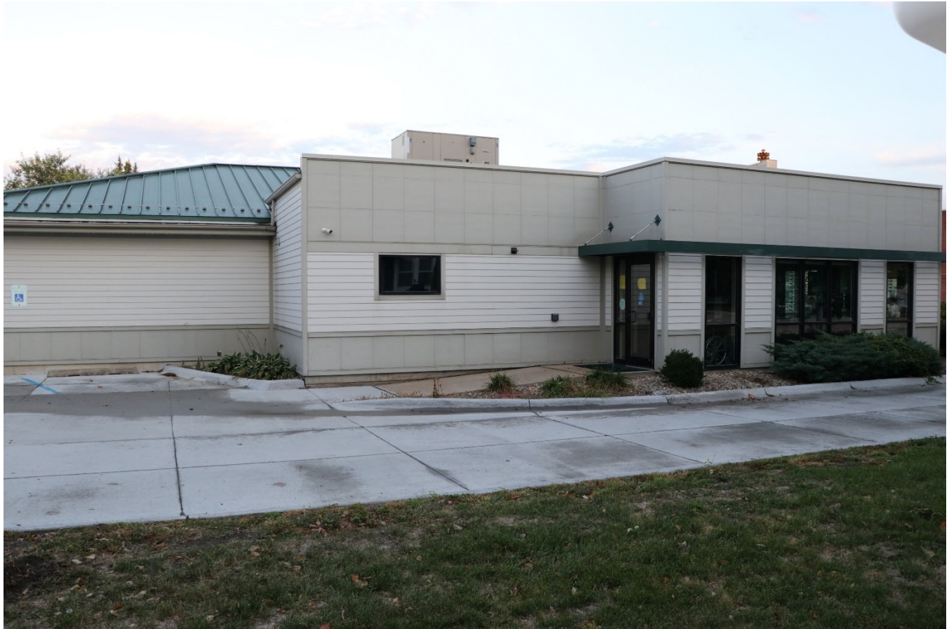
Photograph 44-02265-003. West elevation, looking east (October 2023)
