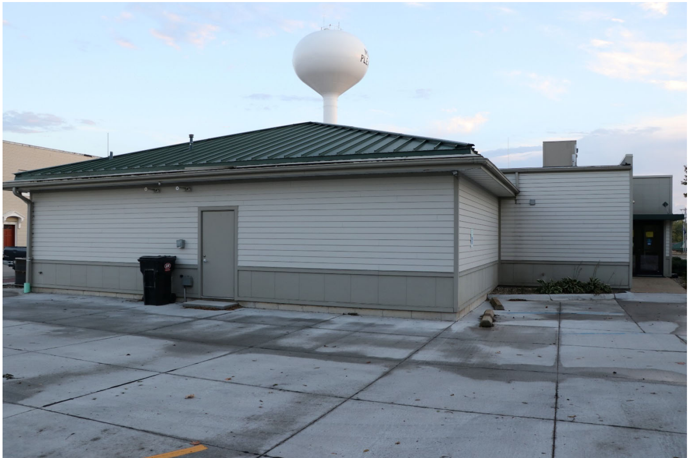
Photograph 44-02265-004. North elevation, looking south (October 2023)
