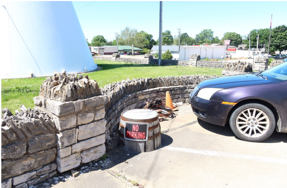
Photograph 44-00377-017. Stone wall, looking southwest (June 2024)
