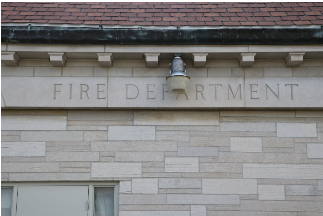
Photograph 44-00377-005. Detail on east section of north elevation of City Hall, looking south (October 2023)
