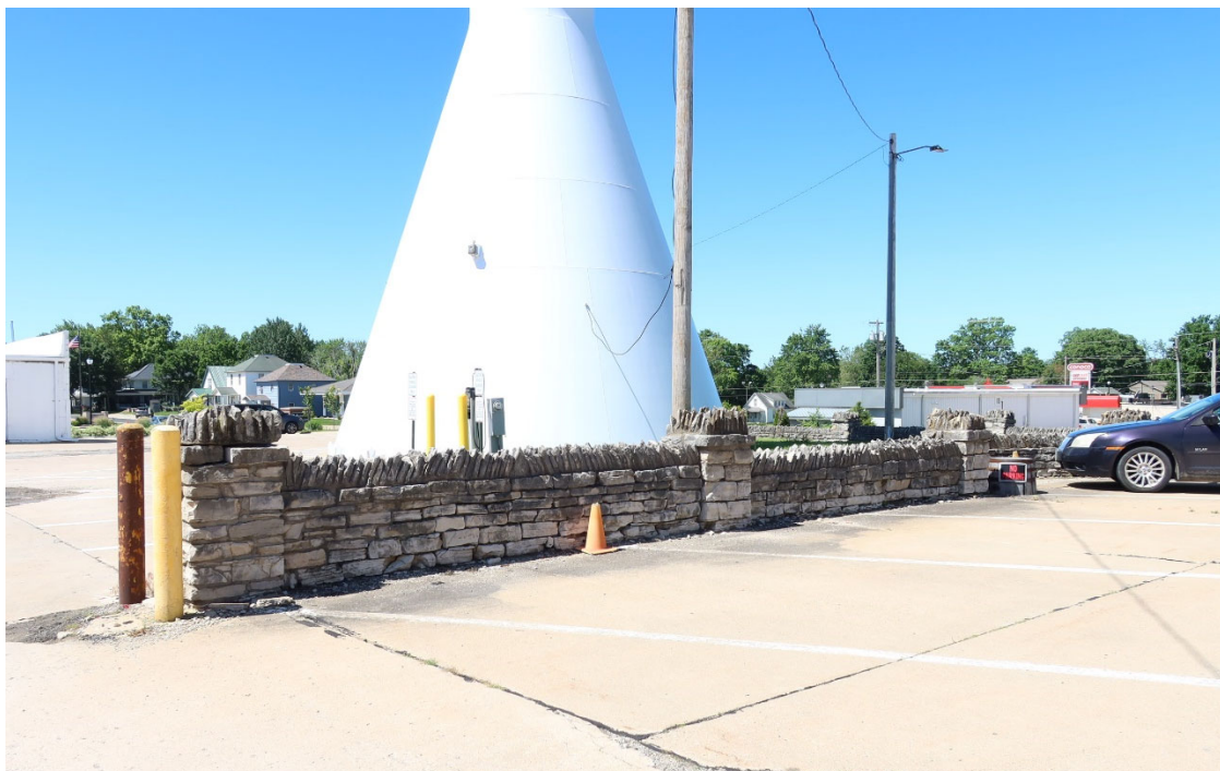
Photograph 44-00377-018. Stone wall, looking southwest (June 2024)
