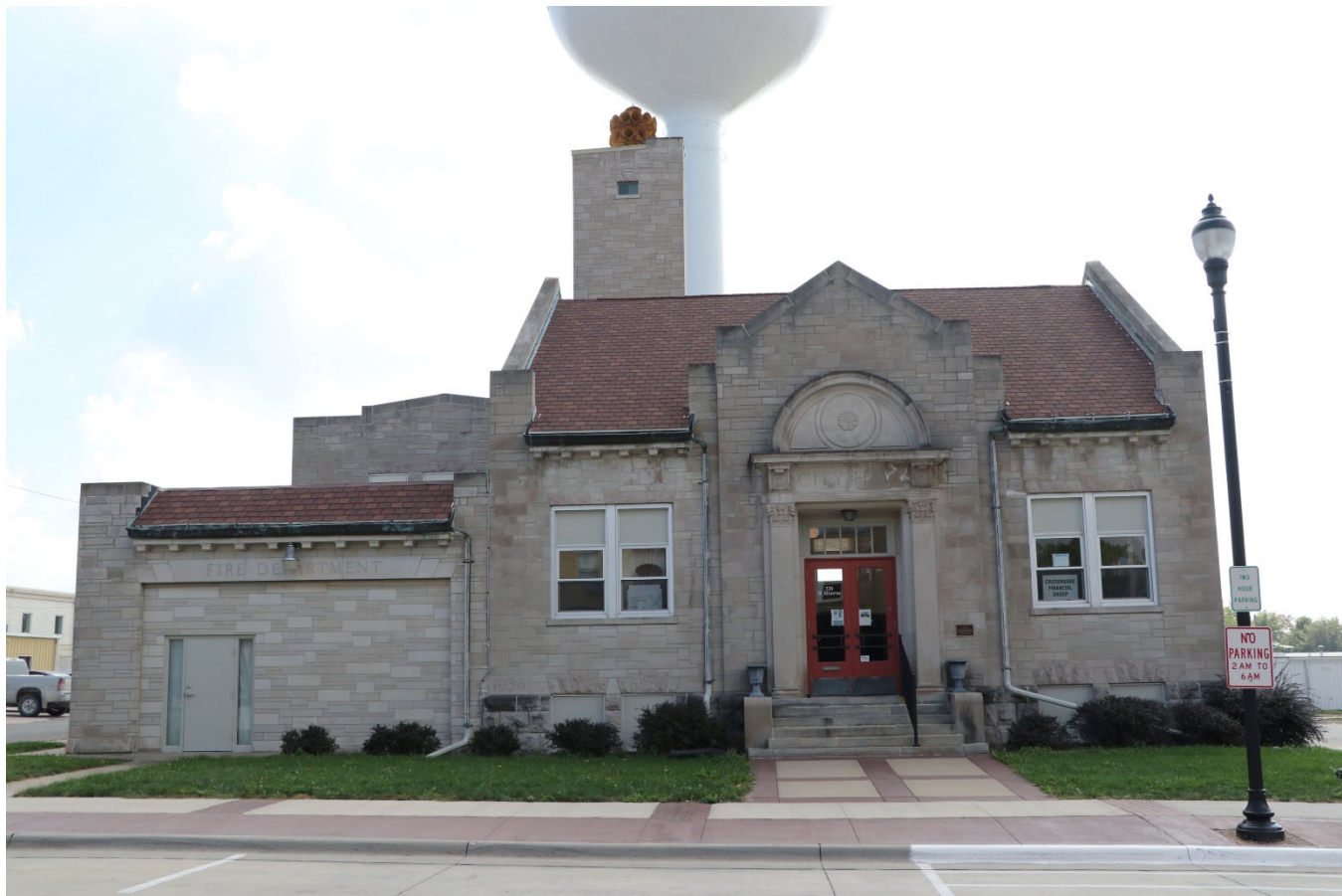
Photograph 44-00377-003. North elevation of City Hall, looking south (October 2023)
