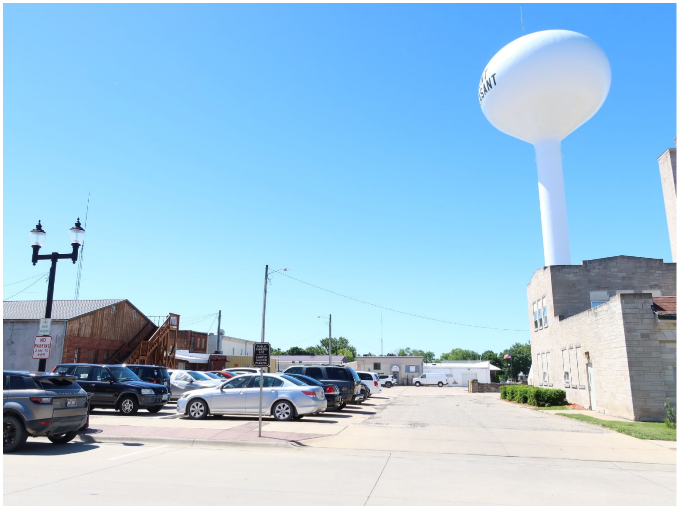
Photograph 44-00377-023. Parking lot to east of city hall, looking south (June 2024)
