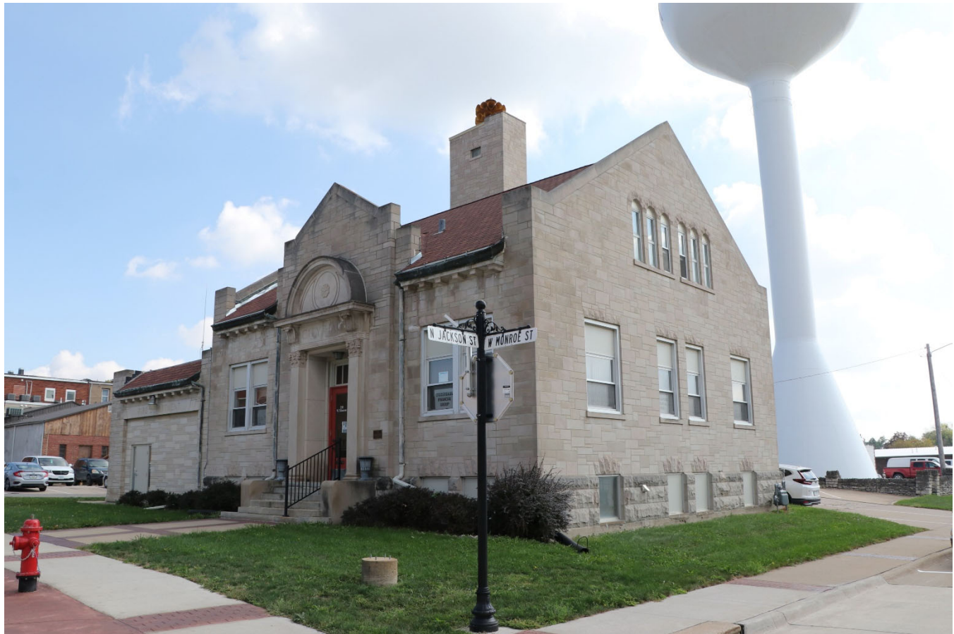
Photograph 44-00377-006. North and west elevations of City Hall, looking southeast (October 2023)
