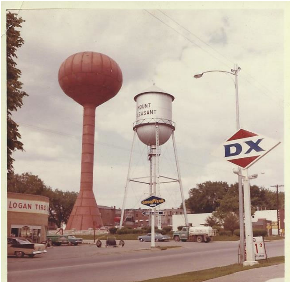
New and old water towers in May 1964 (HCHT Facebook album) prior to painting of new water tower
