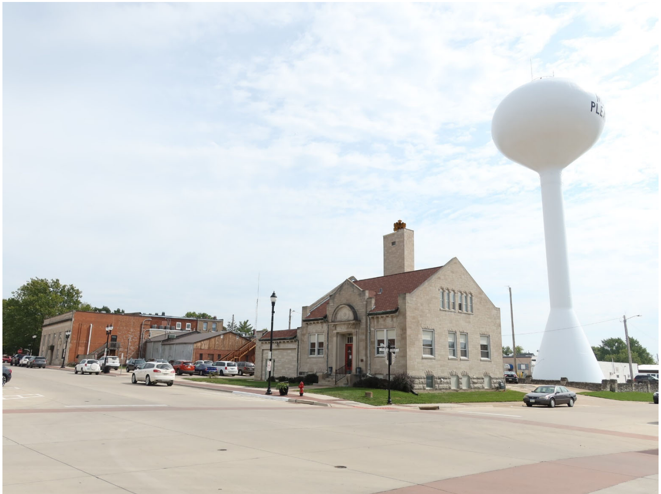
Photograph 44-00377-001. City hall, water tower, stone fence, and parking, looking southeast (June 2024)
