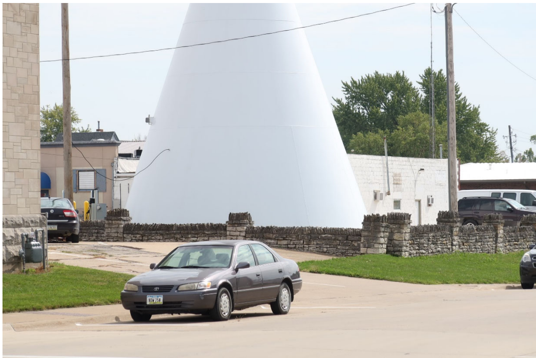
Photograph 44-00377-013. Stone wall, looking southeast (June 2024)
