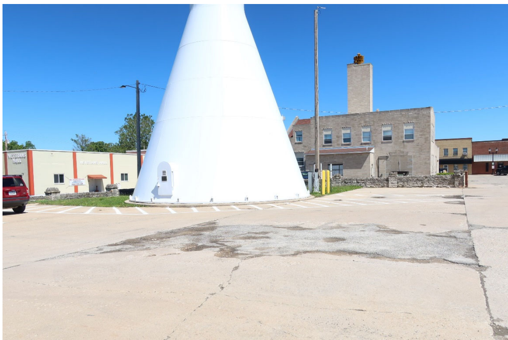
Photograph 44-00377-020. Stone wall to west and north of base of water tower, looking northwest (June 2024)
