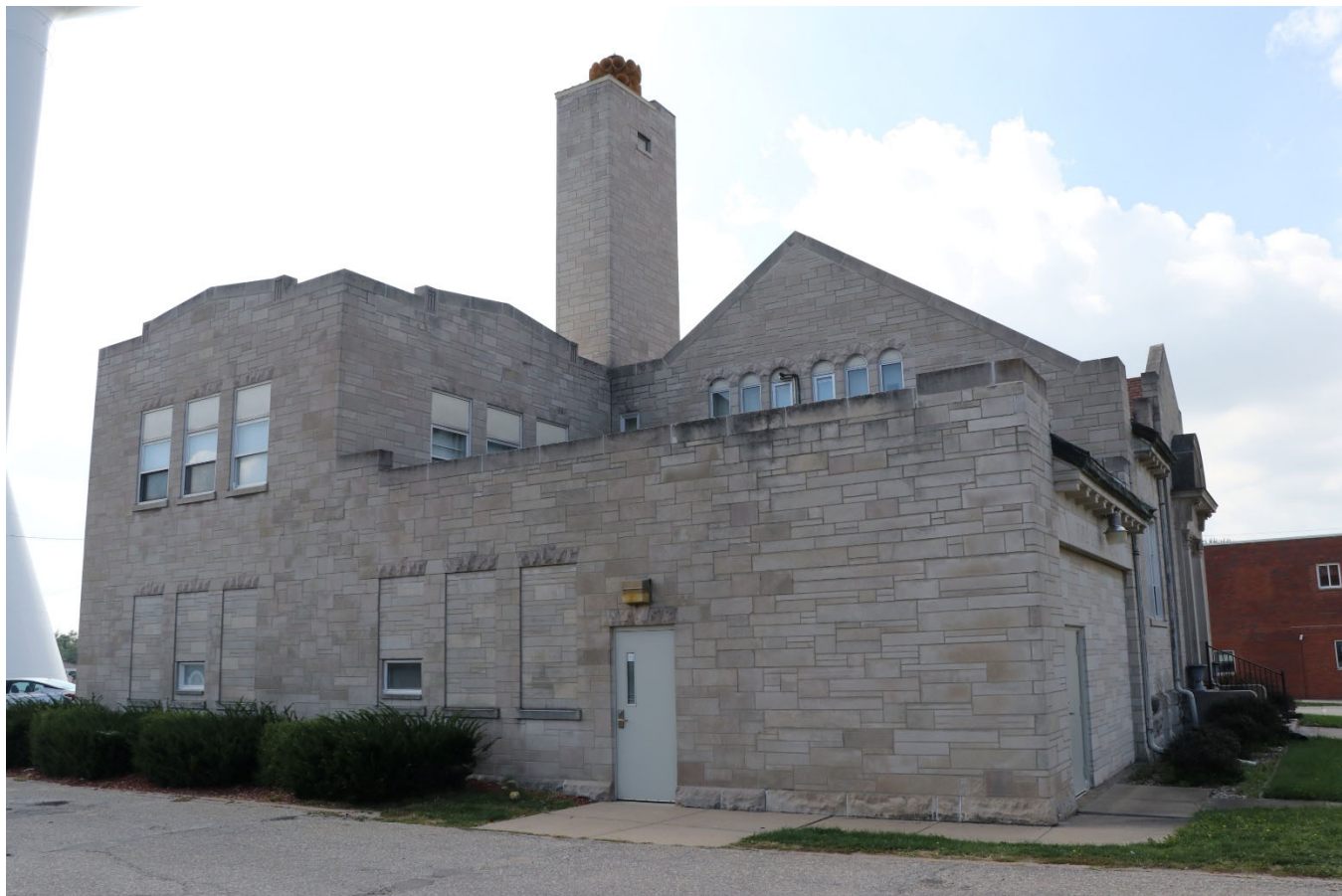
Photograph 44-00377-009. East elevation of City Hall, looking southwest (October 2023)
