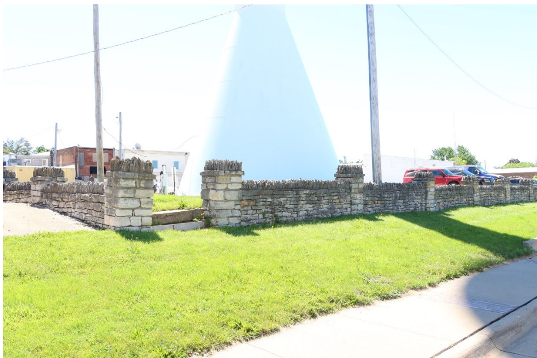
Photograph 44-00377-014. Stone wall, looking southeast (June 2024)
