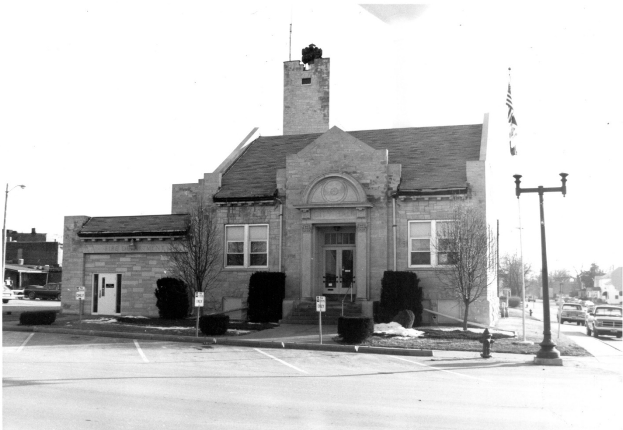
City Hall, 1990 survey photograph (Naumann 1991)
