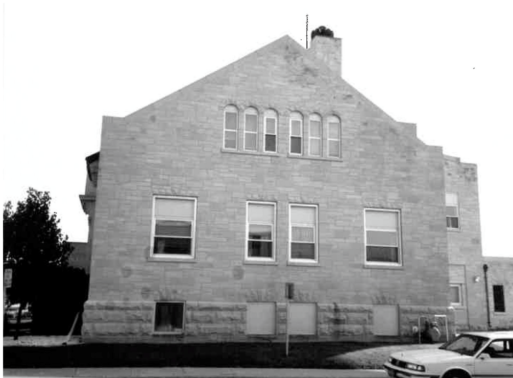
West side of City Hall, 1990 survey photograph (Naumann 1991)
