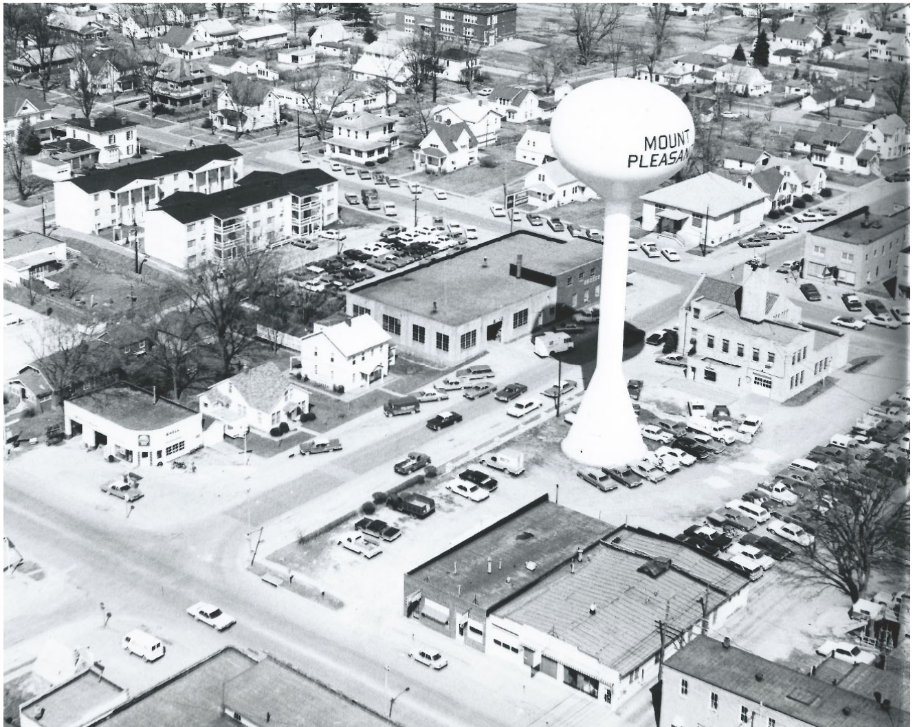
City hall with water tower to south and parking to east and south around 1970 (Magnuson, HCHT files)
