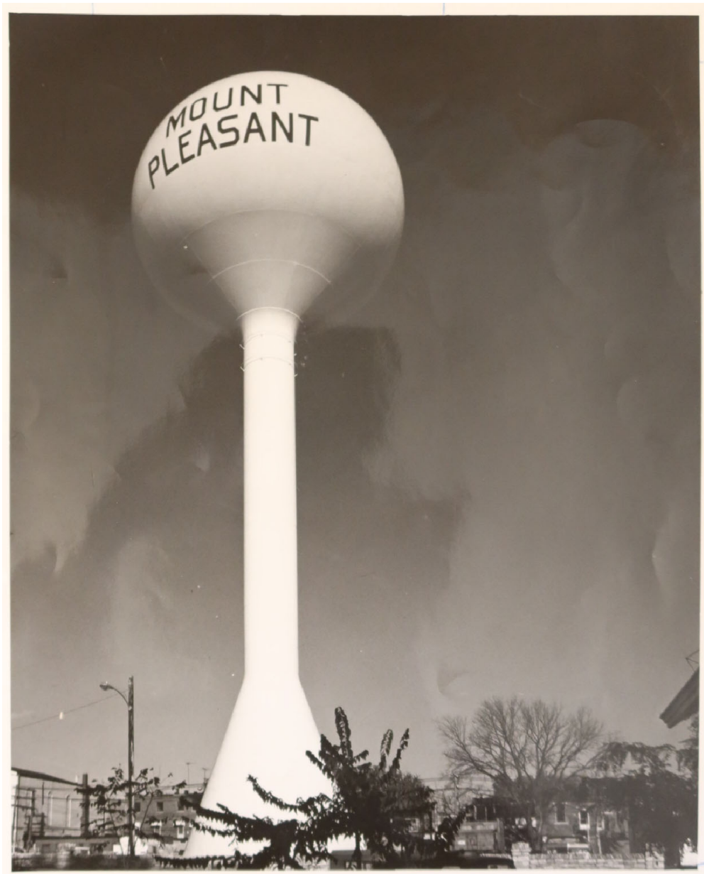
New water tower after completion (HCHS binder, Mt Pleasant Library)
