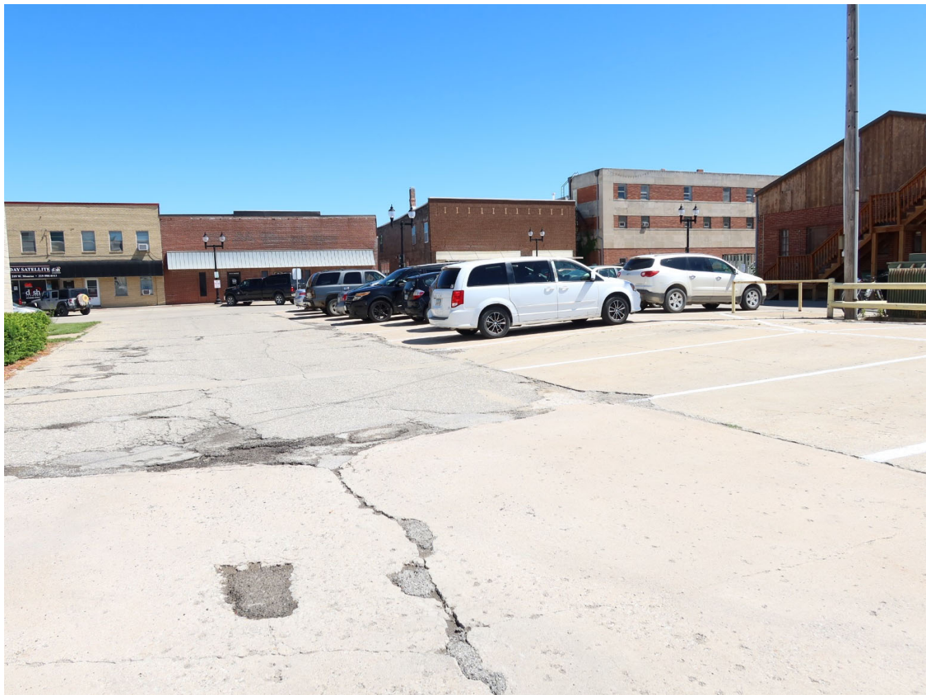
Photograph 44-00377-025. Parking lot to east of city hall, looking northeast (June 2024)
