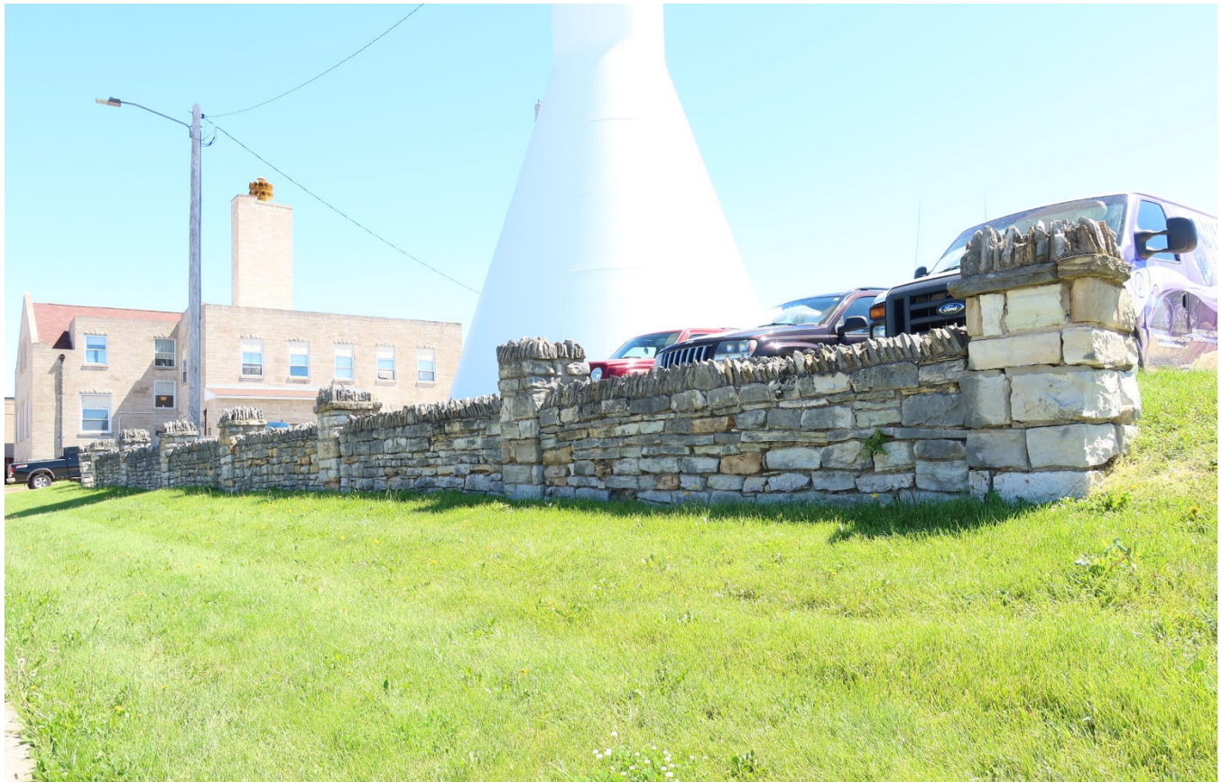
Photograph 44-00377-016. Stone wall, looking northeast (June 2024)
