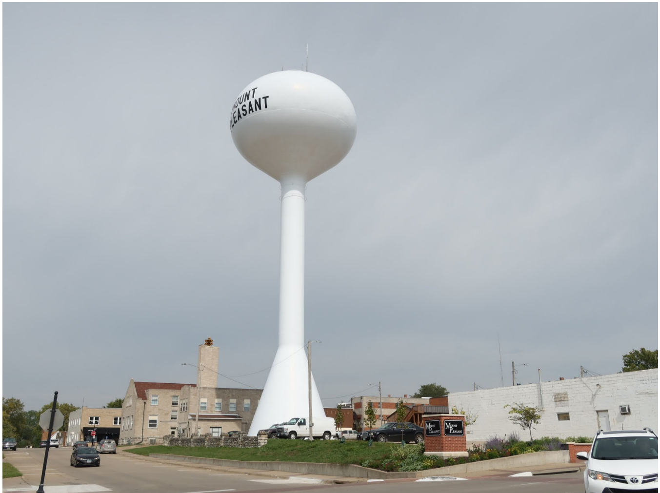
Photograph 44-00377-012. City hall, water tower, and stone wall, looking northeast (June 2024)
