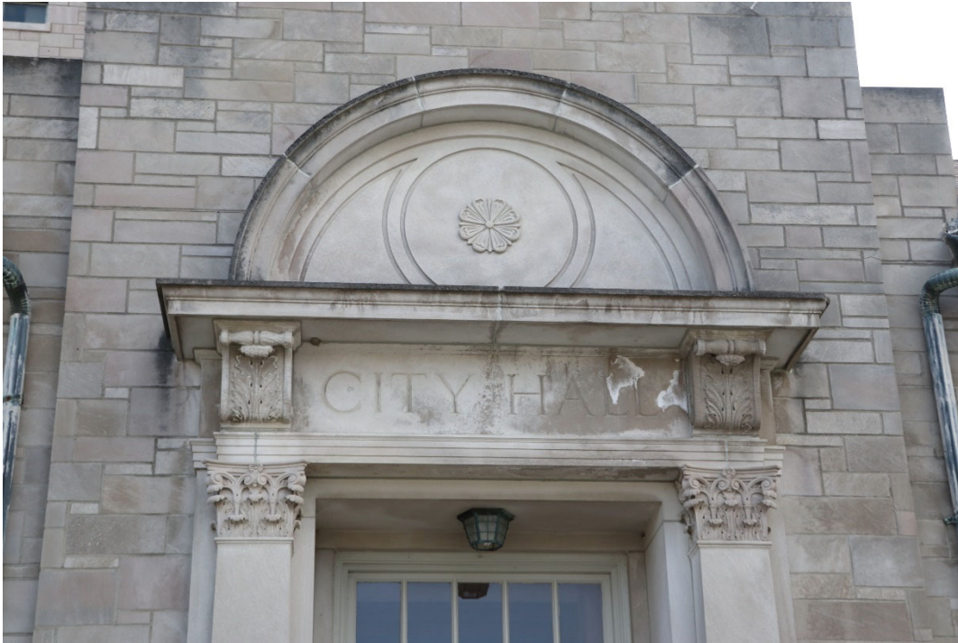
Photograph 44-00377-004. Detail above entry on north elevation of City Hall, looking south (October 2023)
