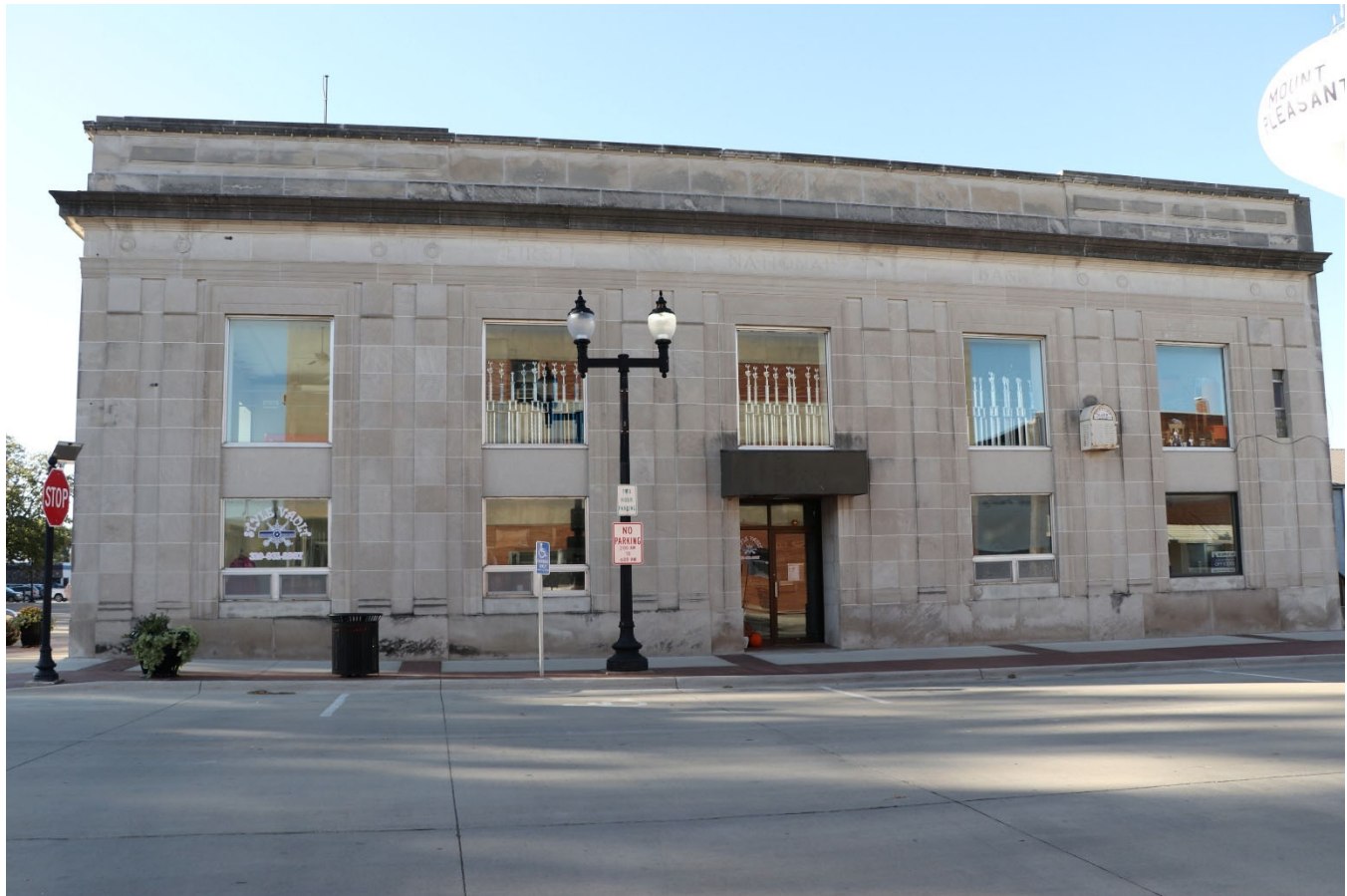
Photograph 44-00203-002. North elevation, looking south (October 2023)
