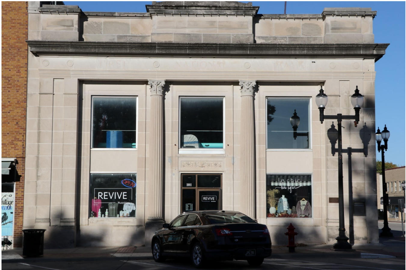
Photograph 44-00203-001. East elevation, looking west (October 2023)
