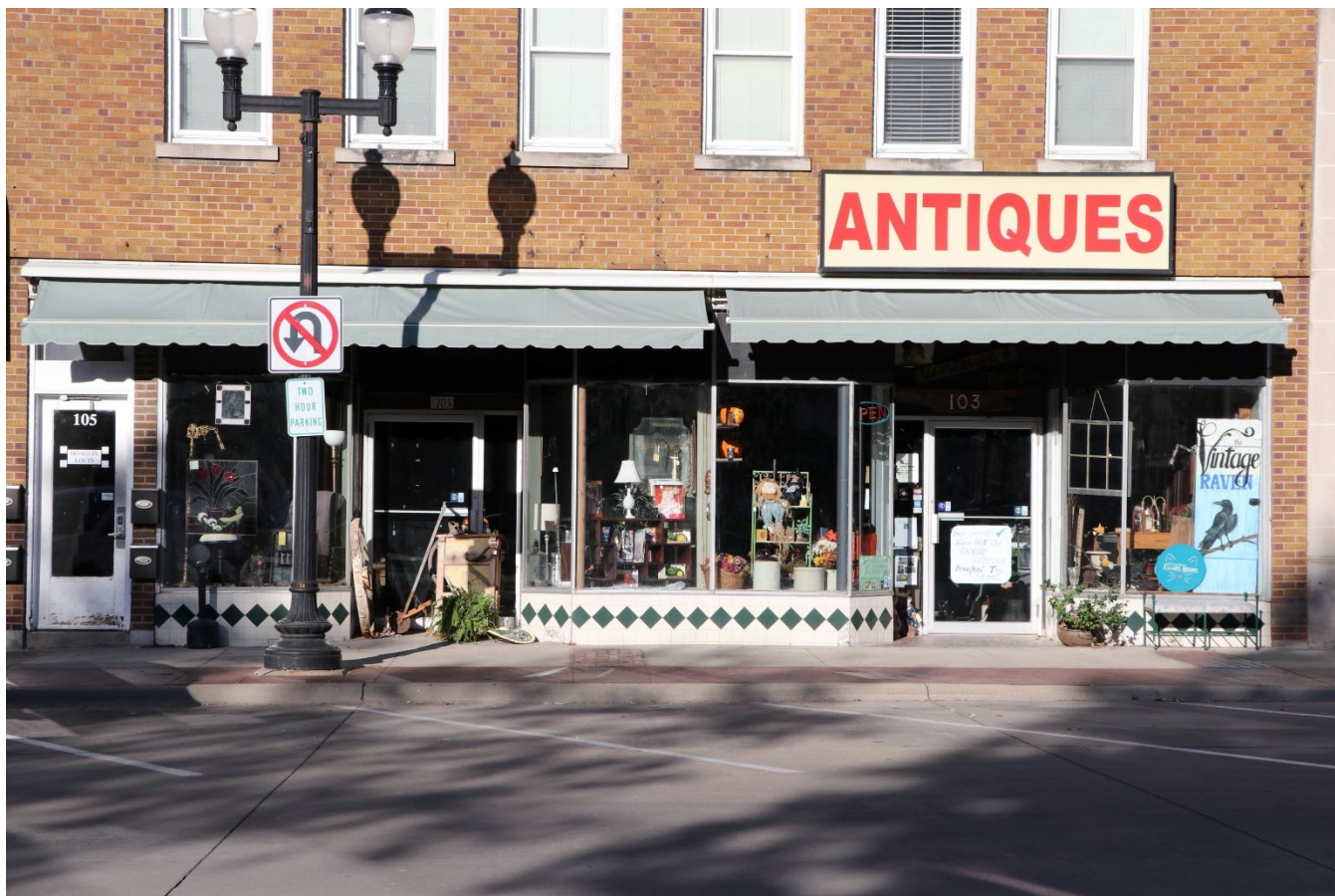
Photograph 44-00204-002. Storefront on east elevation, looking west (October 2023)
