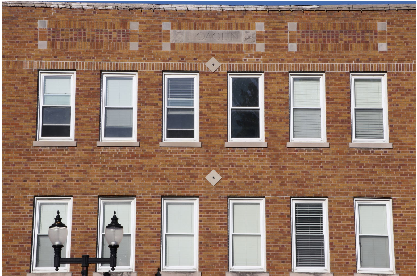
Photograph 44-00204-003. Upper stories on east elevation, looking west (October 2023)
