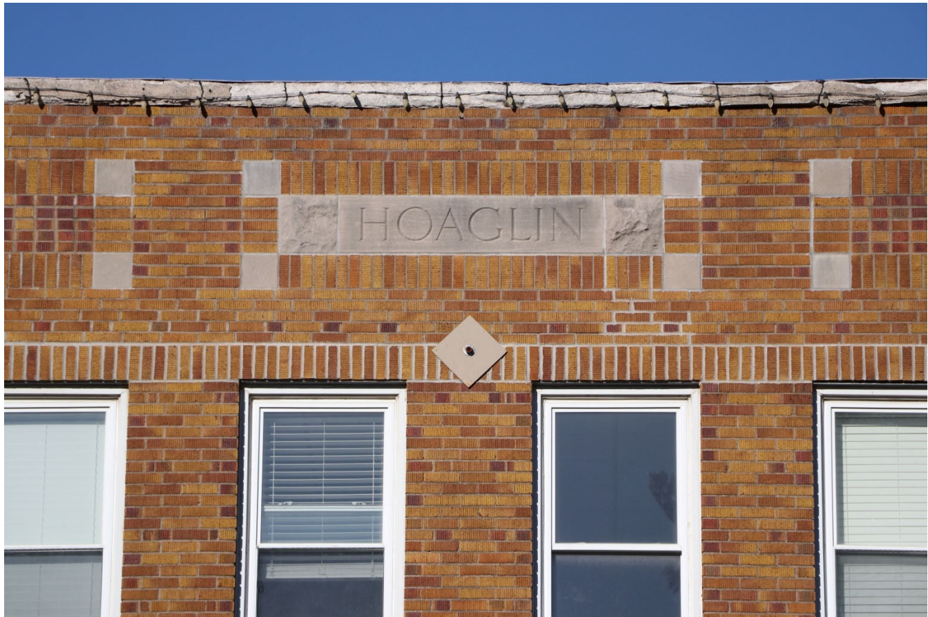
Photograph 44-00204-004. Parapet on east elevation, looking west (October 2023)
