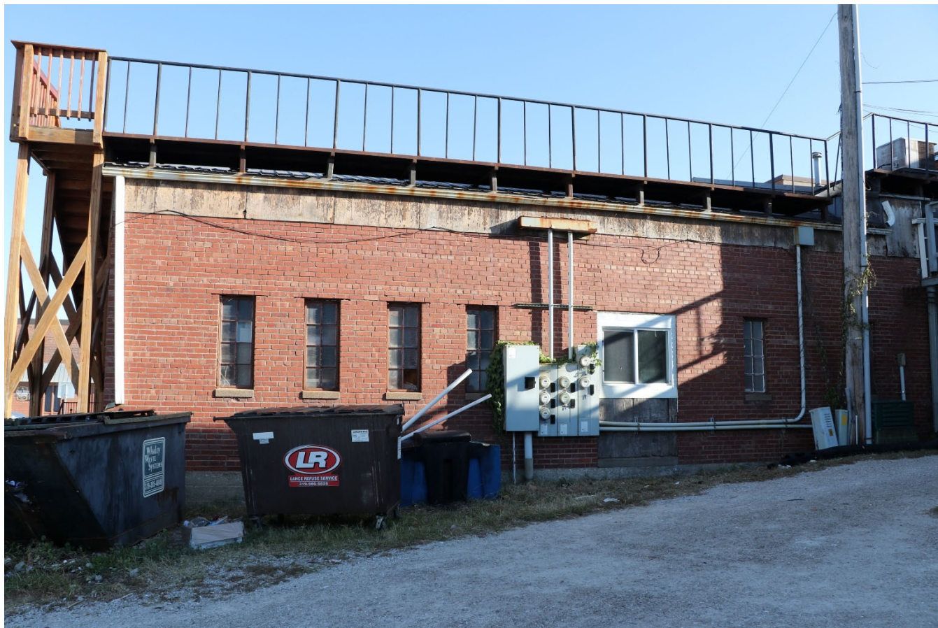
Photograph 44-00204-006. South elevation of rear addition, looking north (October 2023)
