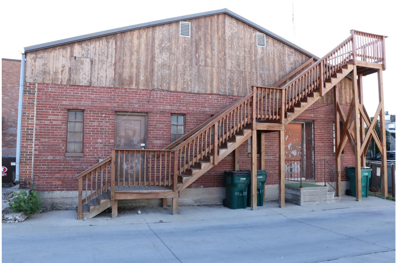
Photograph 44-00204-005. West (Rear) elevation of rear addition, looking east (October 2023)
