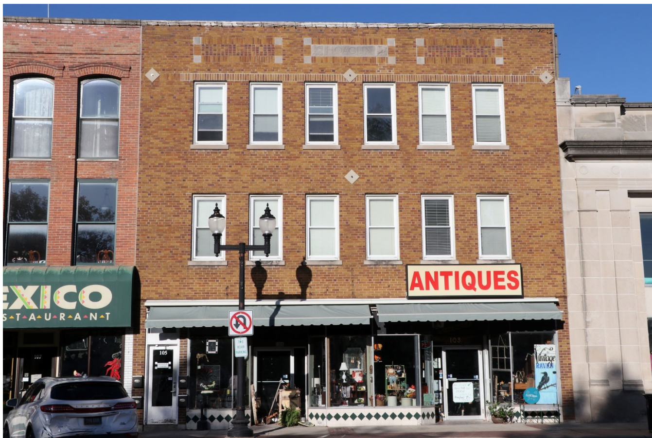
Photograph 44-00204-001. East elevation, looking west (October 2023)
