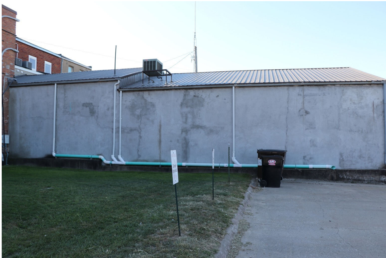
Photograph 44-00204-007. North elevation of rear addition, looking south (October 2023)
