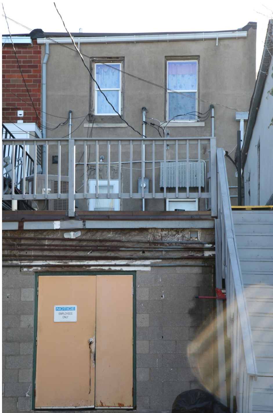
Photograph 44-00205-004. West elevation, looking east (October 2023)
