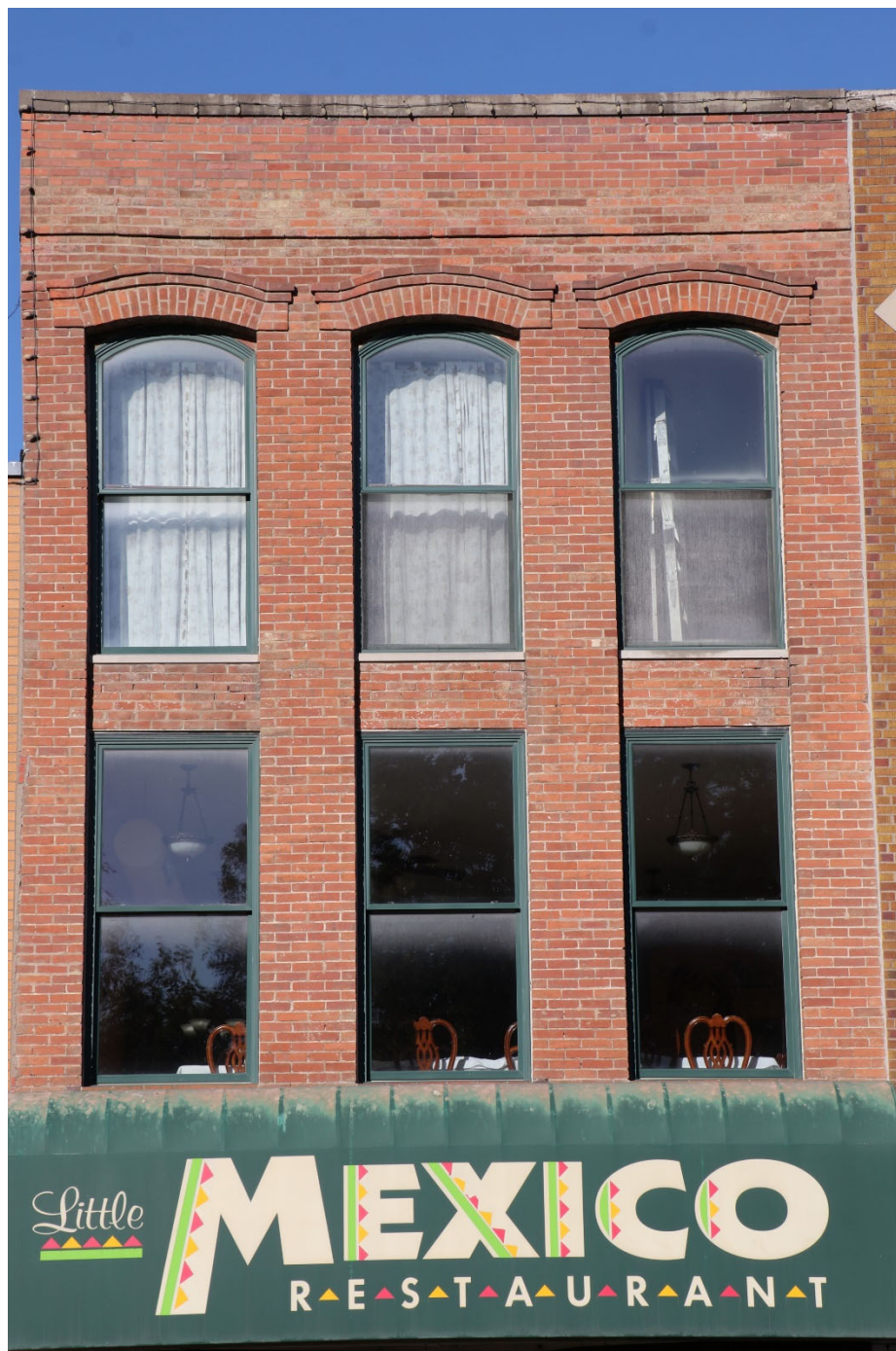
Photograph 44-00205-003. Upper stories on east elevation, looking west (October 2023)
