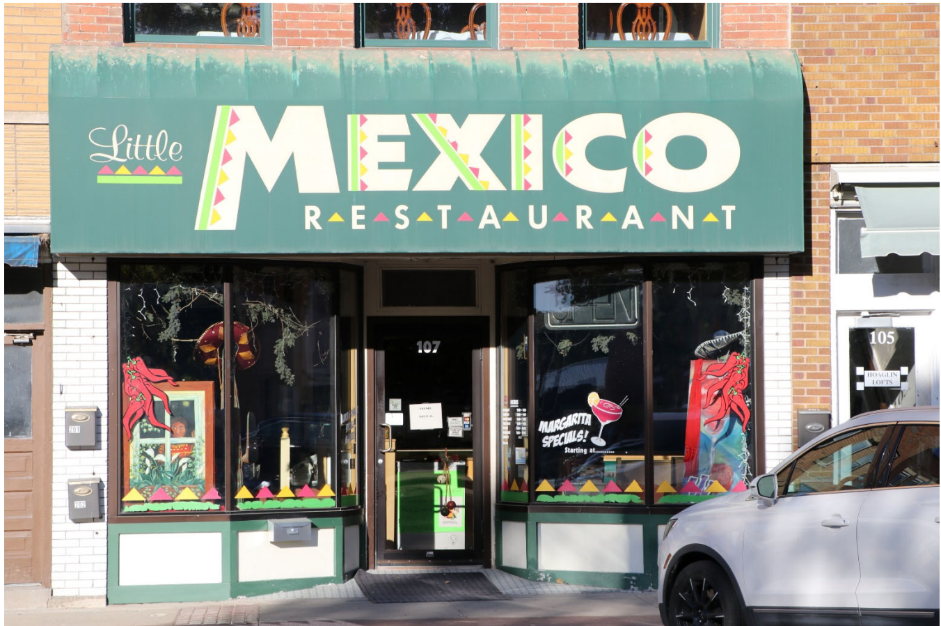
Photograph 44-00205-002. Storefront on east elevation, looking west (October 2023)
