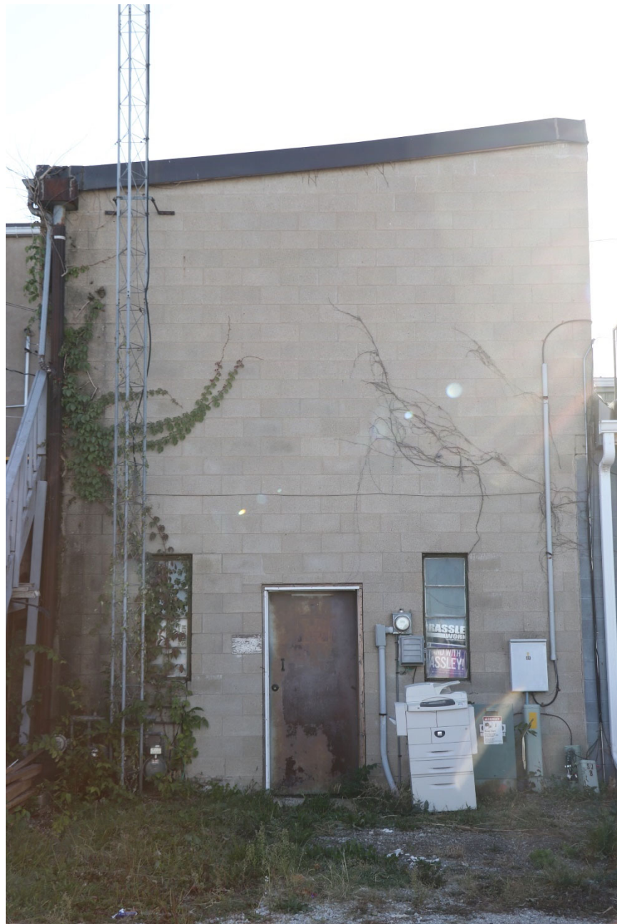
Photograph 44-00206-004. West elevation, looking east (October 2023)
