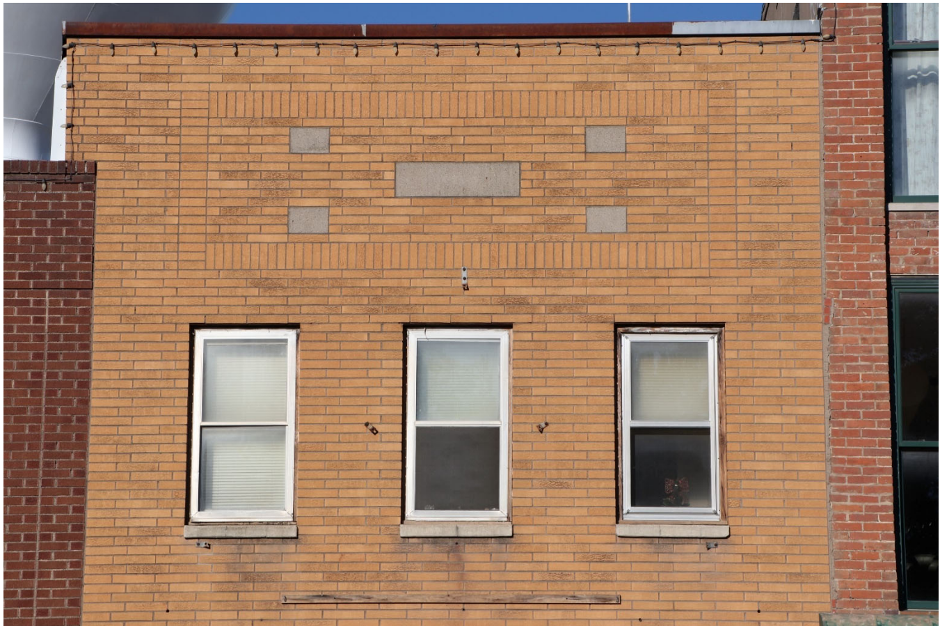
Photograph 44-00206-003. Upper portion of east elevation, looking west (October 2023)
