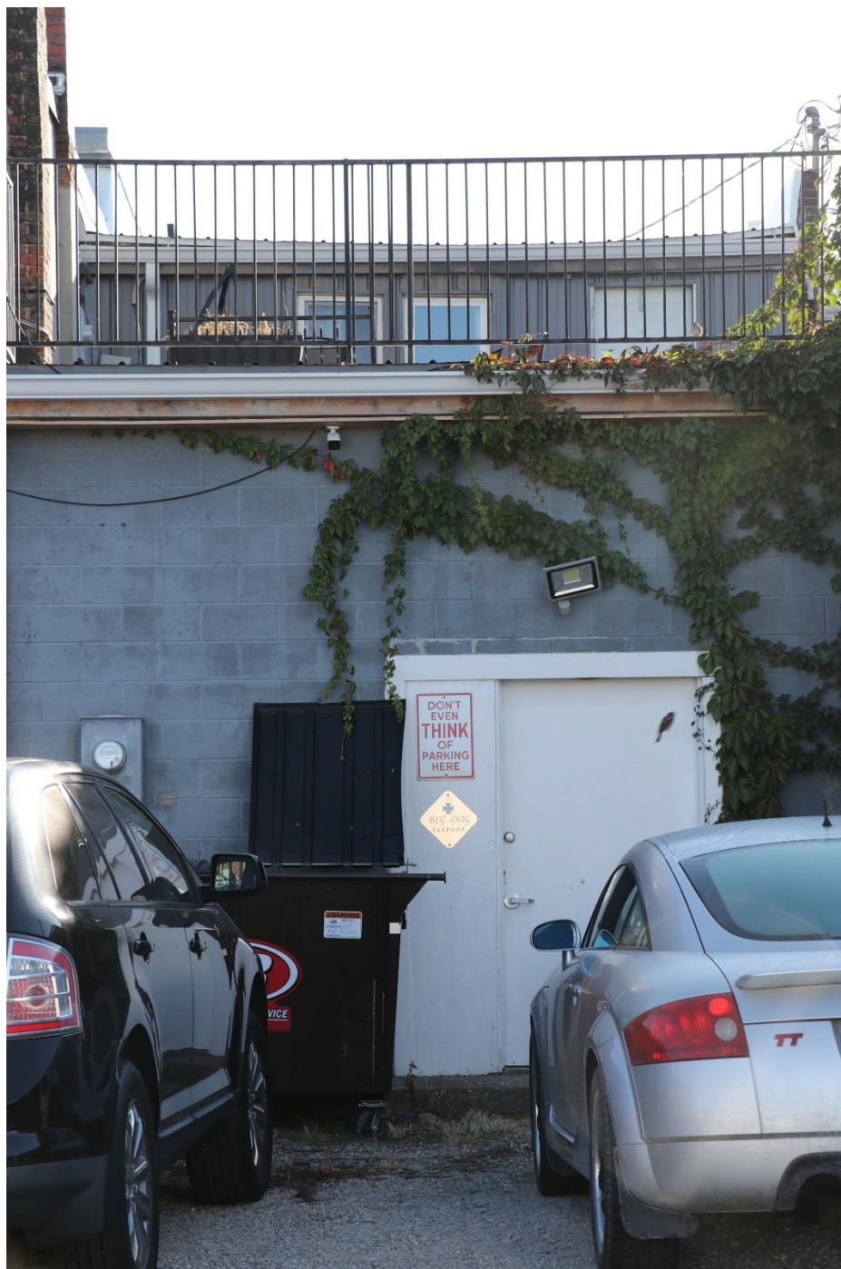
Photograph 44-00207-002. West elevation, looking east (October 2023)
