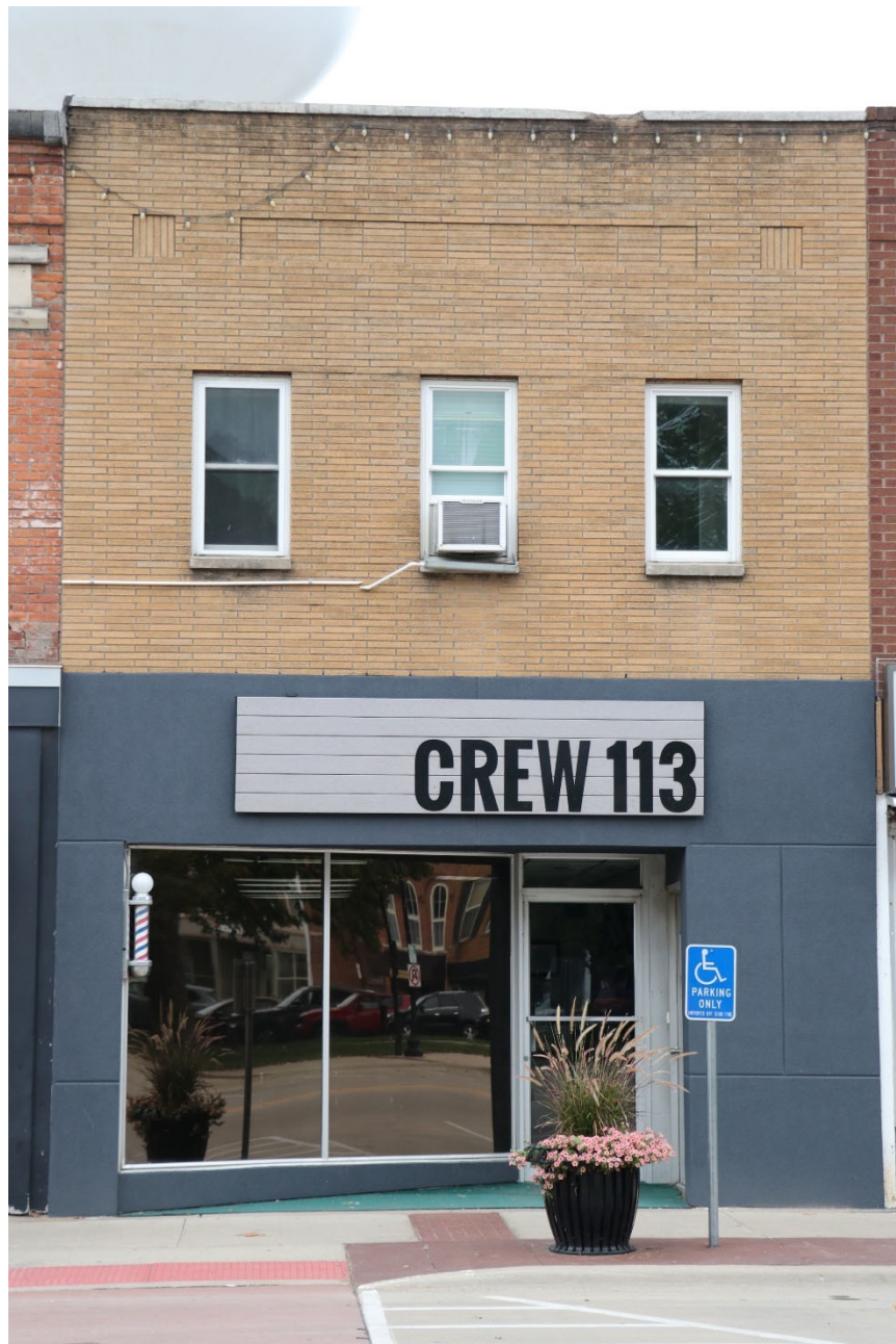
Photograph 44-00208-001. East elevation, looking west (October 2023)
