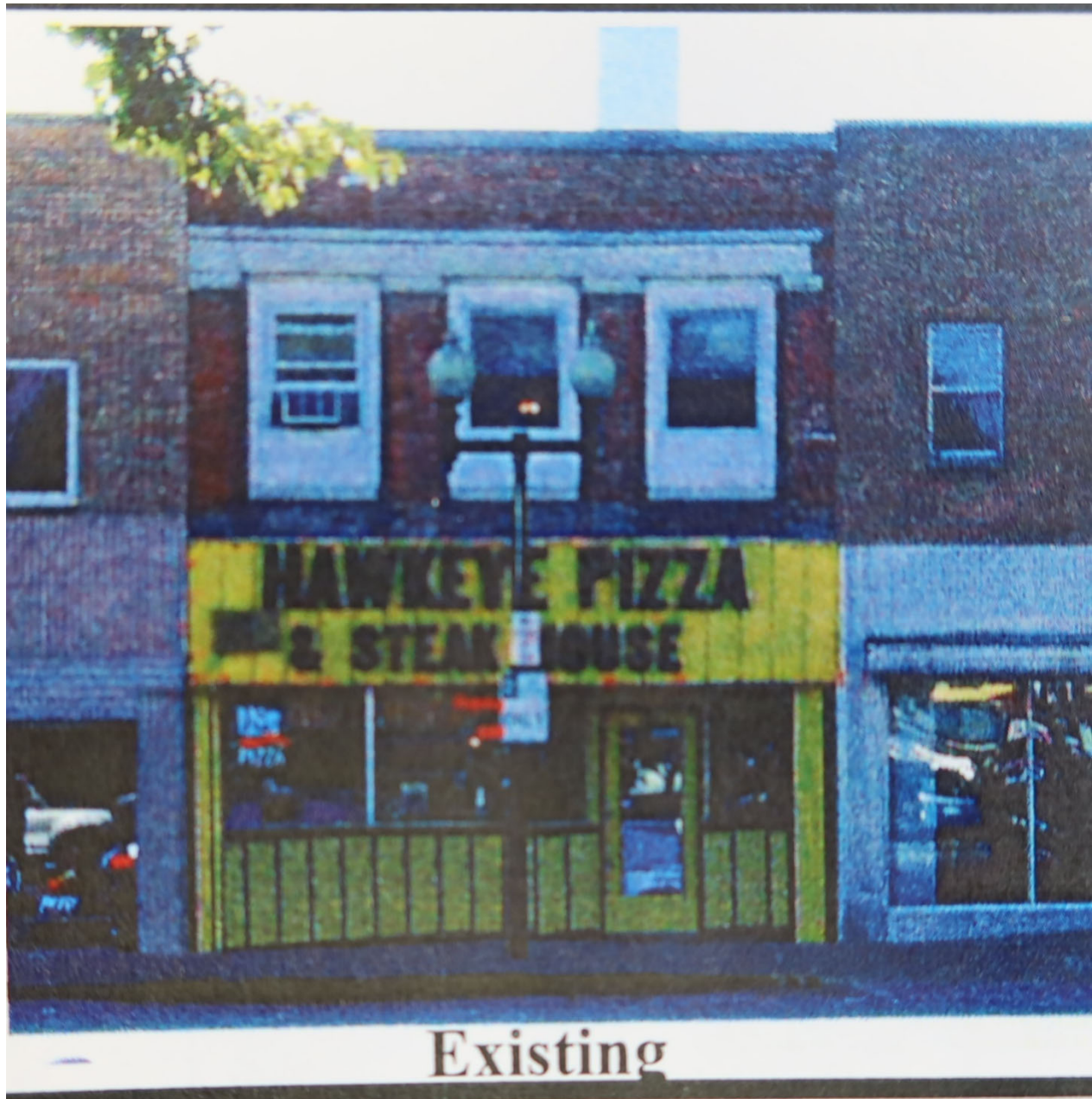
Building in May 2004 (City of Mt Pleasant building permits)
