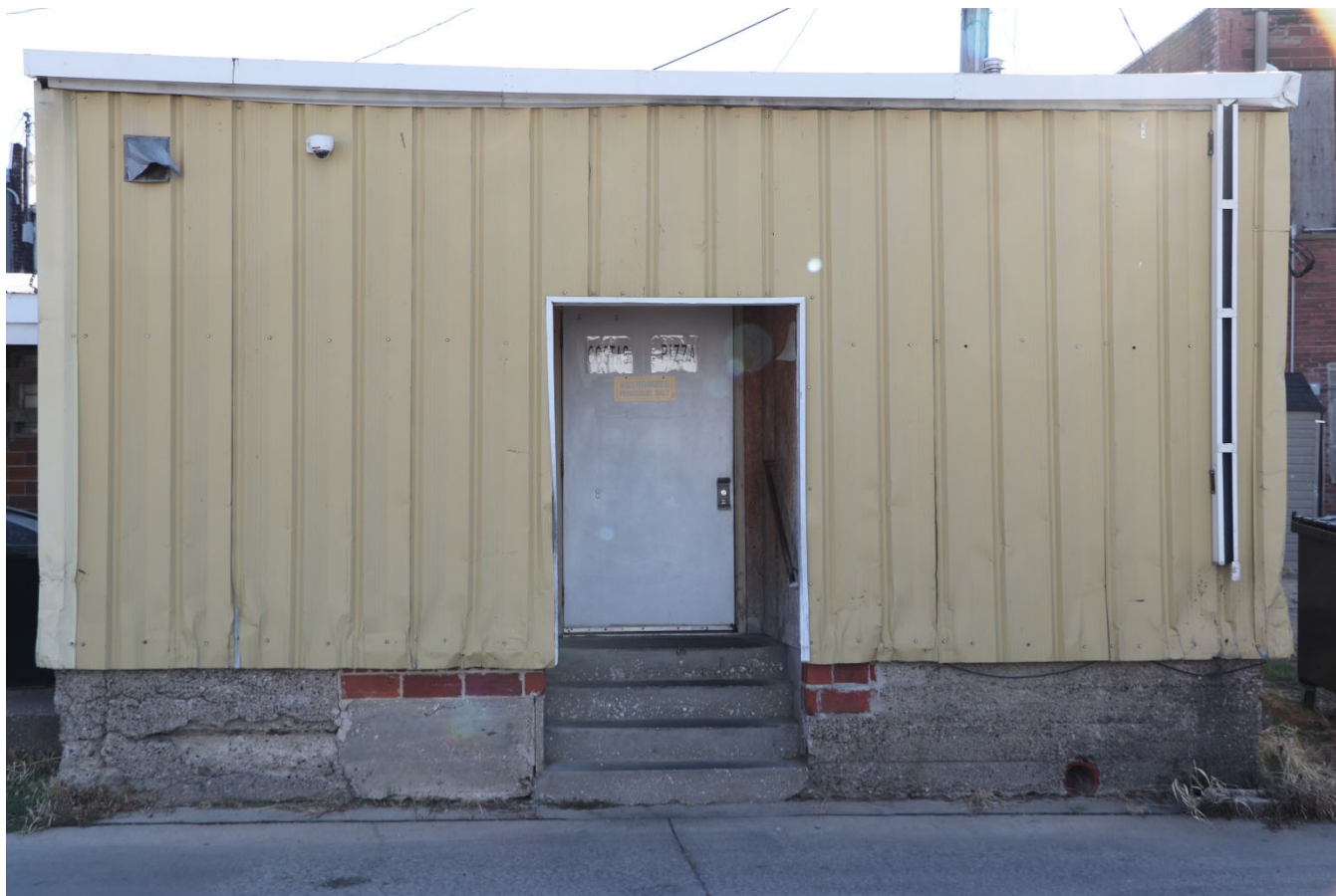
Photograph 44-00209-004. West (rear) elevation of rear addition, looking south (October 2023)
