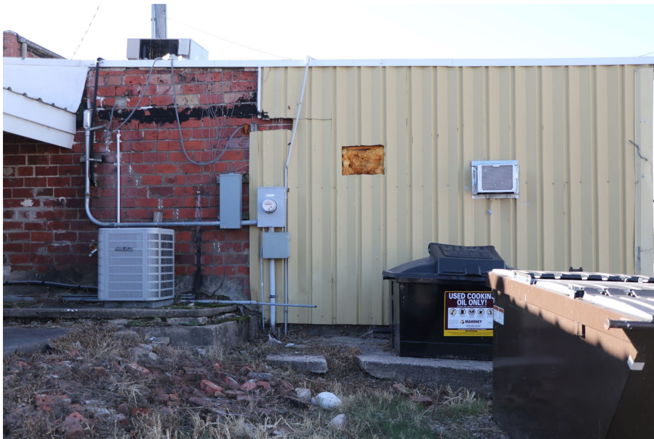
Photograph 44-00209-003. North elevation of rear addition, looking south (October 2023)
