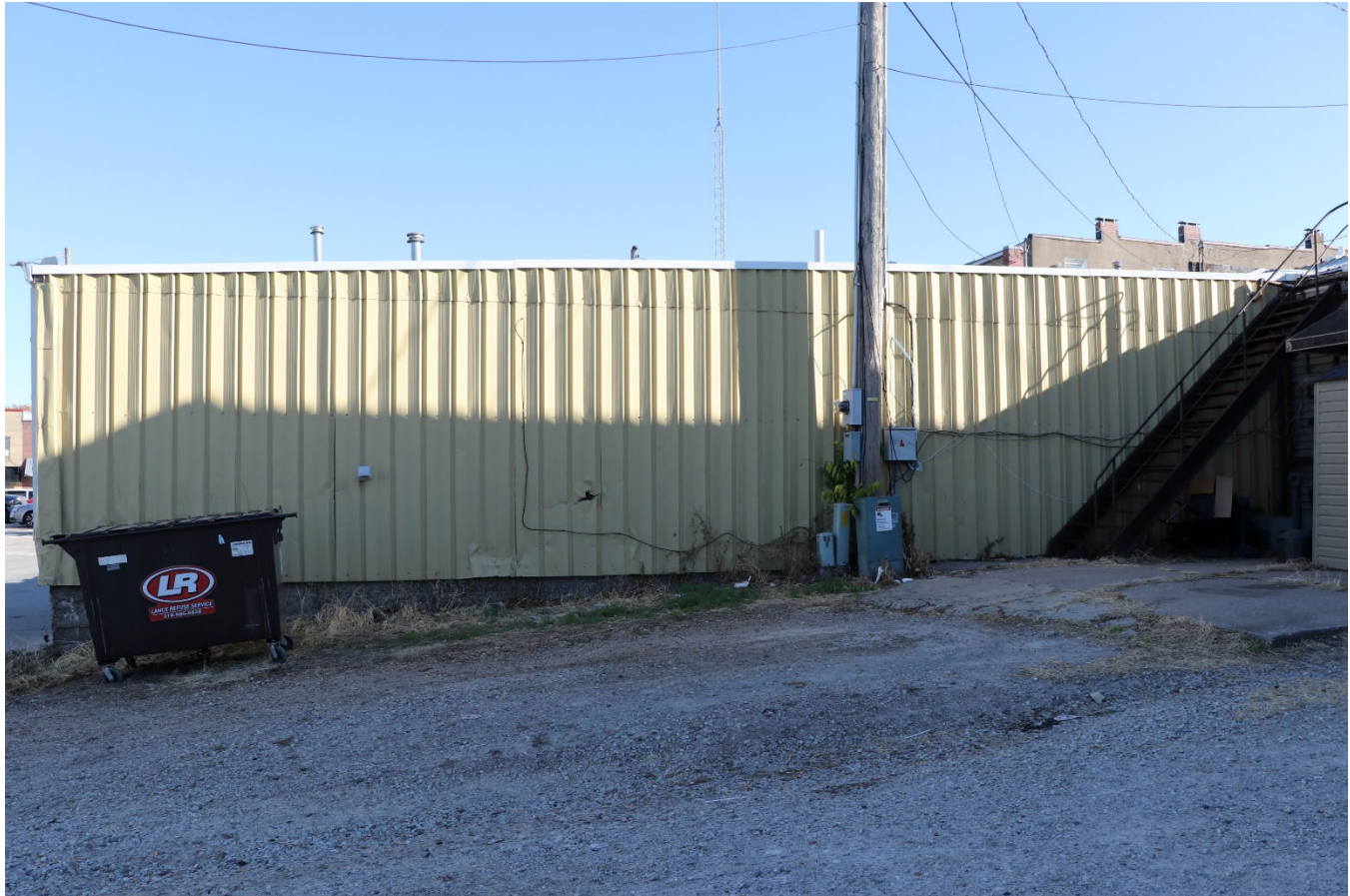
Photograph 44-00209-002. South elevation of rear addition, looking north (October 2023)
