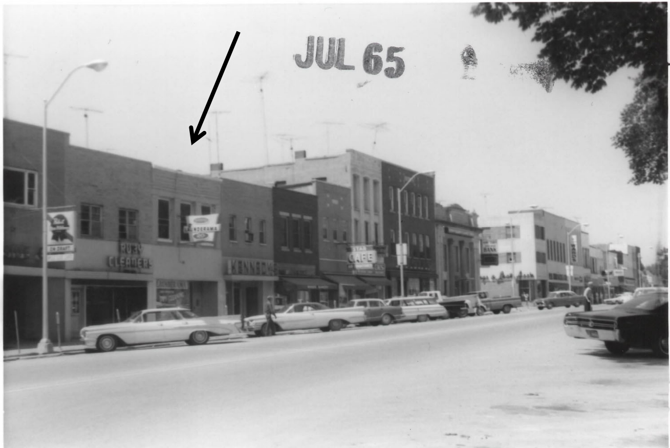
West side of square (100 block S. Jefferson St) in 1965 (HCHT collection)
