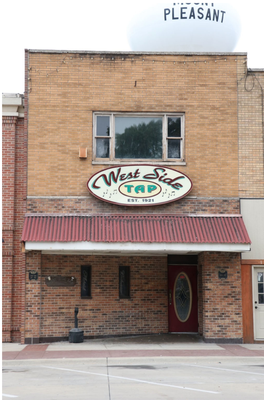
Photograph 44-00211-001. East elevation, looking west (October 2023)
