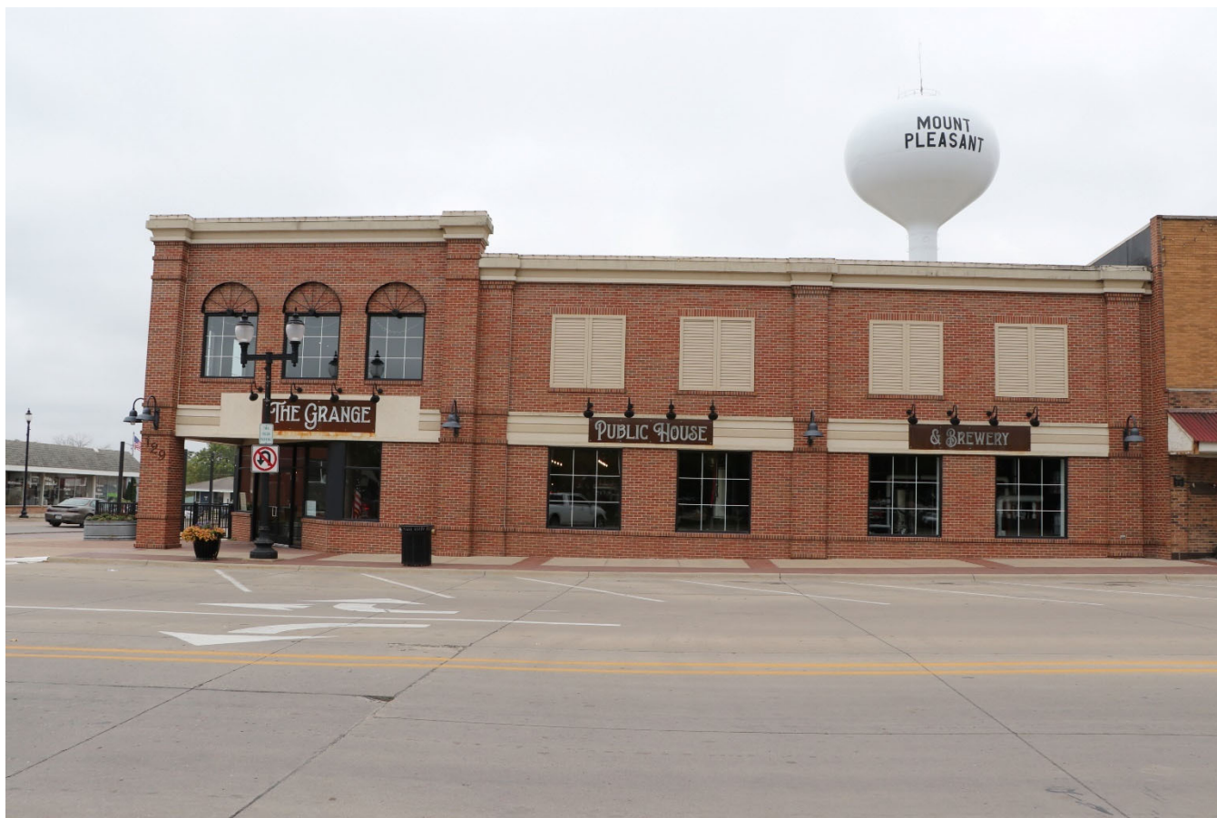
Photograph 44-02250-001. East elevation, looking west (October 2023)
