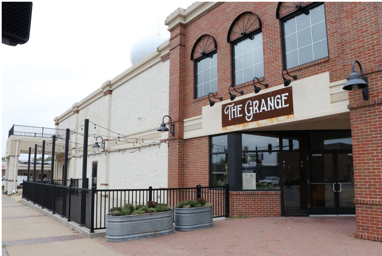
Photograph 44-02250-002. South elevation, looking northwest (October 2023)
