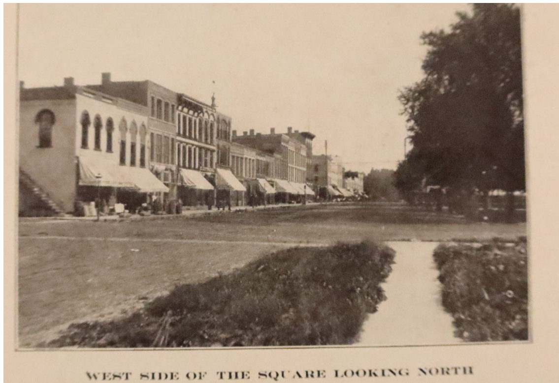
WEST SIDE OF THE SQUARE LOOKING NORTH Five buildings at south end of west side of square in 1909 ( Mt Pleasant Beautiful )
