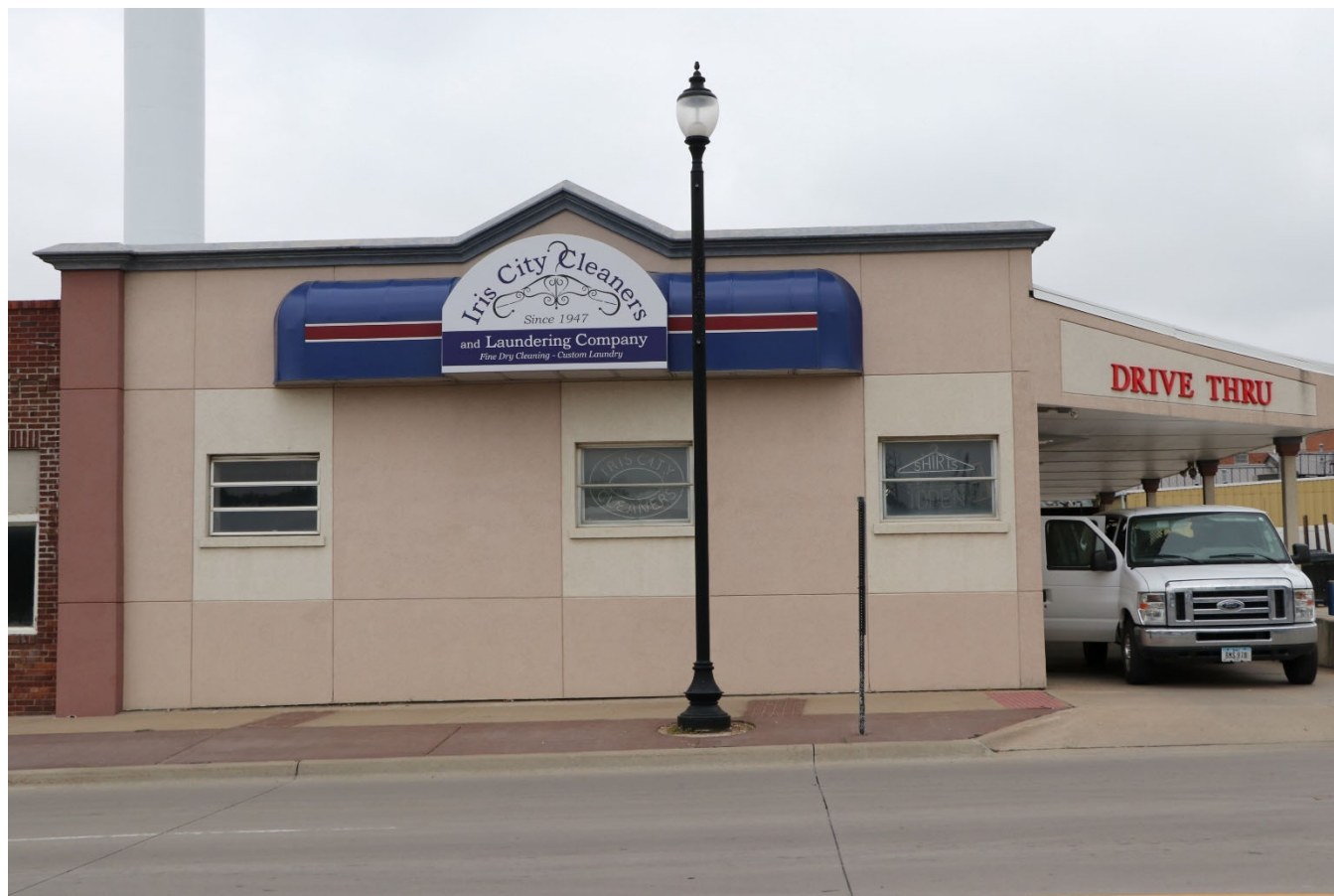
Photograph 44-00446-001. South elevation, looking north (October 2023)
