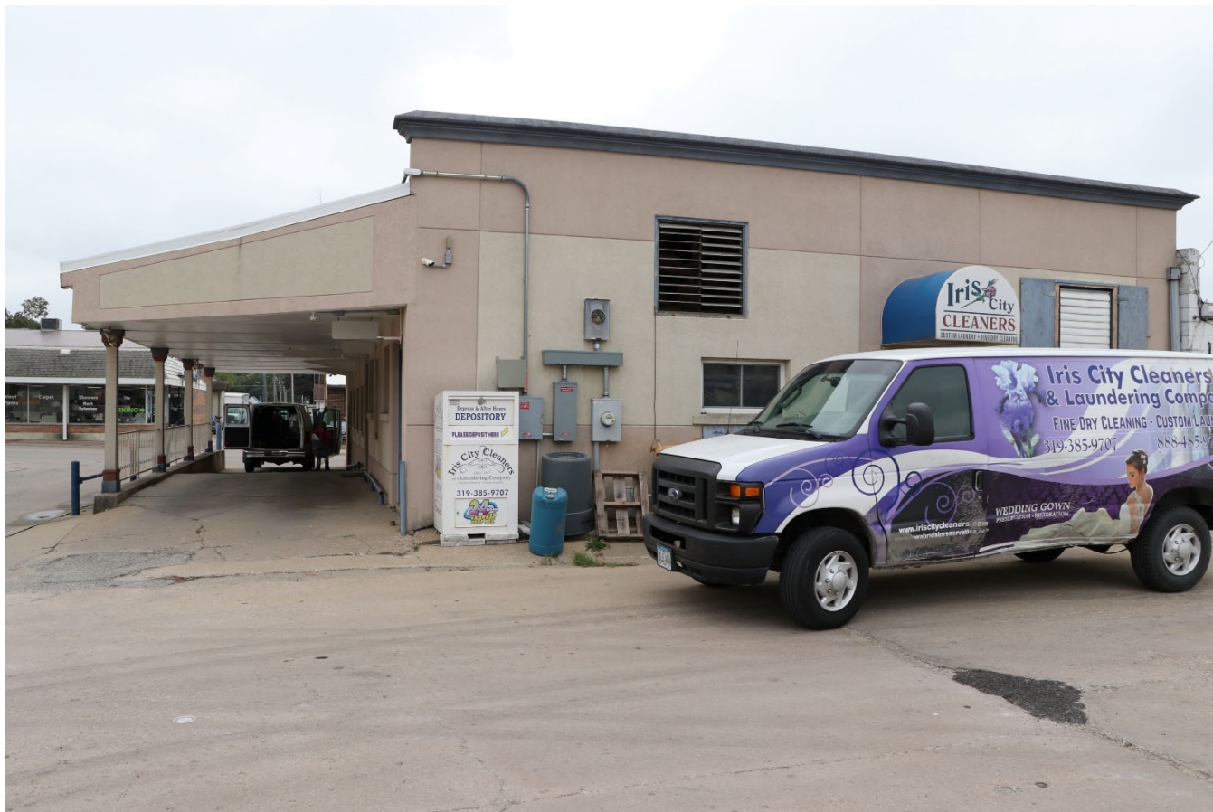
Photograph 44-00446-003. North elevation, looking south (October 2023)
